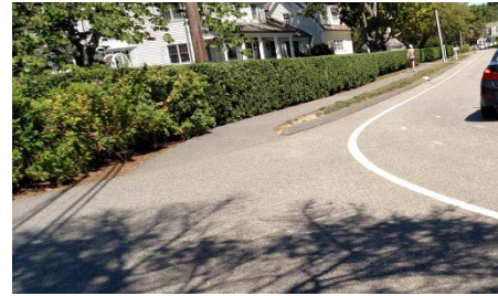
Figure 11. Sidewalk Ends at Owenoke Park
