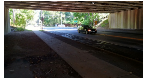
Figure 5. Under the I-95 Bridge
