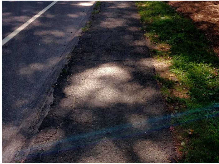
Figure 23. Repair Cracked Sidewalks
