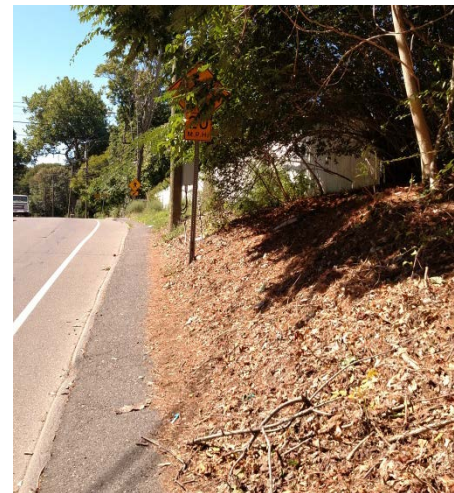
Figure 9. Narrowing Sidewalk Due to Leaf Debris
