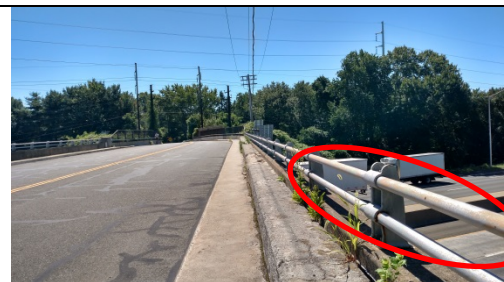
Figure 28. Add Fence to Railing
