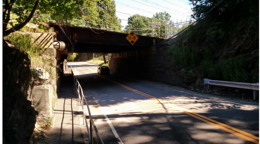
Figure 21. Add Lighting Under the Bridge
