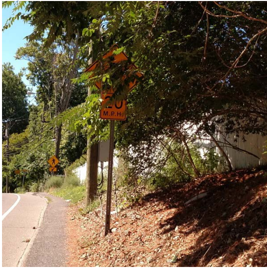
Figure 22. Trim Branches Blocking Sign
