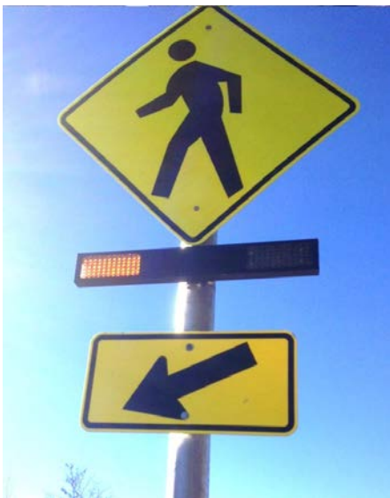
Figure 26. Rectangular Rapid Flashing Beacon
