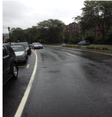
Figure 5. Sharp Curve with Limited Sight Distance on Union Street
