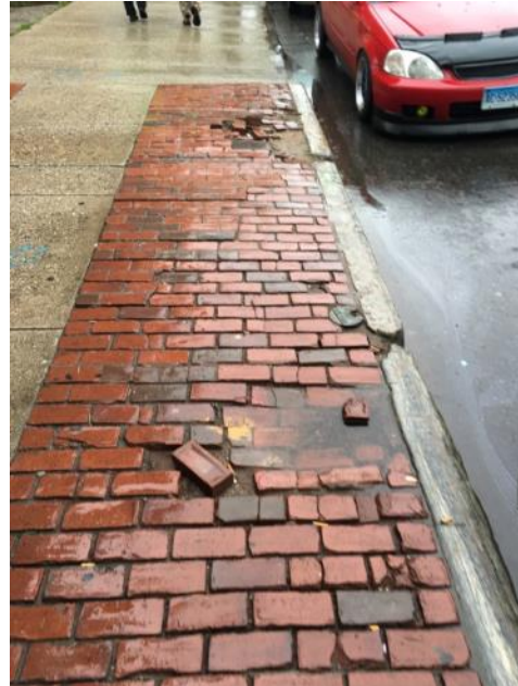
Figure 17. Repair Damaged Sidewalks
