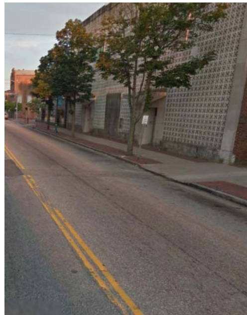
Figure 19. Add Shoulder Lane Markings
