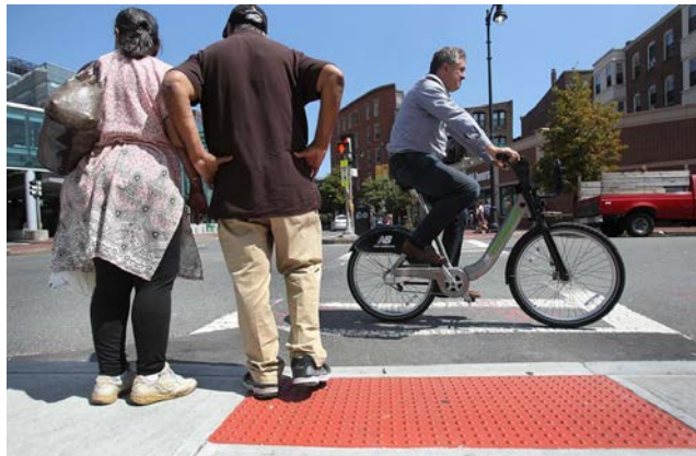
Figure 29. Ramp and Tactile Warning Strip
