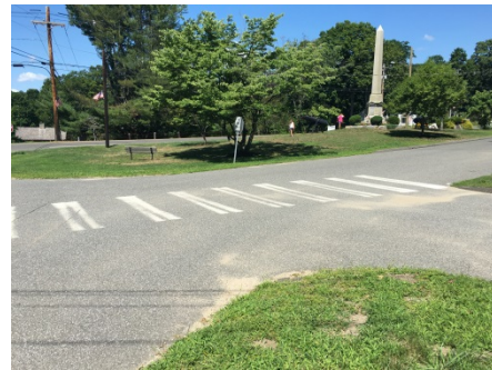
Figure 12. Crosswalk at the Main Street and Park Road Intersection
