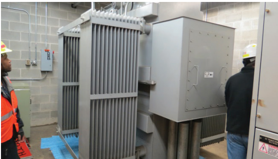
FIGURE 3-26: LIQUID FILLED TRANSFORMER
