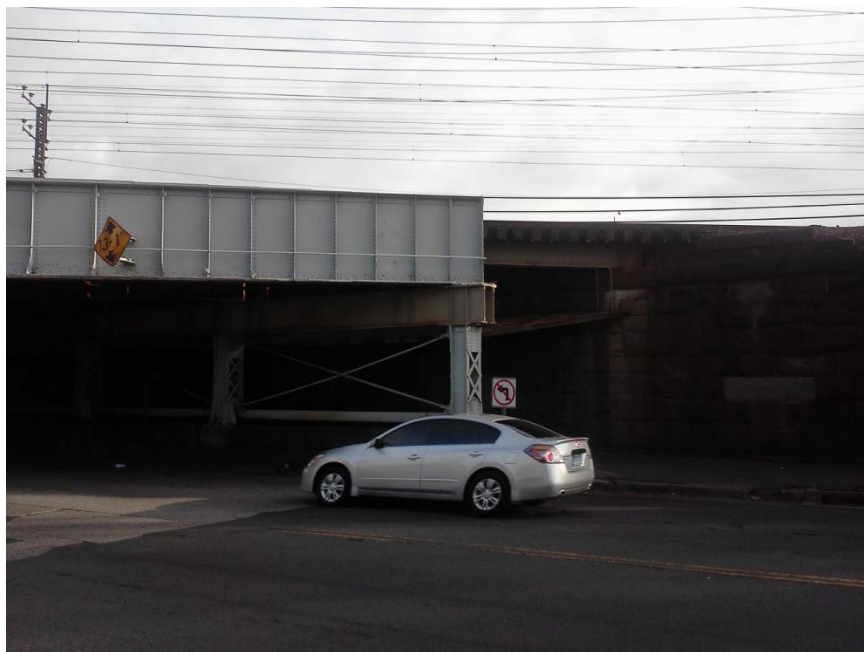
South Elevation of the East Main Street Bridge
