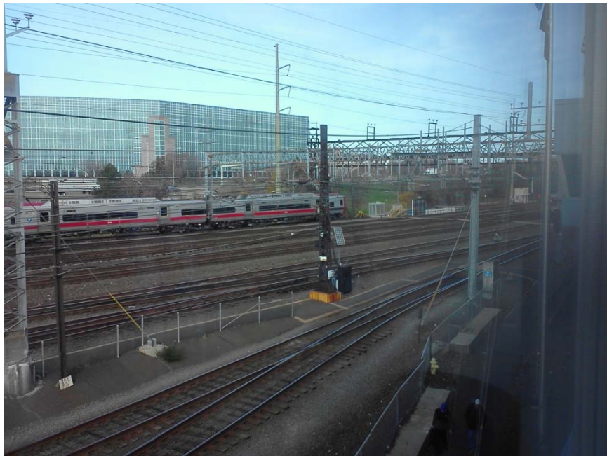
View of entrance to rail yard
