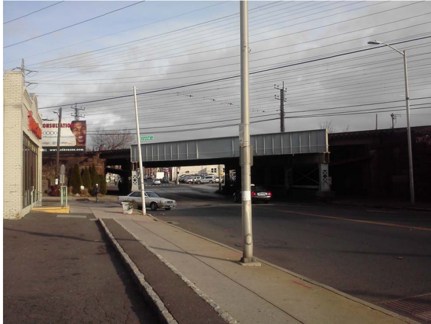
North Elevation of the East Main Street Bridge
