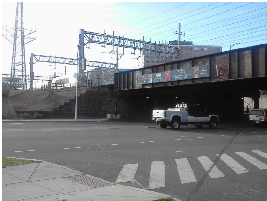
South Elevations of the Atlantic Street Bridge
