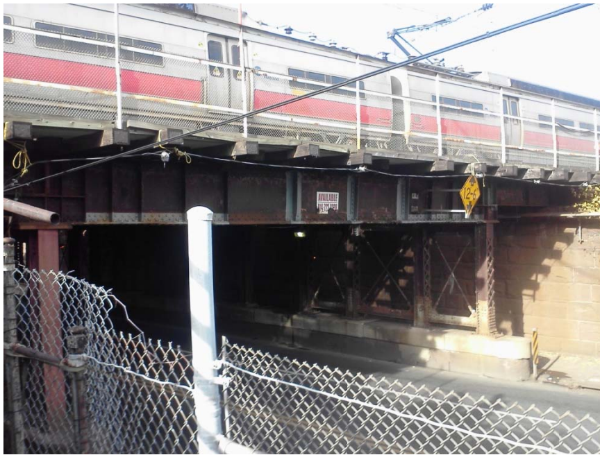
South Elevation of the Elm Street Bridge
