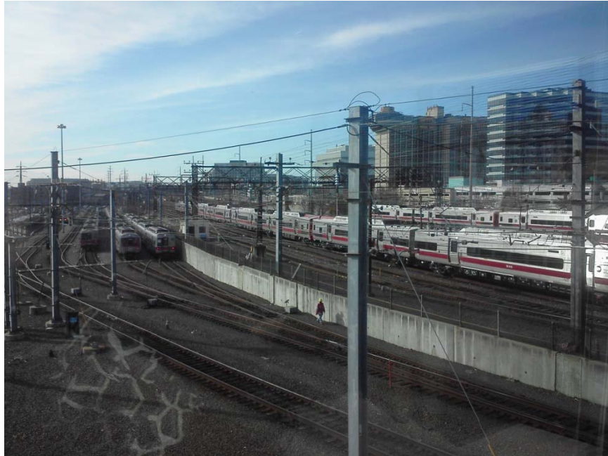
View of rail yard looking west
