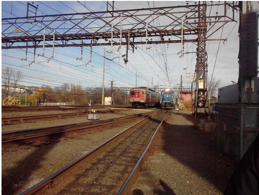
Top View of the Elm Street Bridge looking east
