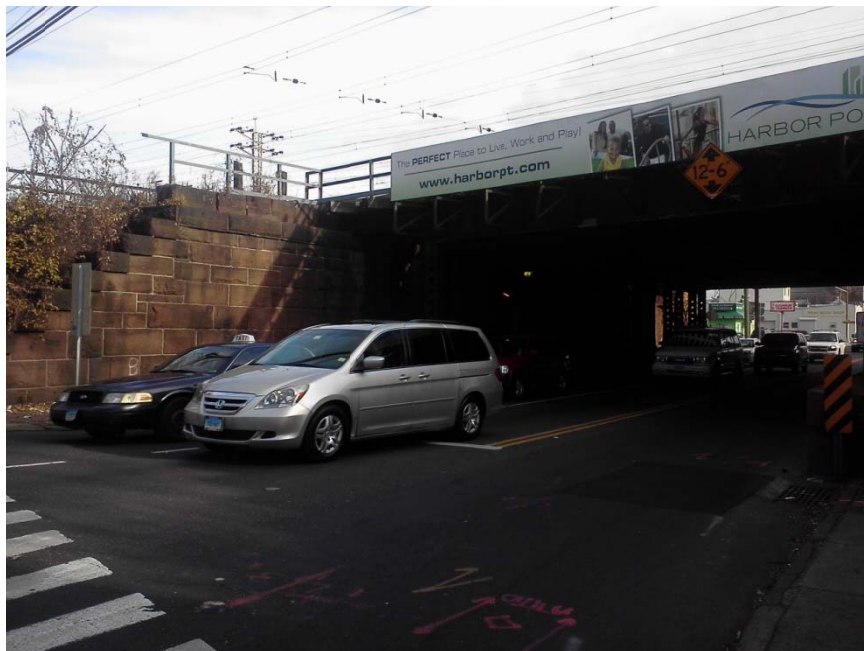
North Elevation of the Elm Street Bridge
