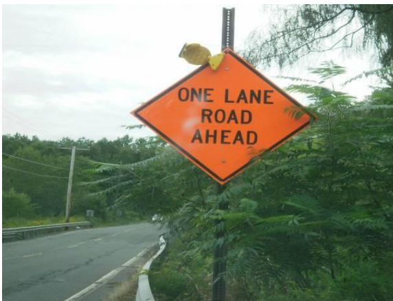
Advance construction warning sign.
