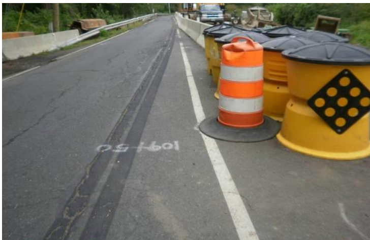
Good covering of existing pavement markings with experimental resin pavement marking
