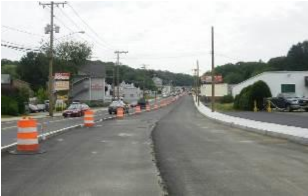
Good spacing of traffic drums.
