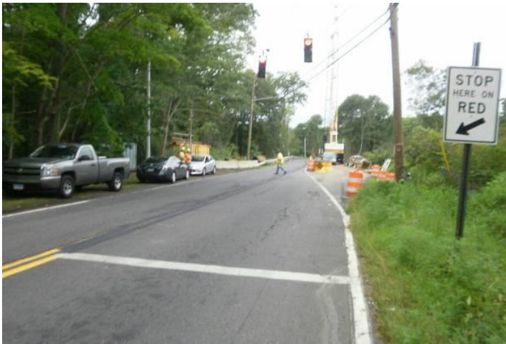
Temporary signalization installed with stop bar, sign and new edge line.
