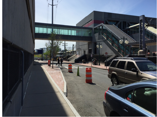
Exhibit 2-5. Stamford Station Entrance at Station Place
