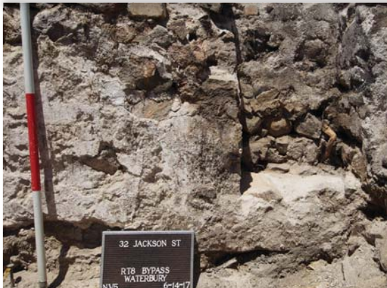
THE NICHE IN THE BASEMENT WALL AT THE COLLINS HOUSE.
