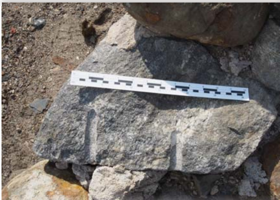
A DISPLACED GRANITE FOUNDATION STONE FOUND ON THE KELLY LOT AT NUMBER 23, WITH DRILL HOLES FROM QUARRYING.
