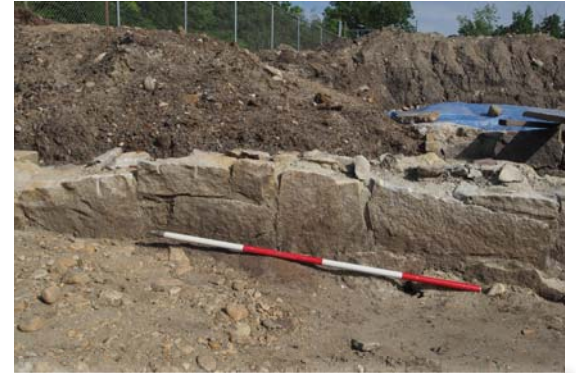
FOUNDATION MASONRY, FRONT HOUSE AT 23 JACKSON STREET, EXTERIOR OF NORTH WALL.
