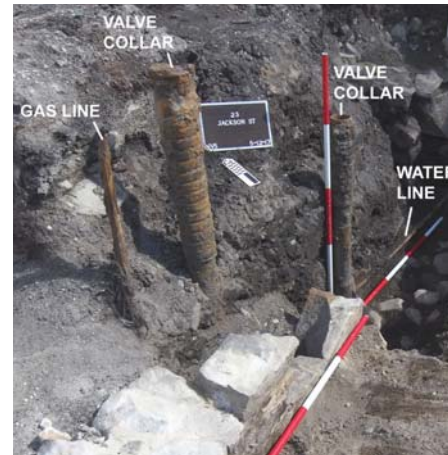
ON THE INTERIOR OF THE FOUNDATION WALL OF THE FRONT KELLY HOUSE, GAS AND WATER LINES AND TWO VALVE COLLARS WERE FOUND. THE WATER LINE EXTENDED INTO THE HOUSE FROM THE JACKSON STREET MAIN.
