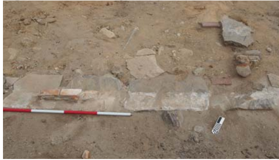
FOUNDATION OF THE MCAULIFFE HOUSE, 31 JACKSON STREET. LINE OF MORTAR SHOWS WHERE BRICKS OF THE UPPER PART OF THE FOUNDATION WERE PLACED. DISPLACED MASONRY IS RELATED TO A SIDE ENTRANCE.
