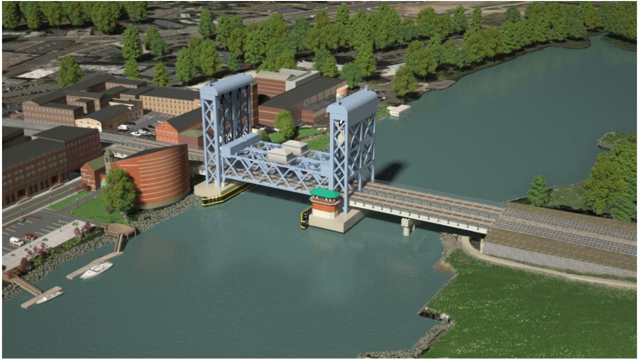
Figure ES-5—Rendering of the Short Span Vertical Lift Bridge in the Closed Position (Option 8A)
