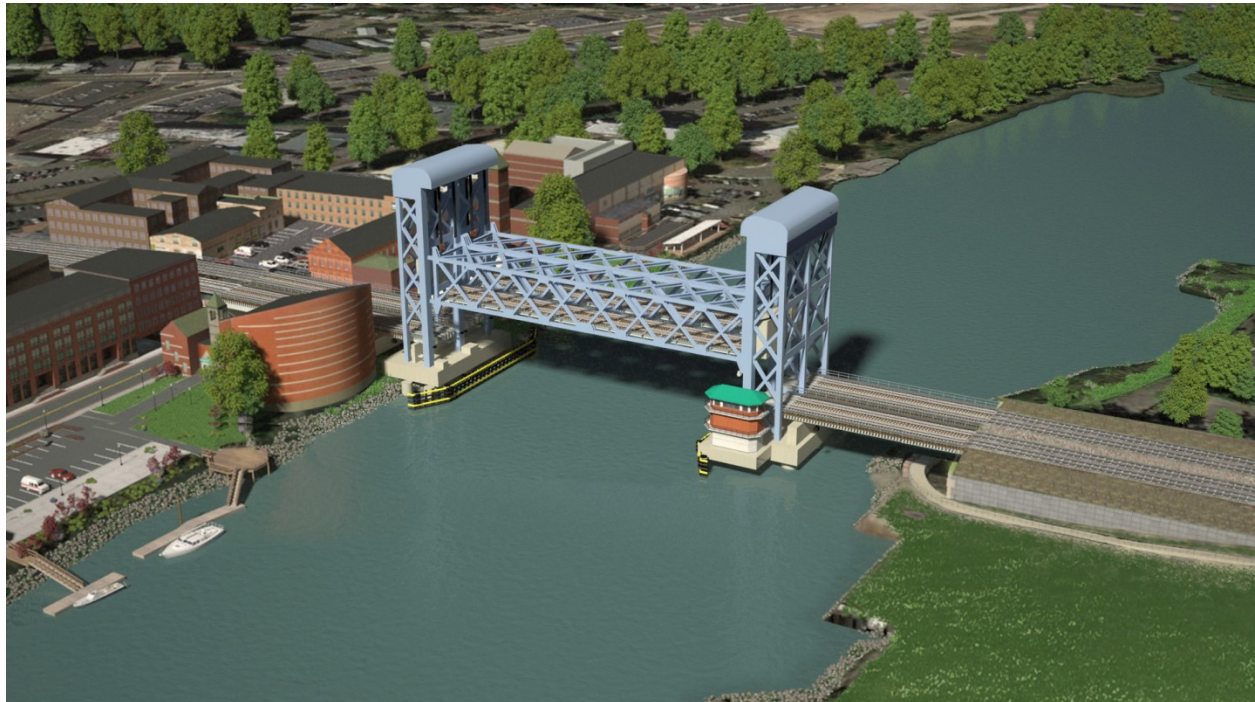
Figure ES-9—Rendering of the Long Span Vertical Lift Bridge in the Open Position (Option 11C)
