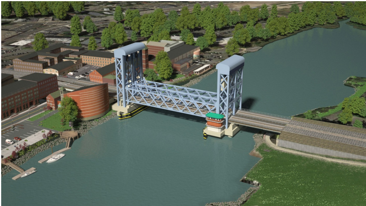
Figure ES-8—Rendering of the Long Span Vertical Lift Bridge in the Closed Position (Option 11C)
