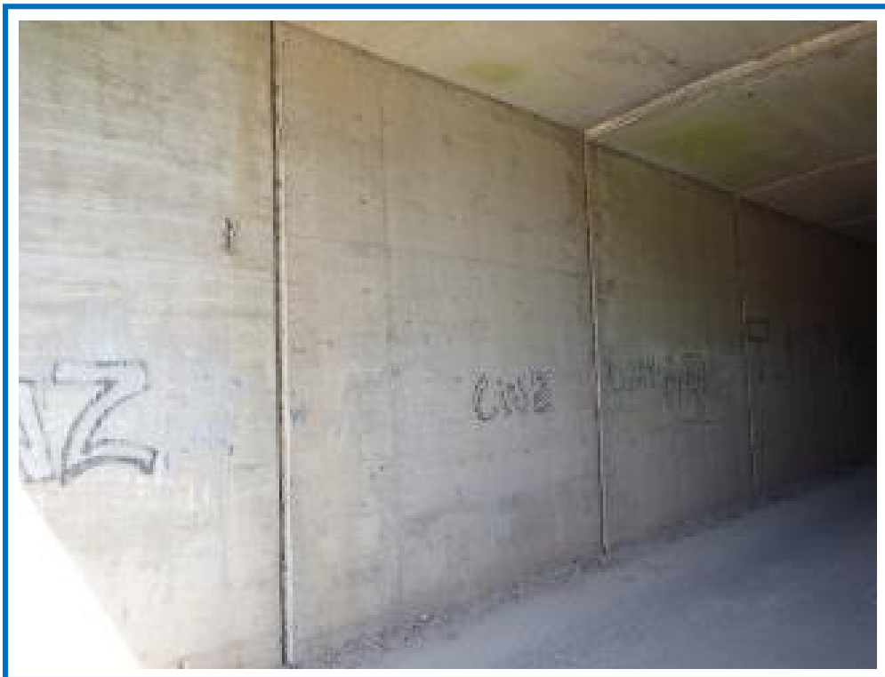
Panels 1 thru 4 North Wall
