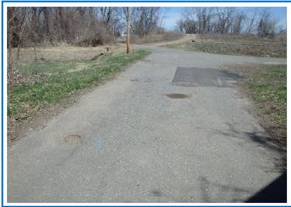
Looking East from Bridge (Note: Water and sewer manholes in roadway)
