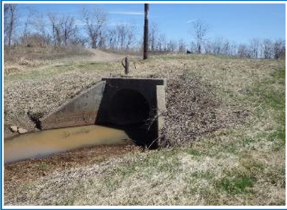
Drainage Structure to East of Bridge
