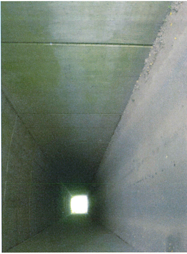
Photo # 6 A VIEW THRU THE STRUCTURE.
