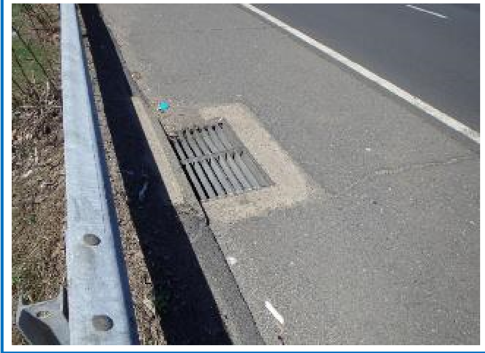
Catch Basin at NW Corner
