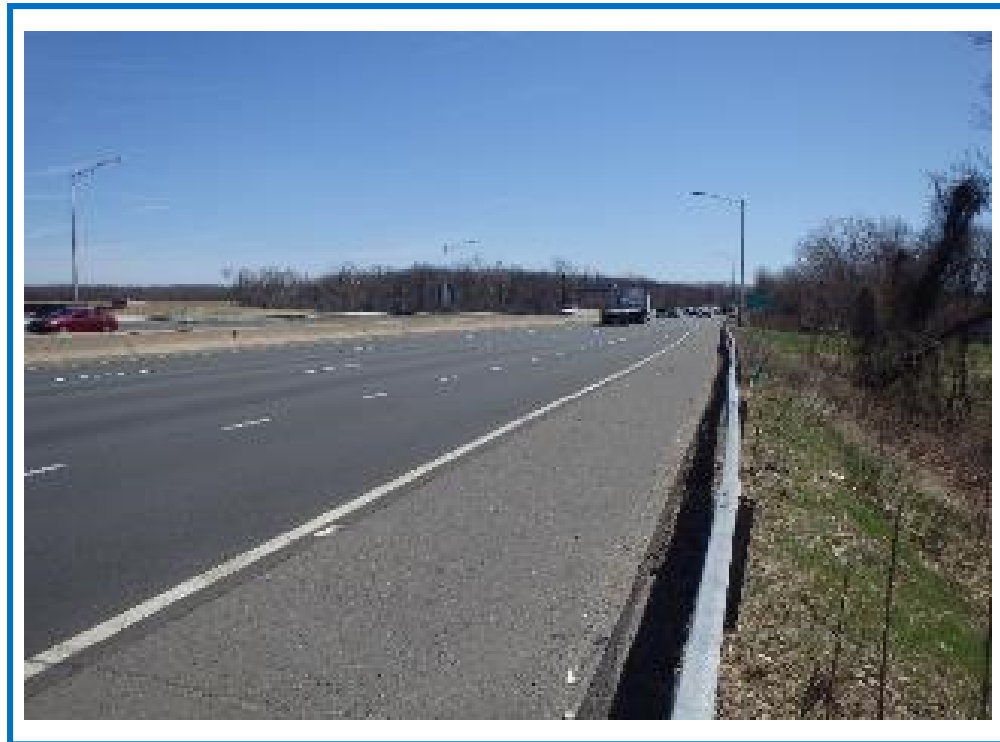
Bridge from South Approach (Note: Interstate 91 Northbound)
