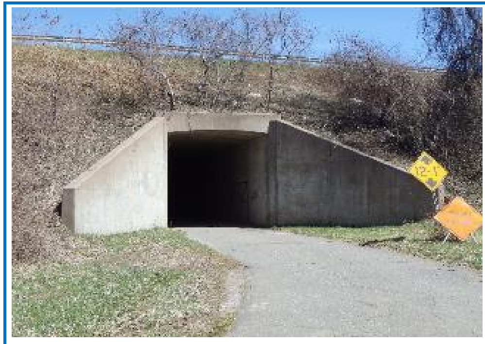
West Elevation of Bridge No. 02555
