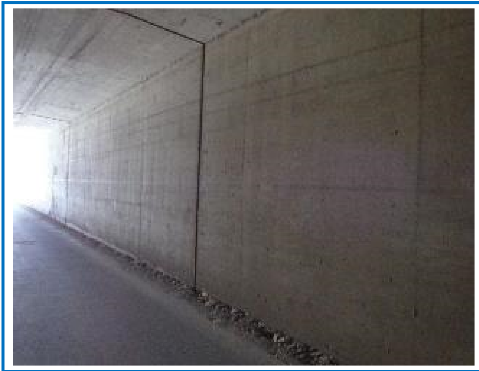
Panel 6 South Wall
