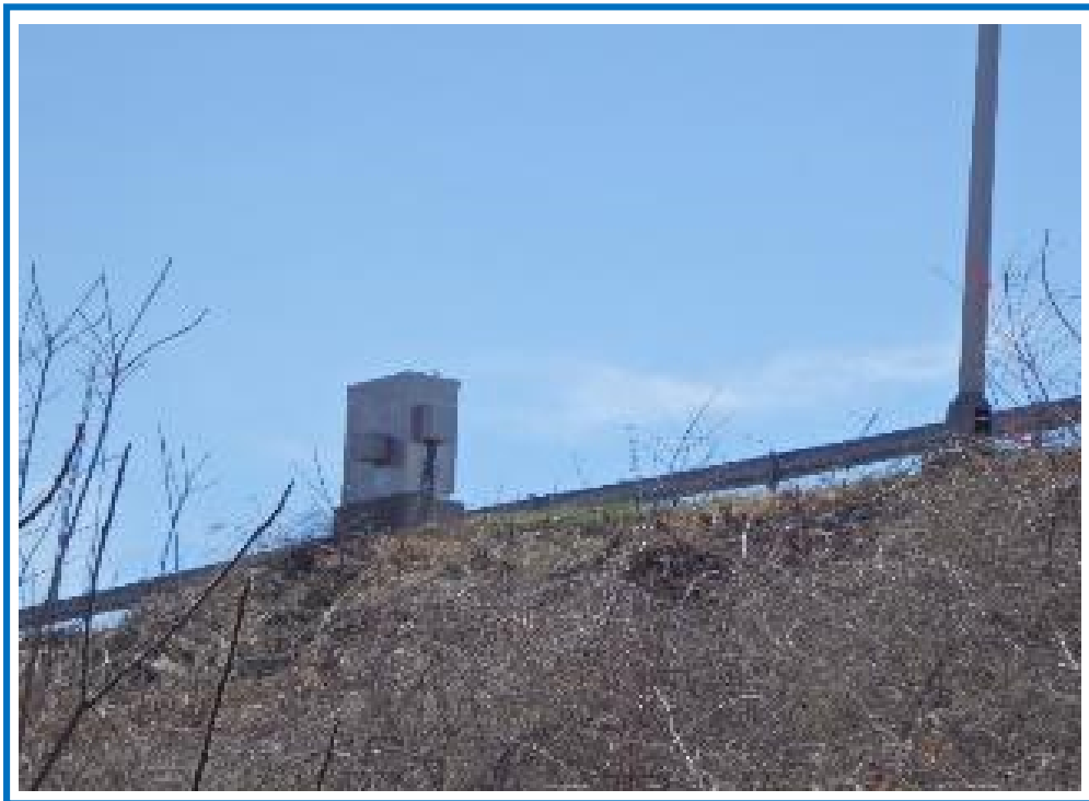
Service Cabinet at Northeast Corner
