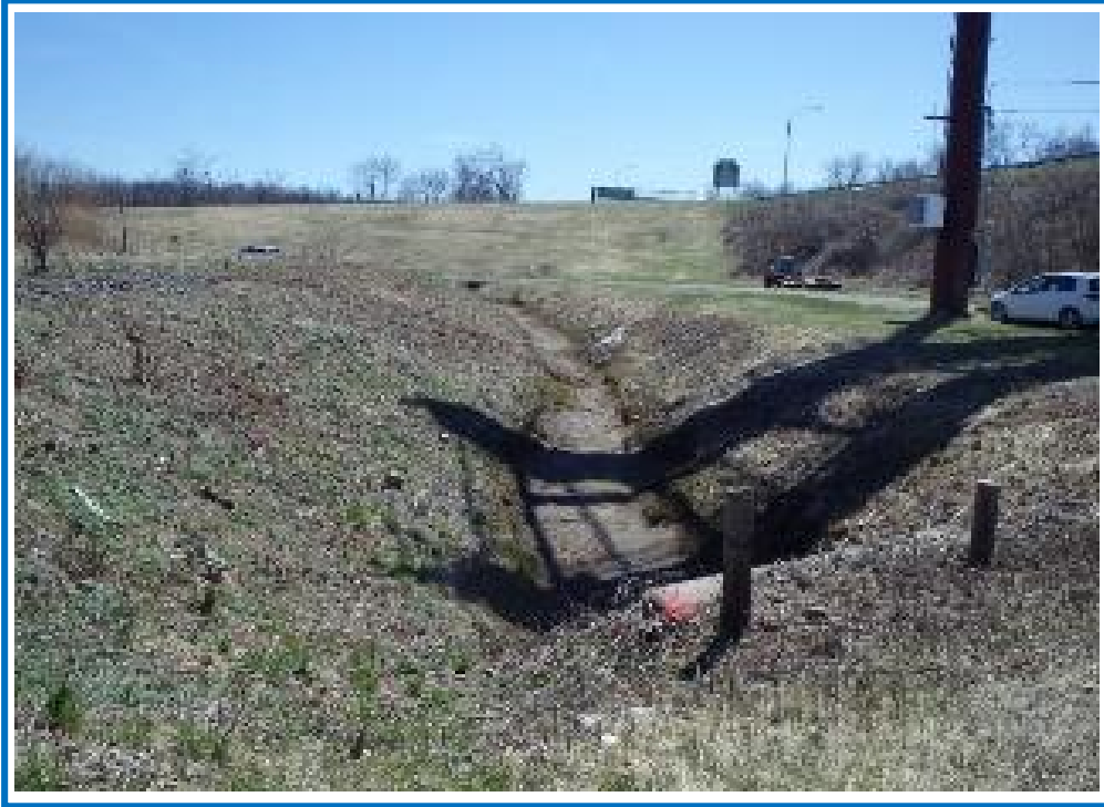
Drainage Channel East of Bridge Looking South
