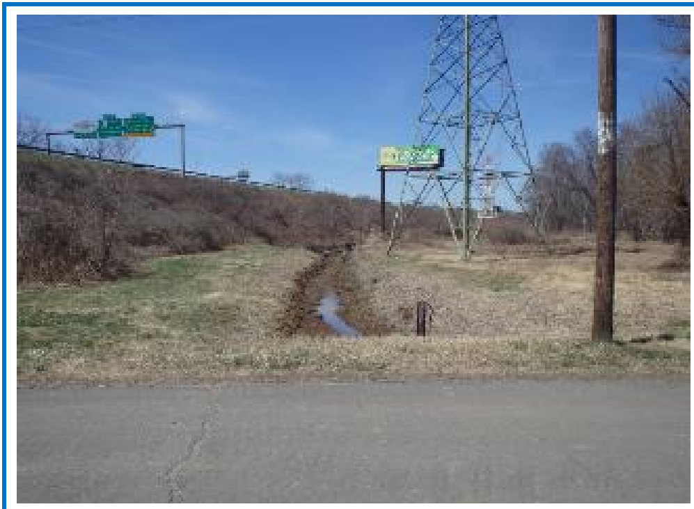
Drainage Channel East of Bridge Looking North
