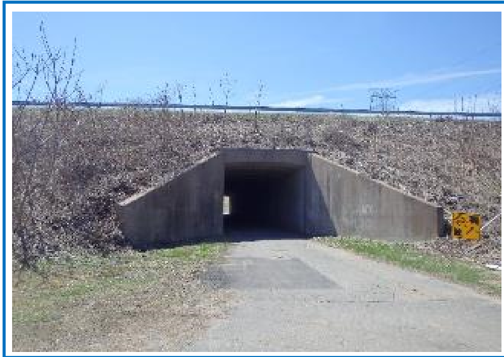
East Elevation of Bridge No. 02555
