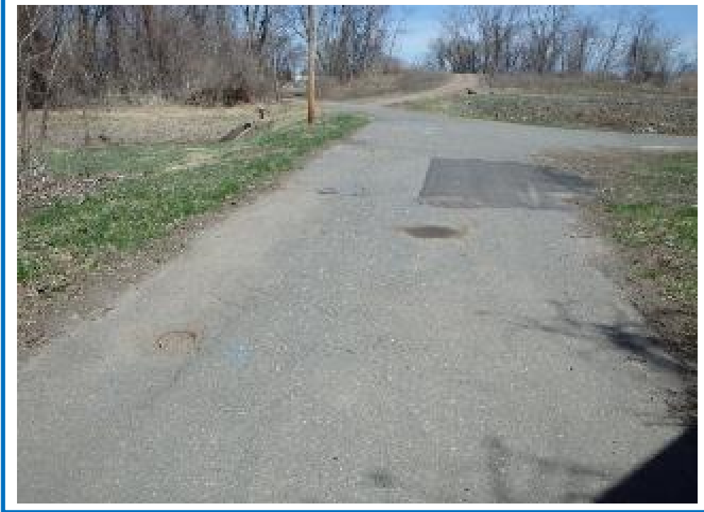
Looking East from Bridge (Note: Water and sewer manholes in roadway)
