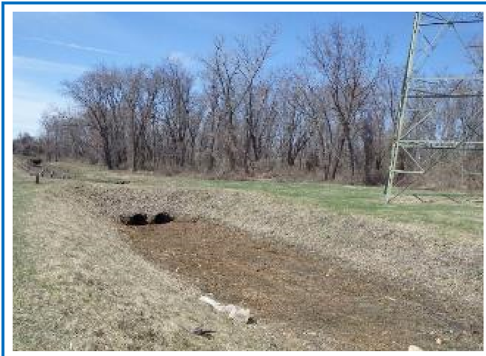
Drainage Structure Channel Looking West from Bridge
