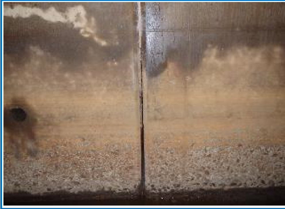
North Abutment Elevation Joint at South Wall between Panels 9 and 10
