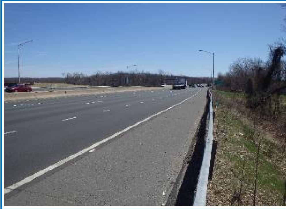
Bridge from North Approach (Note: I-91 Southbound)
