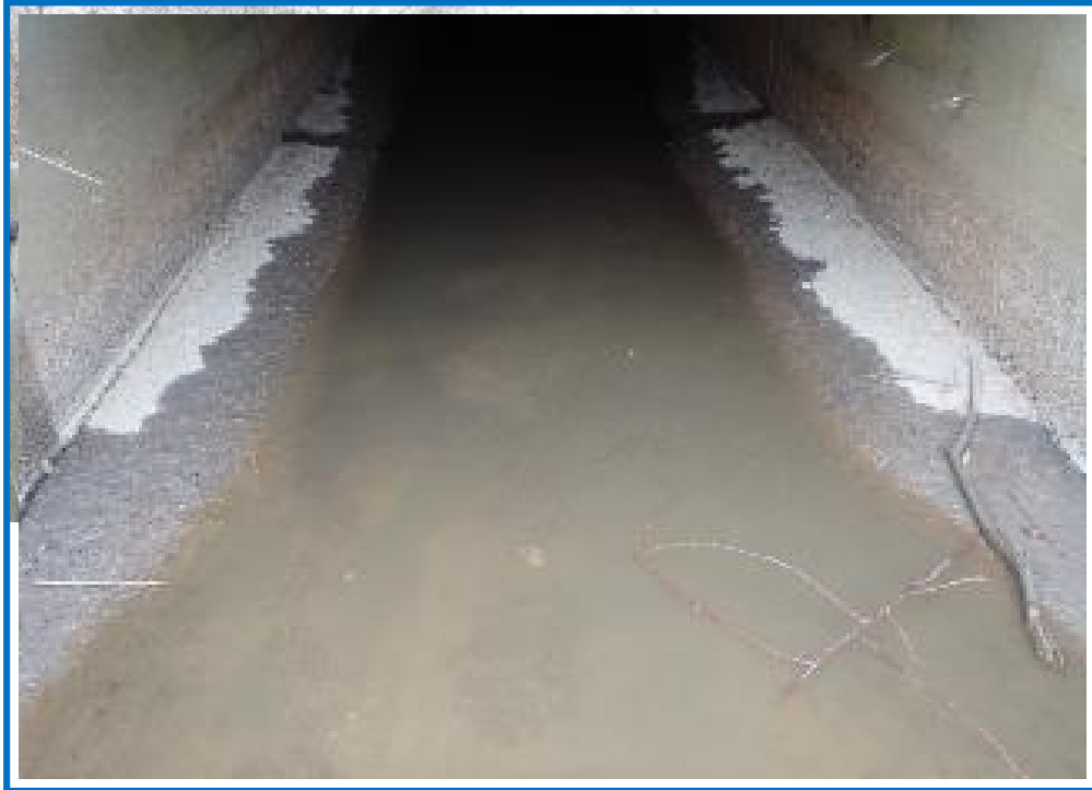
Culvert Bottom at West End
