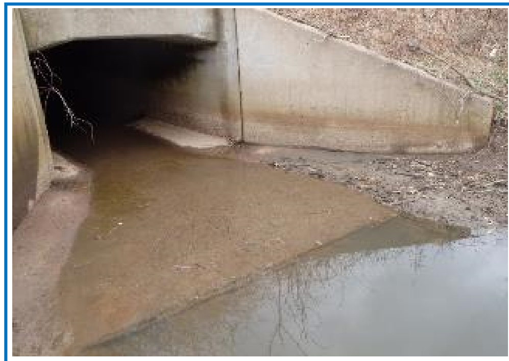
East Elevation of Bridge No. 03244
