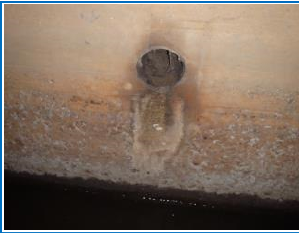
Typical 4" Weep Hole at North Panel 6
