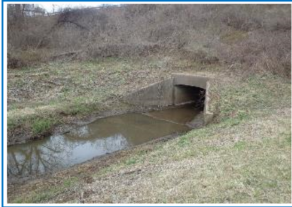
West Elevation of Bridge No. 03244
