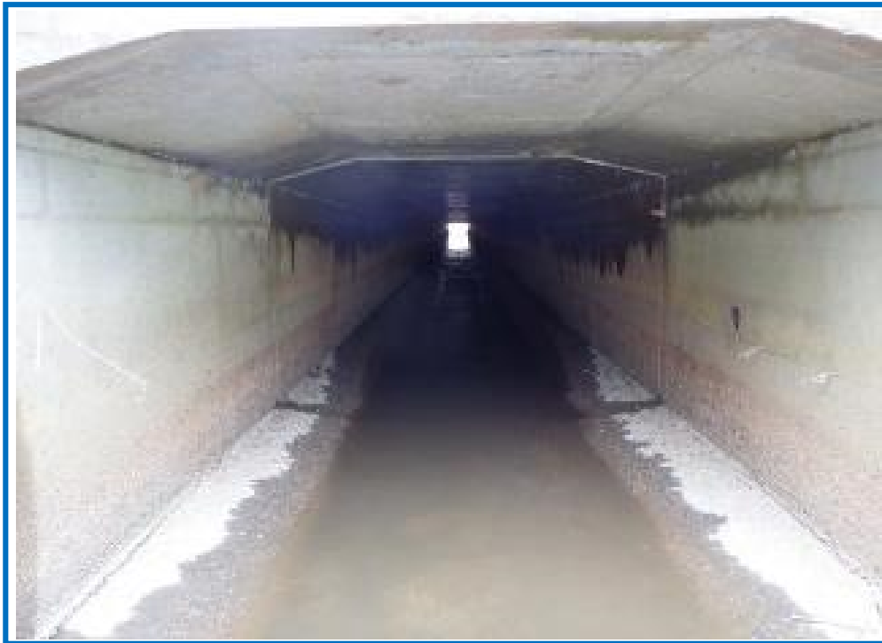
Looking East Through Culvert from West End
