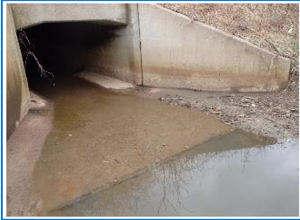
Apron at East End
