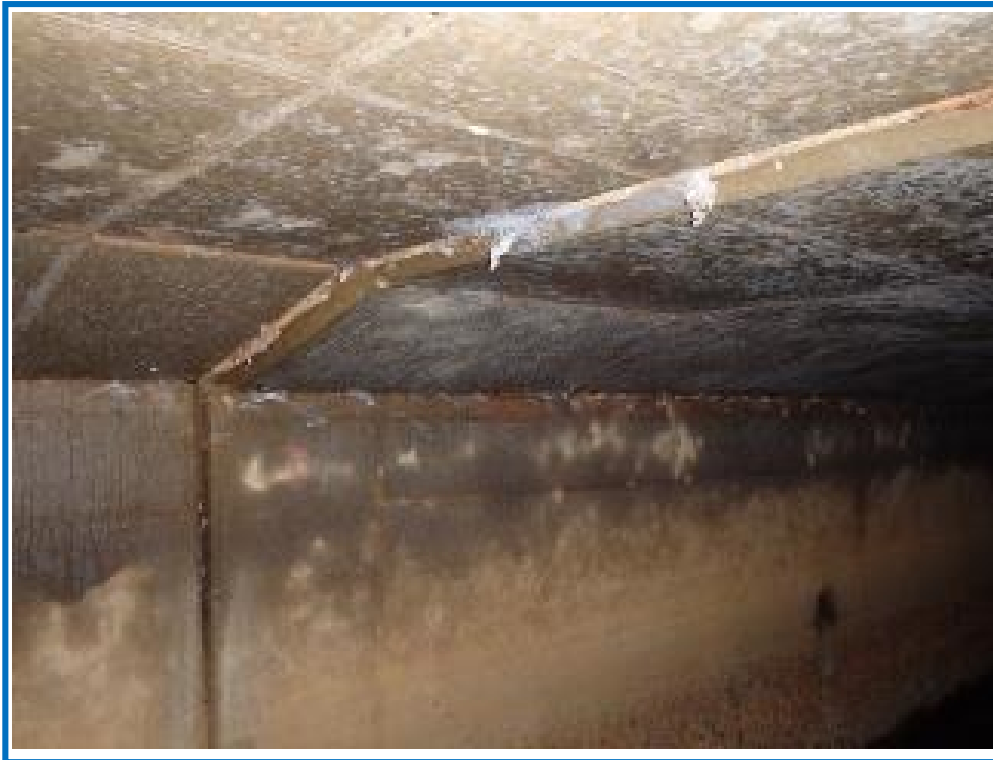
Joint 2 Top Panel (Note: Typical misalignment up to ½")
