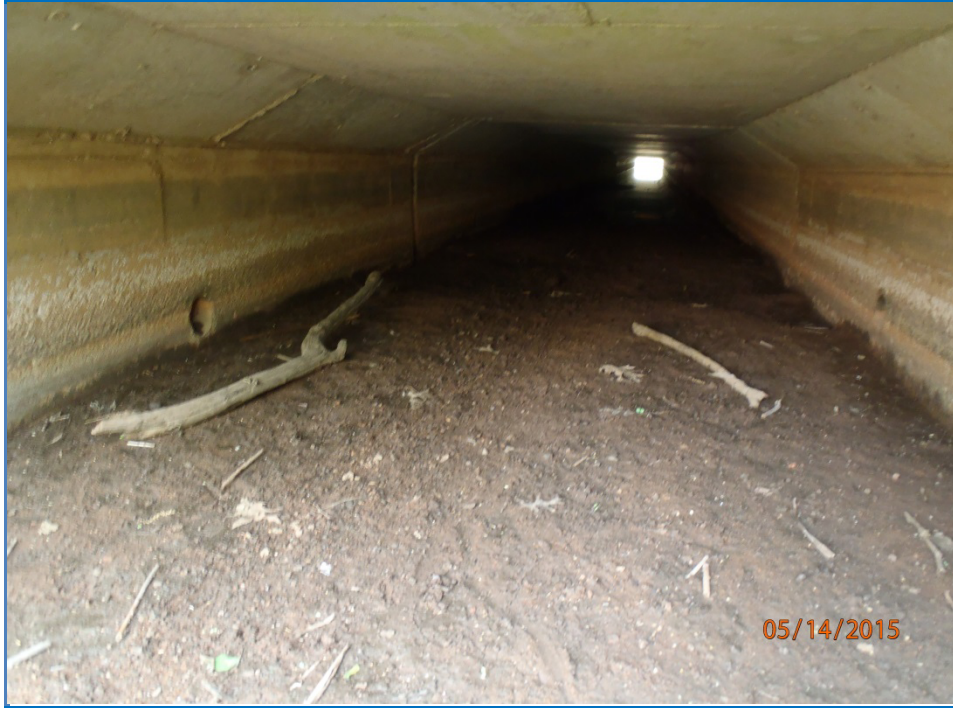
7: Inside culvert Note sediment and debris
