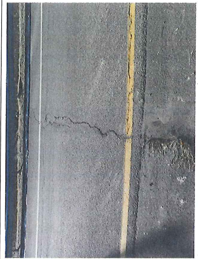
Photo # 10: I-91 TR 828, Bituminous Concrete Pavement Over the Culvert, Looking South
