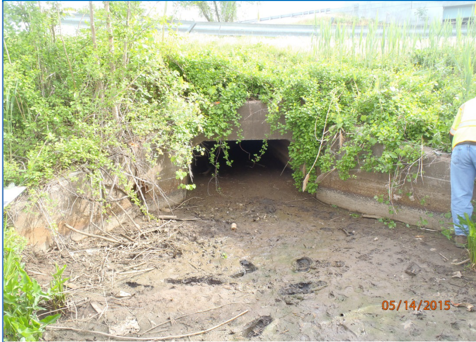
1: South Endwall, Outlet. Note CMP outlet at SW Wingwall
