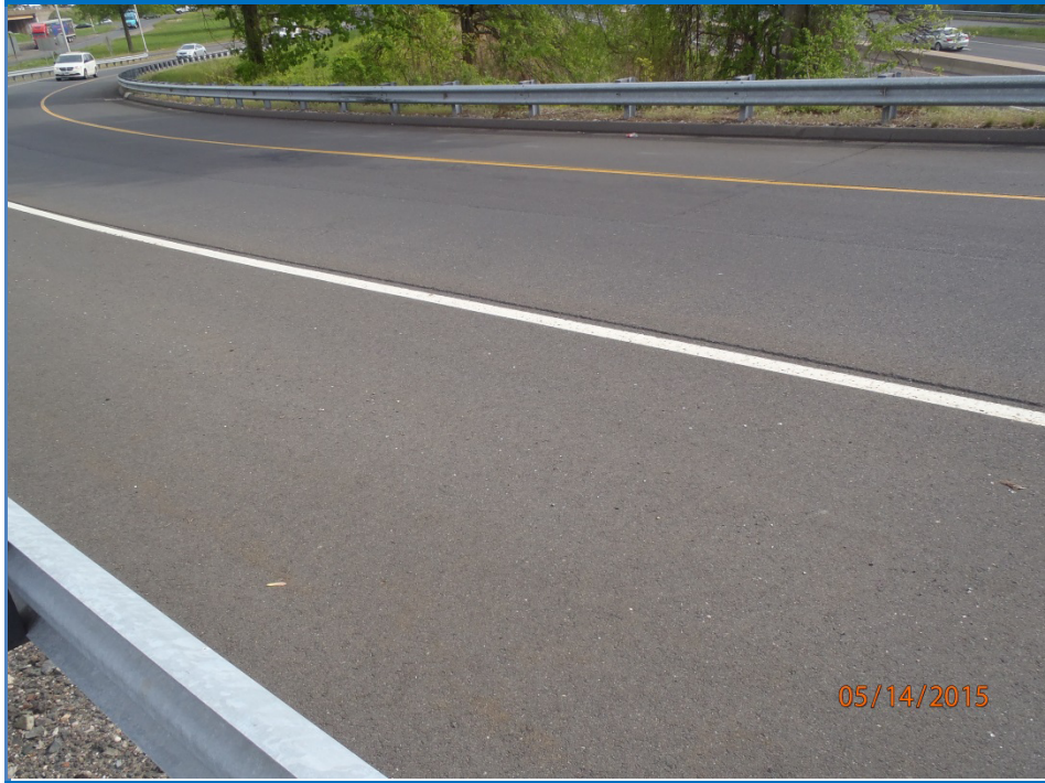
3: TR 15-191, Looking northerly up off-ramp
