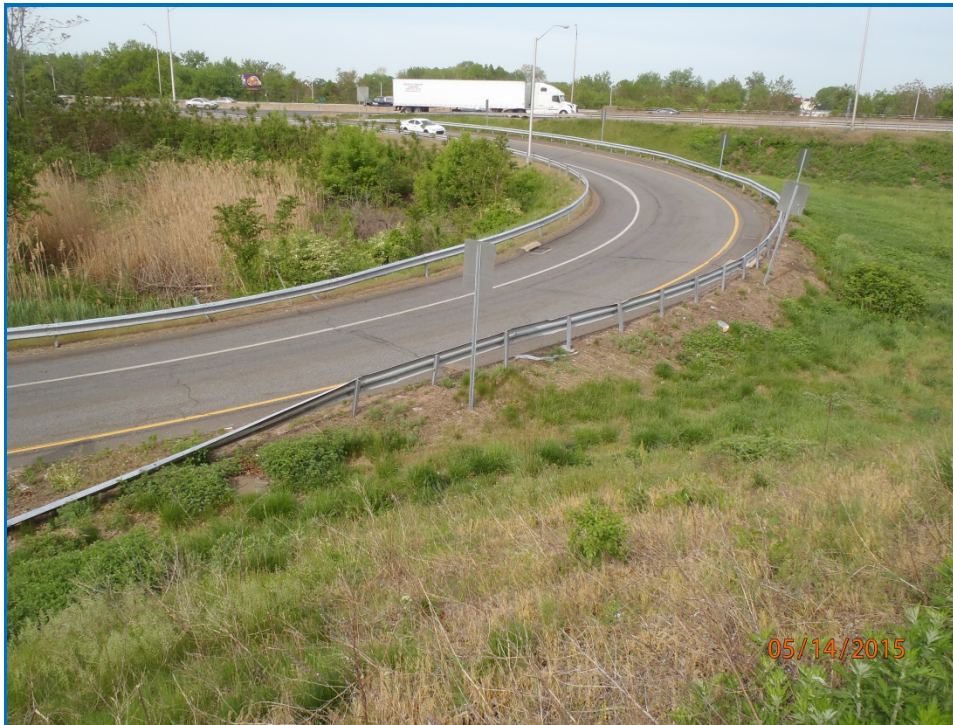
4: TR-828, Looking westerly towards I-91
