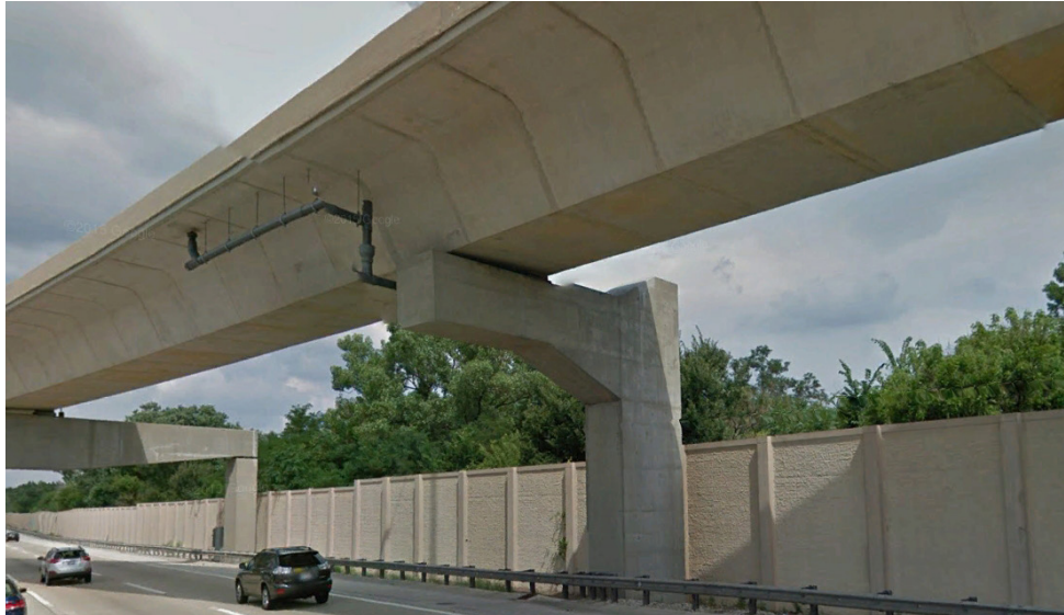
Figure DS4.1: Cantilever Pier I-355 / I-88 Interchange – Downers Grove, IL
