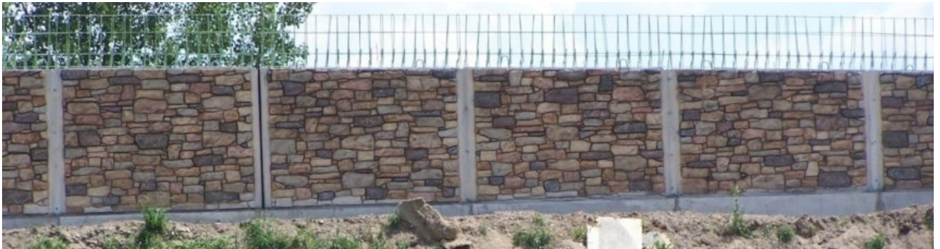
Figure DS5.2: Precast Concrete Wingwalls
