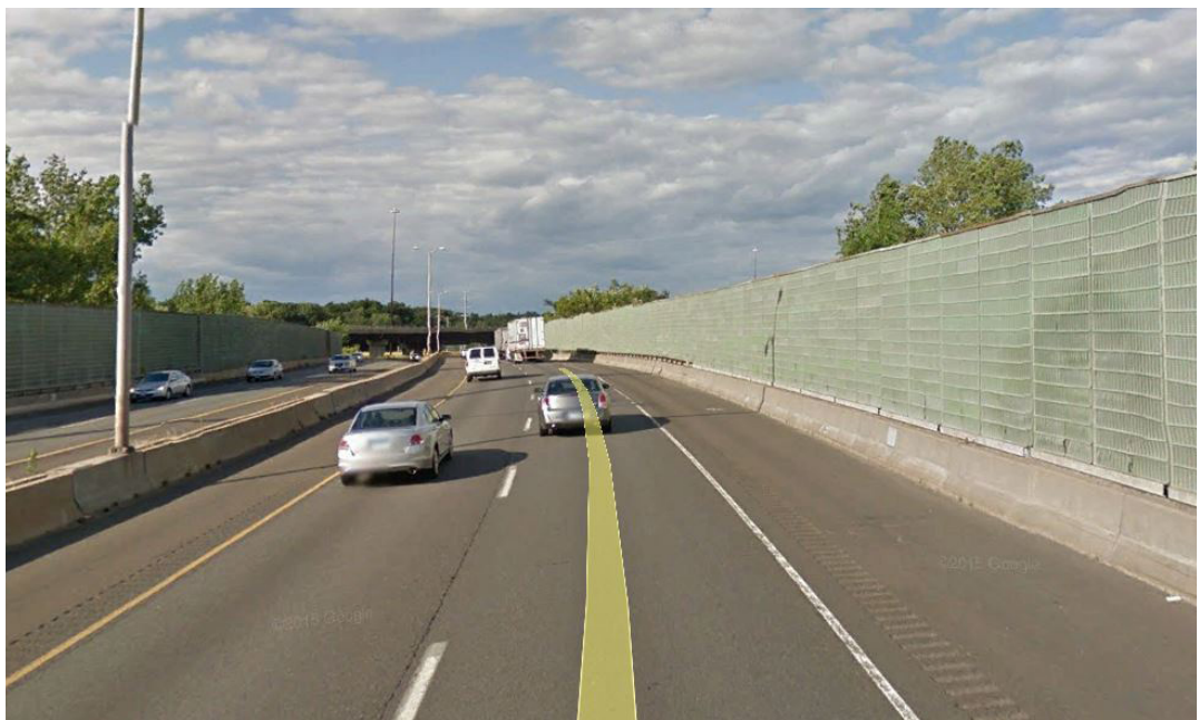
Figure P4.1: Reconstructed Noise Barrier at South Curb Line from Exit 91 to Project Limit
