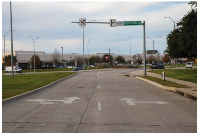
LOCATION: N Riverside Drive/Northern Cross Boulevard, Fort Worth, Texas. SOURCE: Lee Rodegerdts.
