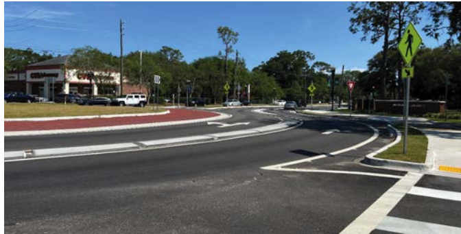
LOCATION: University Boulevard/Merrill Road, Jacksonville, Florida. SOURCE: Federal Highway Administration.
