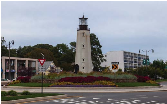
LOCATION: Rehoboth Avenue/Grove Street/Columbia Avenue, Rehoboth Beach, Delaware. SOURCE: Lee Rodegerdts.
