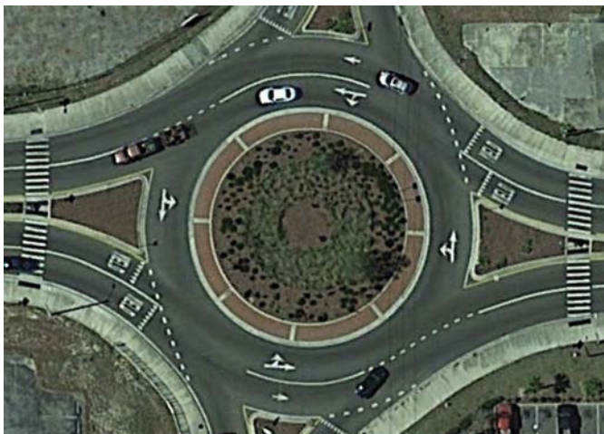
LOCATION: 40th Street/East Yukon Street, Tampa, Florida. SOURCE: Google Earth.
