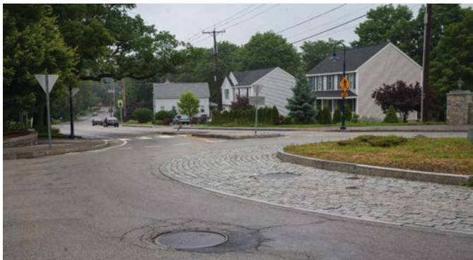
Exhibit 13.3. Example of flush truck apron using pavers.
