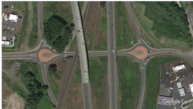
LOCATION: Dike Access Road/I-5 Ramps, Woodland, Washington. SOURCE: Google Earth.
