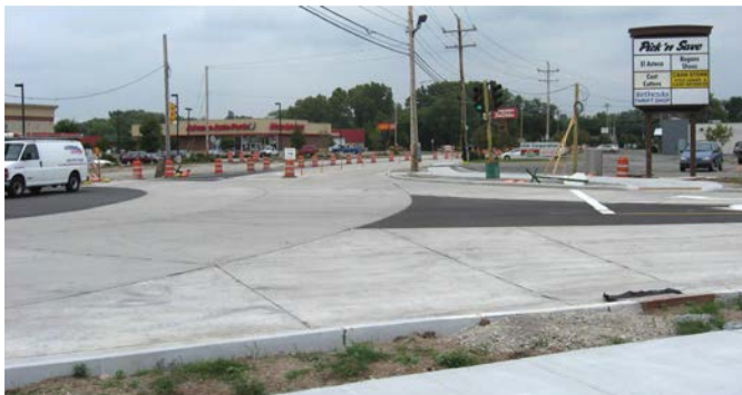
Exhibit 15.2. Example construction with temporary signals and pavement.
