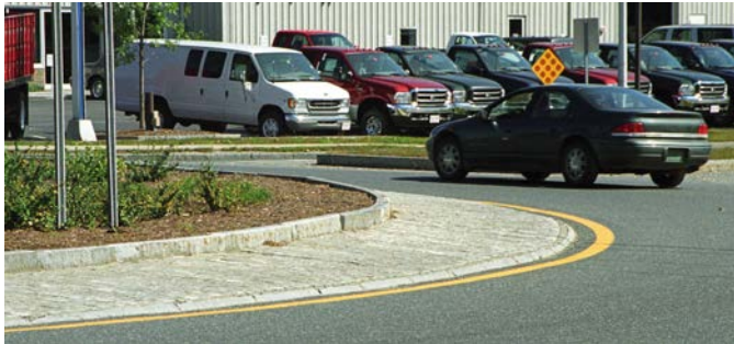
Exhibit 13.2. Example of raised truck apron using pavers.
