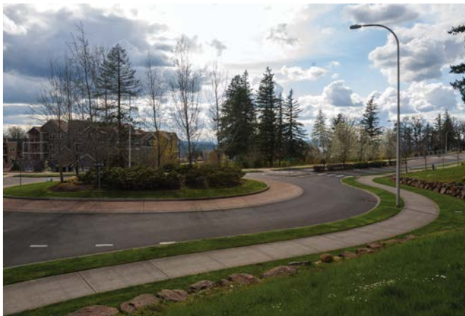
LOCATION: Monterey Avenue/Causey Avenue, Clackamas, Oregon. SOURCE: Lee Rodegerdts.
