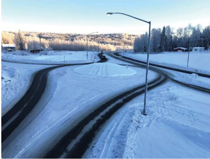
LOCATION: Chena Hot Springs Road/Steese Highway Northbound Ramps, Fairbanks, Alaska. SOURCE: Gary Katsion.
