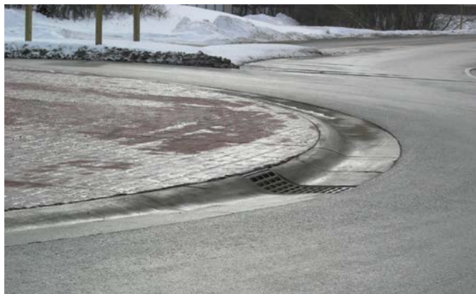
LOCATION: De Pere, Wisconsin. SOURCE: Wisconsin Department of Transportation.
