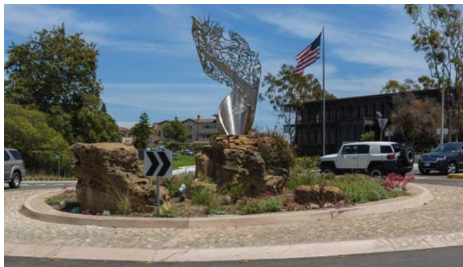
NOTE: Boulders should be constructed of frangible materials. LOCATION: Carlsbad Boulevard/State Street, Carlsbad, California. SOURCE: Lee Rodegerdts.
