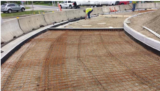
LOCATION: Route 9–Route 126/I-95 Northbound Ramps/Service Plaza Drive, West Gardiner, Maine. SOURCE: Jonathan French.
