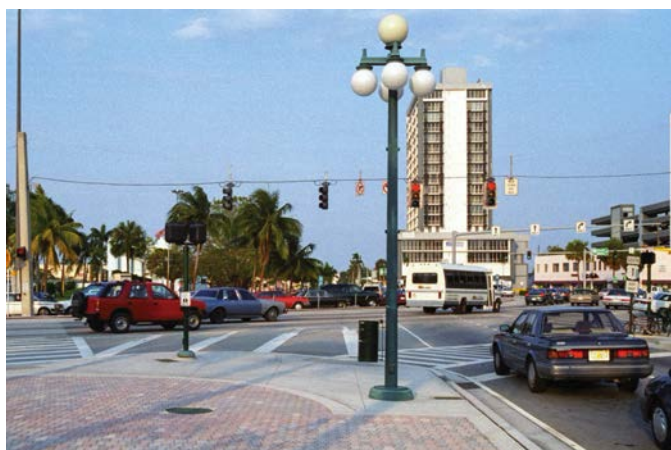
Exhibit 2.5. Example of signalized traffic circle.
