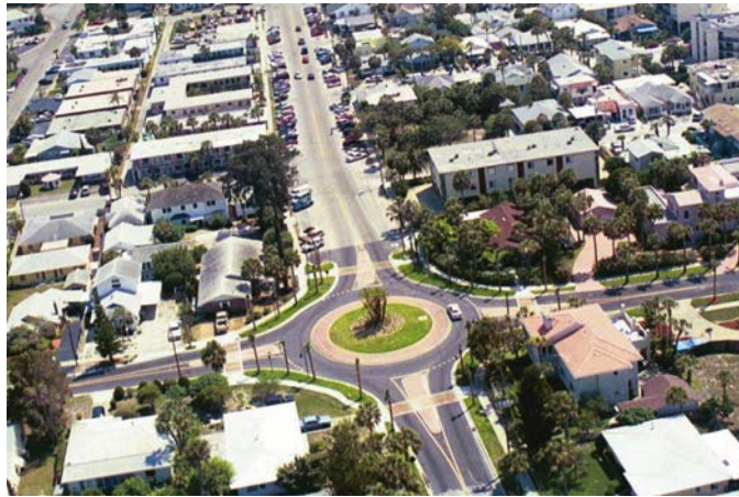
LOCATION: Mandalay Avenue/Acacia Street, Clearwater Beach, Florida. SOURCE: City of Clearwater, Florida, as shown in NCHRP Report 672 (1) .
