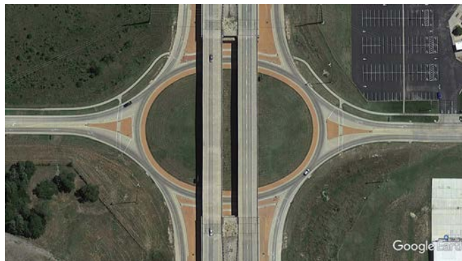
LOCATION: S. Anderson Road/US 50 Ramps, Newton, Kansas. SOURCE: Google Earth.
