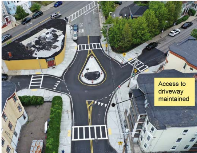
LOCATION: Southern Avenue/Whitfield Street, Boston, Massachusetts. SOURCE: Kittelson & Associates, Inc.
