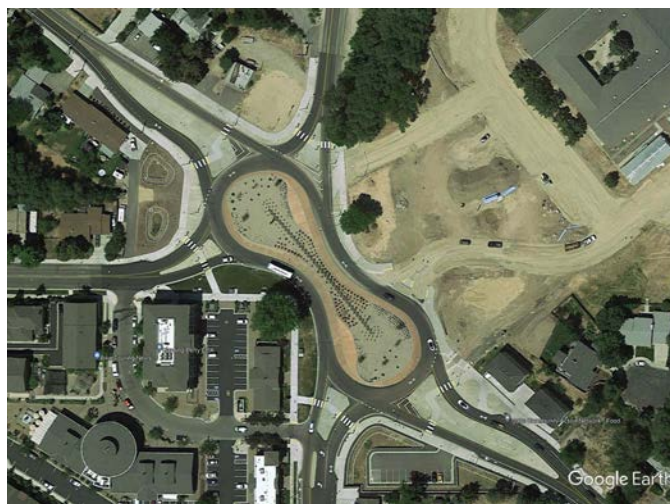
LOCATION: W Hill Road/N 36th Street/W Catalpa Drive, Boise, Idaho. SOURCE: Google Earth.
