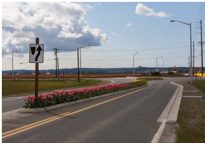
Exhibit 10.111. Example of external curbing introduced at the leading end of a splitter island.
