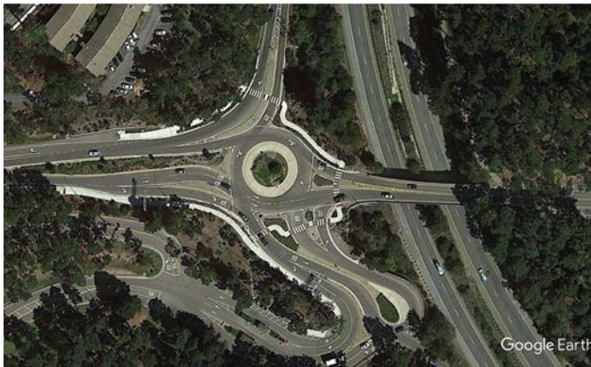
LOCATION: SR 68 / SR 1 Off-Ramp/17 Mile Drive, Monterey, California. SOURCE: Google Earth.
