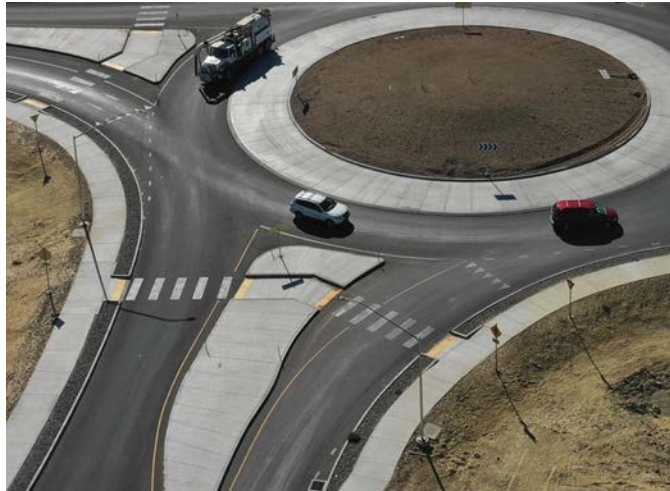
LOCATION: OR 126/SW Tom McCall Road, Prineville, Oregon. SOURCE: Kittelson & Associates, Inc.
