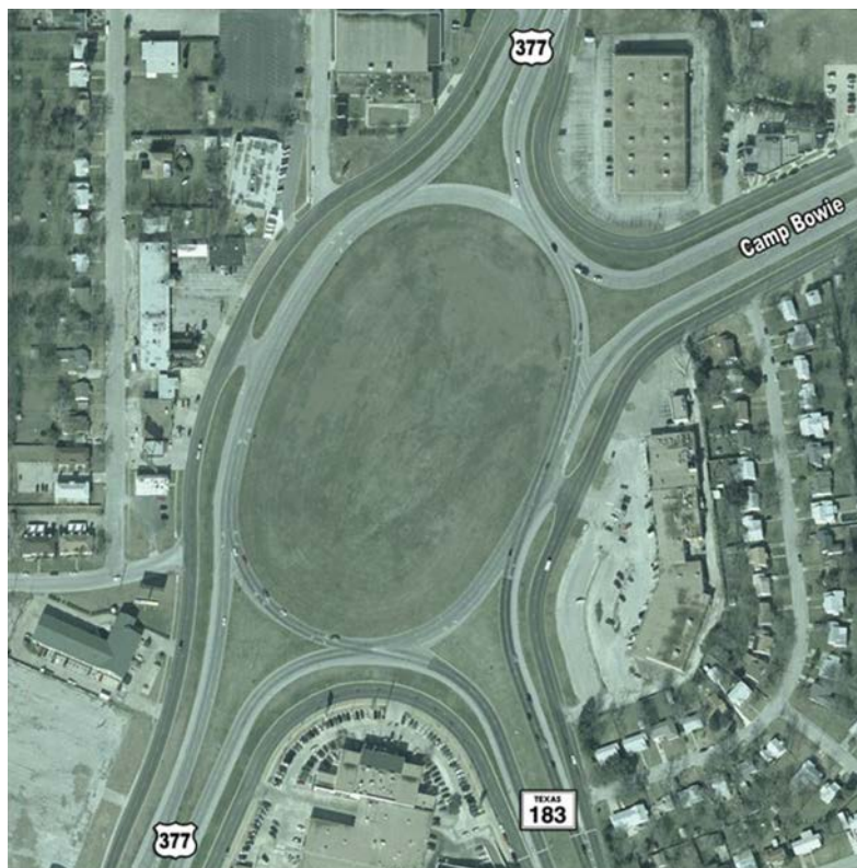
LOCATION: US 377/TX 183/Camp Bowie, Fort Worth, Texas. SOURCE: City of Fort Worth, Texas, as shown in NCHRP Report 672 (1) .
