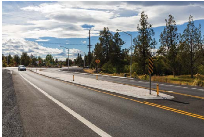
LOCATION: Powell Butte Highway/Neff Road/Alfalfa Market Road, Deschutes County, Oregon. SOURCE: Lee Rodegerdts.
