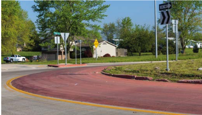
LOCATION: SR 13/Old SR 13/NW 435 Road, Warrensburg, Missouri. SOURCE: Lee Rodegerdts.
