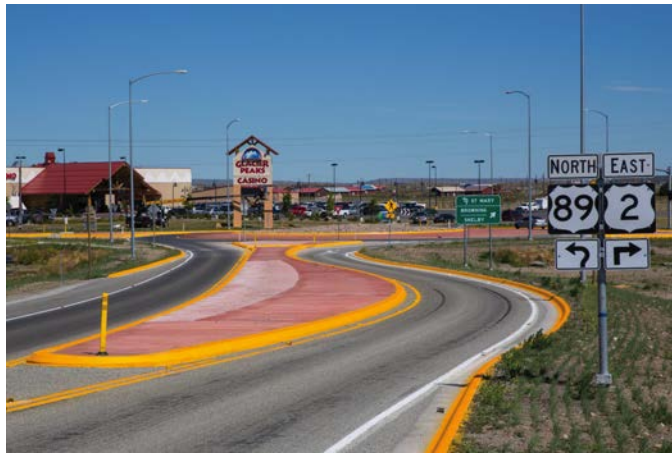
LOCATION: US 2/US 89, Browning, Montana. SOURCE: Lee Rodegerdts.
