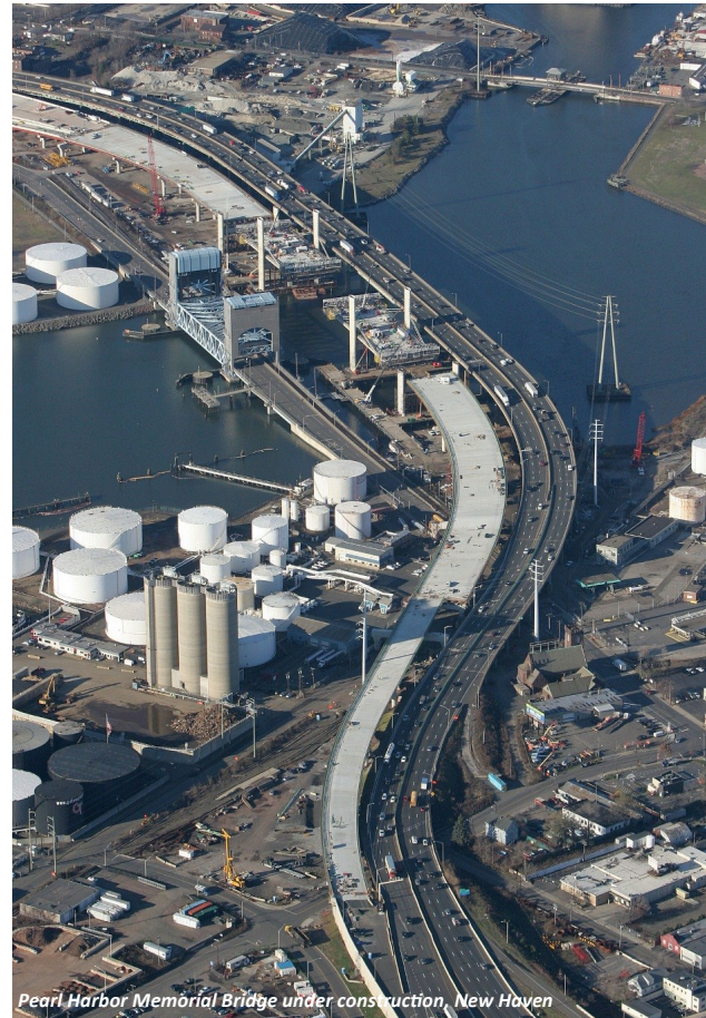
Pearl Harbor Memorial Bridge under construction, New Haven
