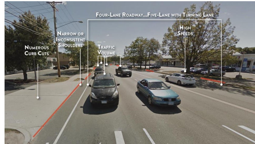
Figure 6: Black Rock Turnpike Typical Conditions
