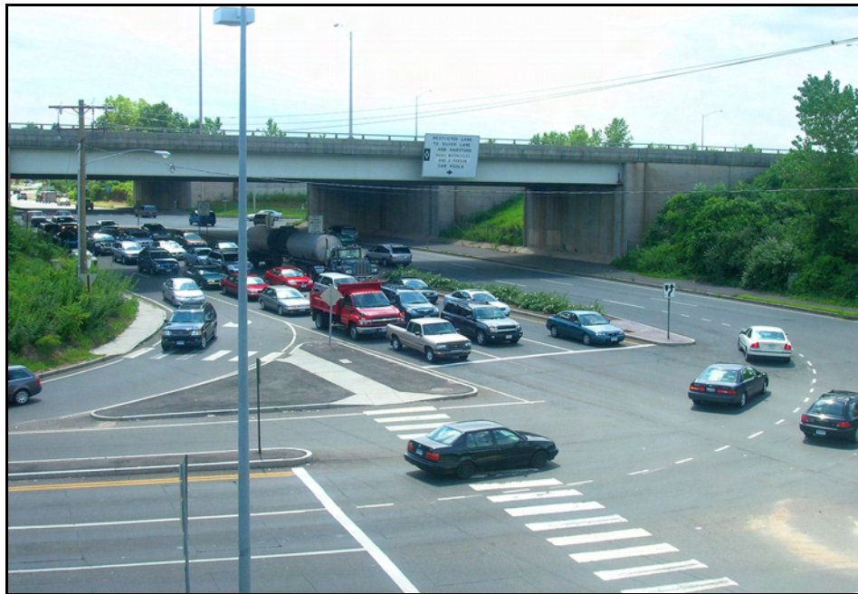
Figure 2-15 Buckland Street northbound at Pavilion Drive, with I-84 overpass
