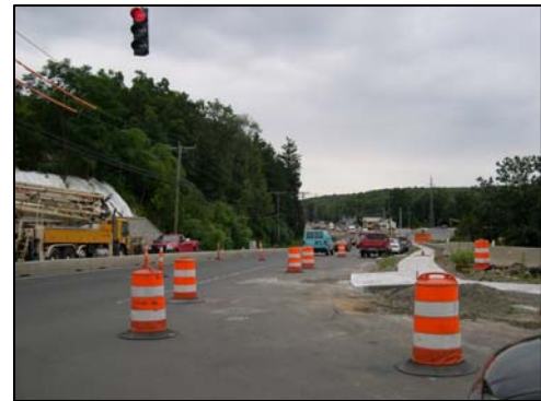
Construction on Route 7 in Wilton (August 6, 2009)
