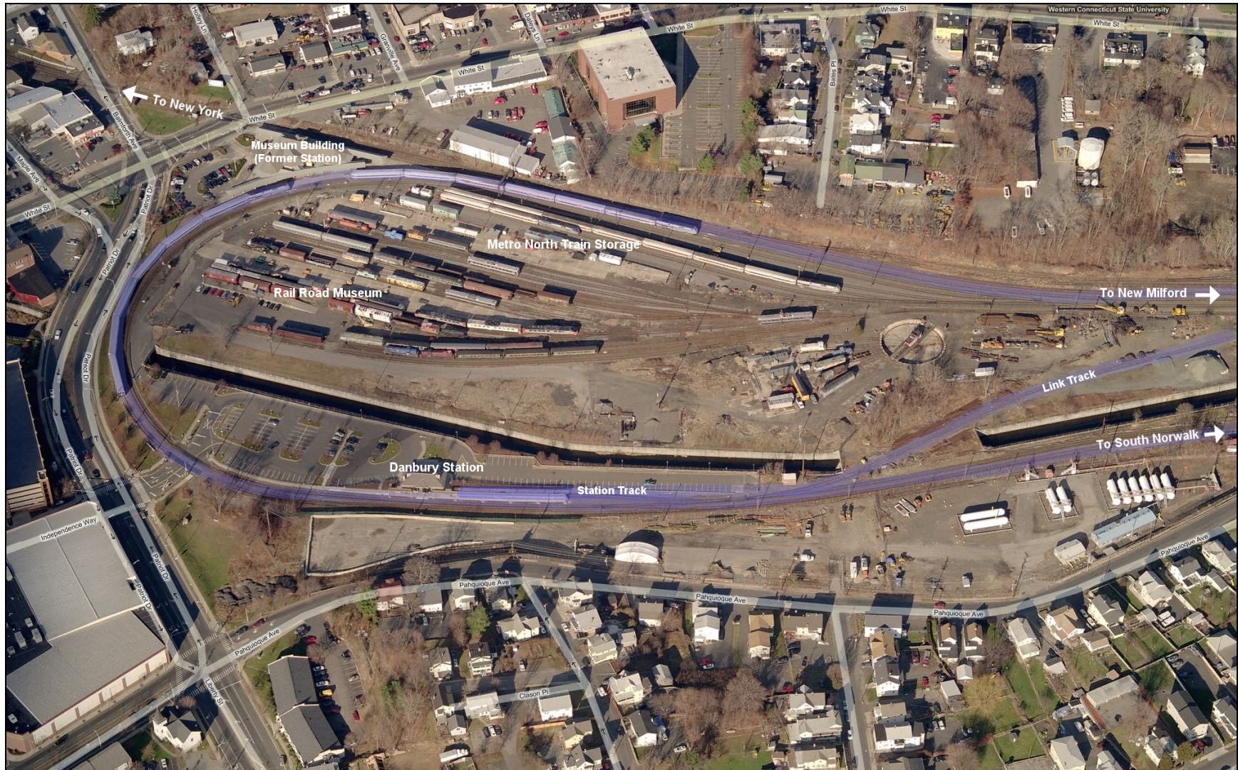
Figure 9: Danbury Rail Yards
