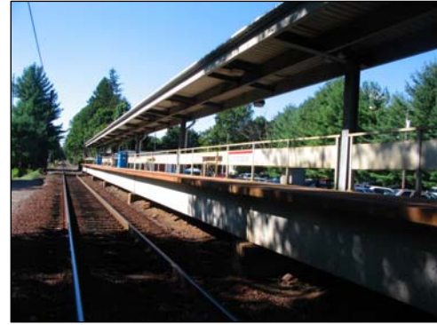
Cannondale Station Platform
