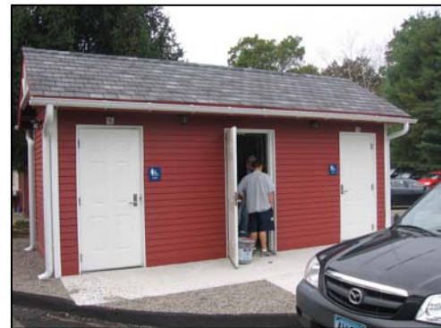
Bathroom Facilities at Cannondale Station
