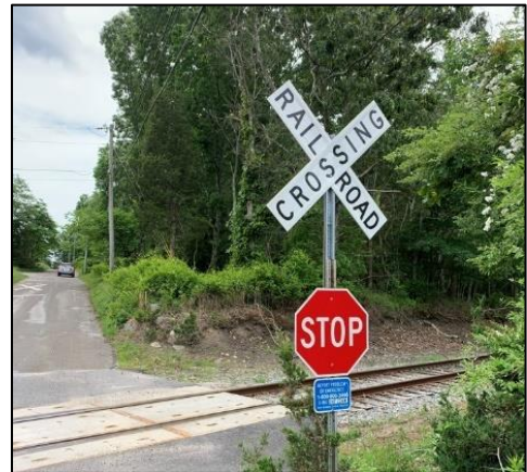
Figure 42: Unfenced Private Grade Crossing - Lower Bartlett Road (MP 5.05)
