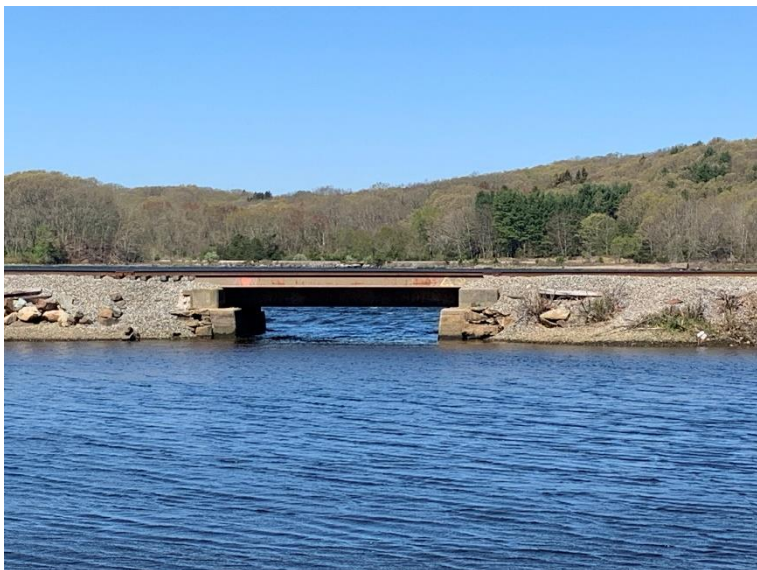
Figure 119: MP 7.09 - UG Bridge - Stoddard Cove
