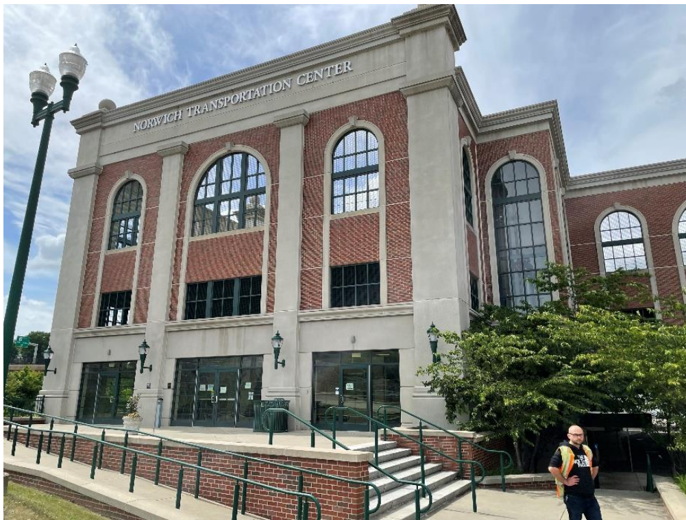
Figure 92: MP 13.21 – Passenger Facility - Norwich Intermodal Center - Main Entrance
