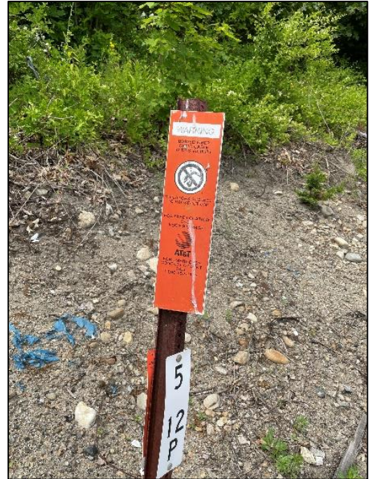
Figure 44: Existing Fiber Optic Cable Warning Post (AT&T)
