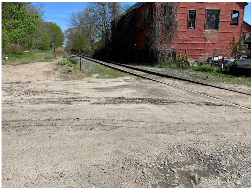
Figure 35: MP 1.79 - Grade Crossing - Farnsworth Street - Old Thames Shipyard
