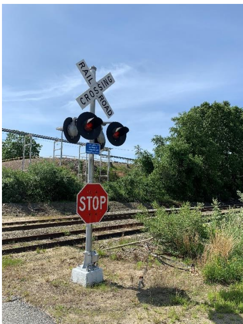
Figure 109: MP 6.08 - Grade Crossing - DOW Chemical
