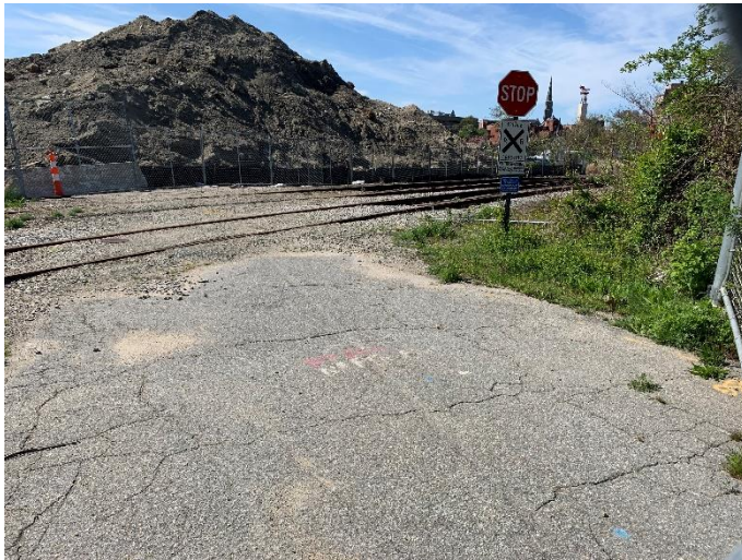
Figure 11: MP 0.40 – Grade Crossing - Thomas Griffin Road - Private Grade Crossing
