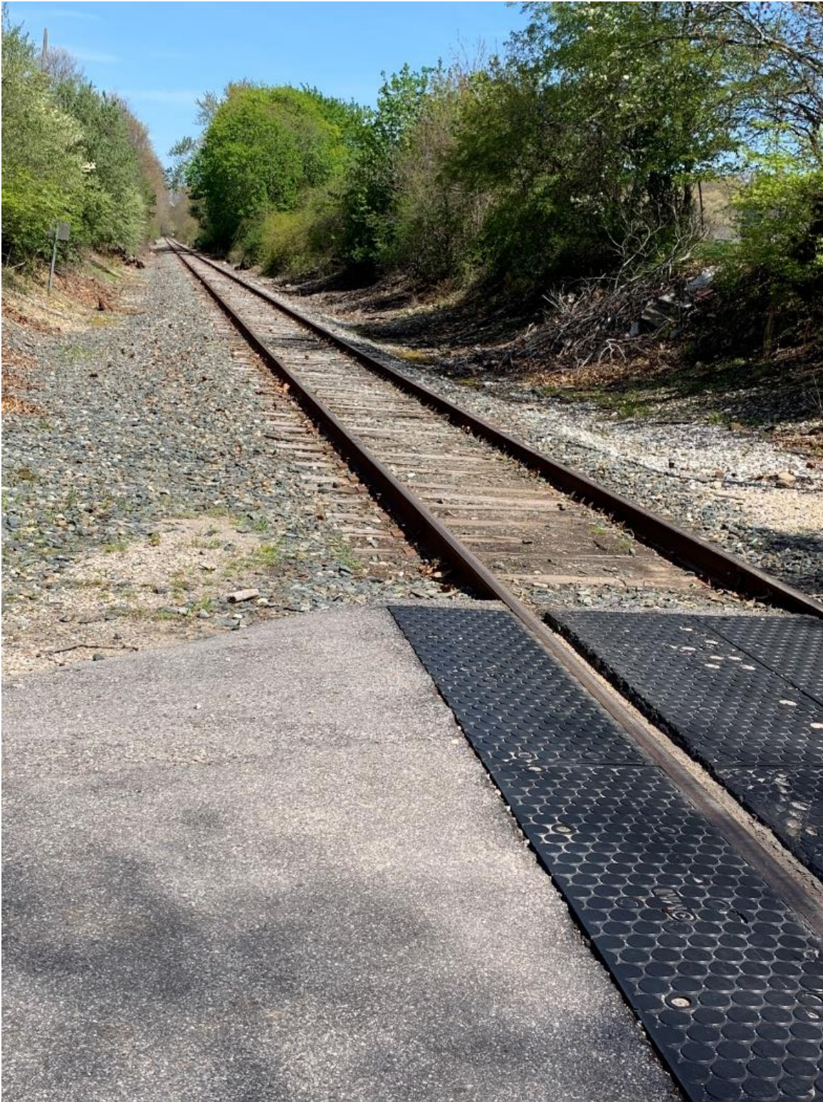
Figure 42: MP 2.37 - Grade Crossing - Bentham Avenue (Looking North)
