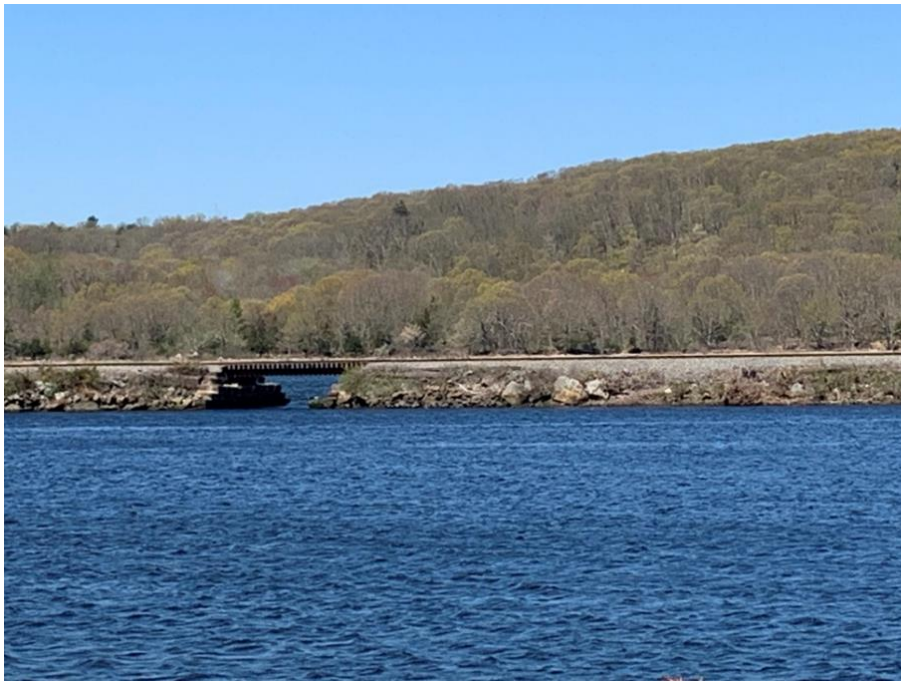
Figure 100: MP 3.80 - UG Bridge - Mill Cove - from Erickson Park (Looking Southwest)
