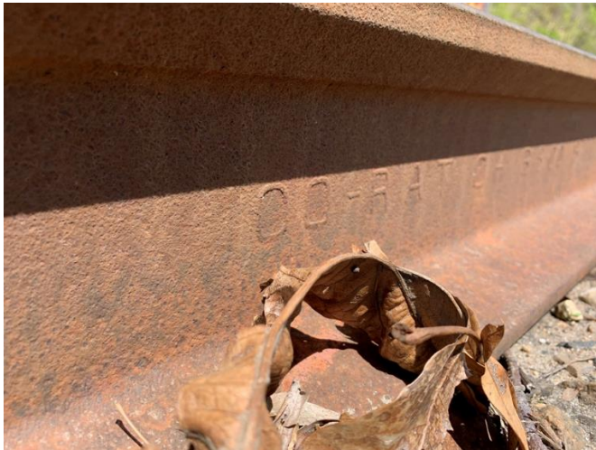
Figure 53: MP 5.76 – Track - 115RE lb/yd Running Rail
