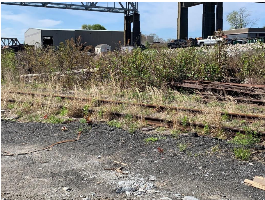
Figure 15: MP 0.65 – Track - Aetna Bridge Company Yard
