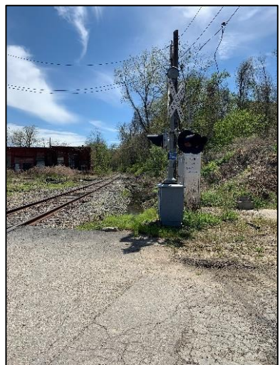
Figure 4: Ponding of Water Alongside Track Bed (MP 11.90)
