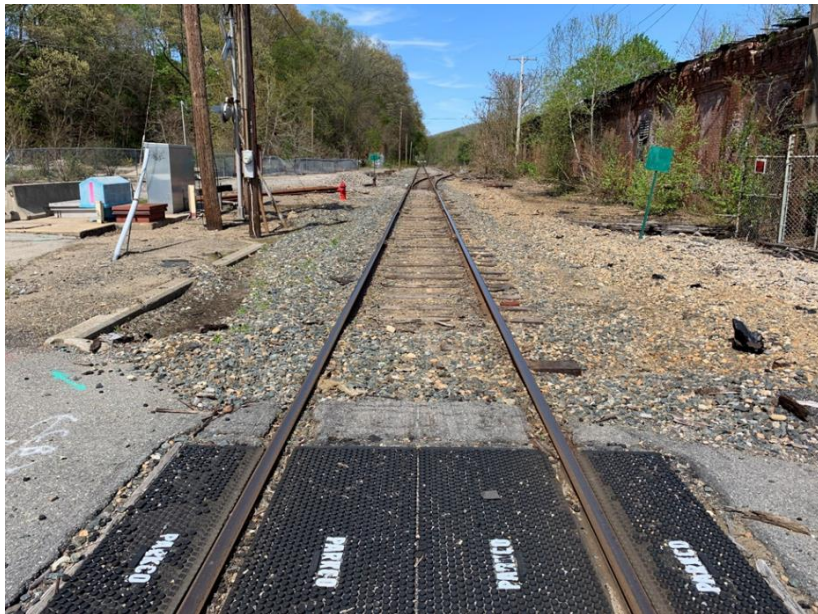
Figure 84: MP 12.12 – Track – Terminal Way – Manual Switch (Looking North)
