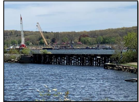
Figure 5: Timber Trestle Bridge
