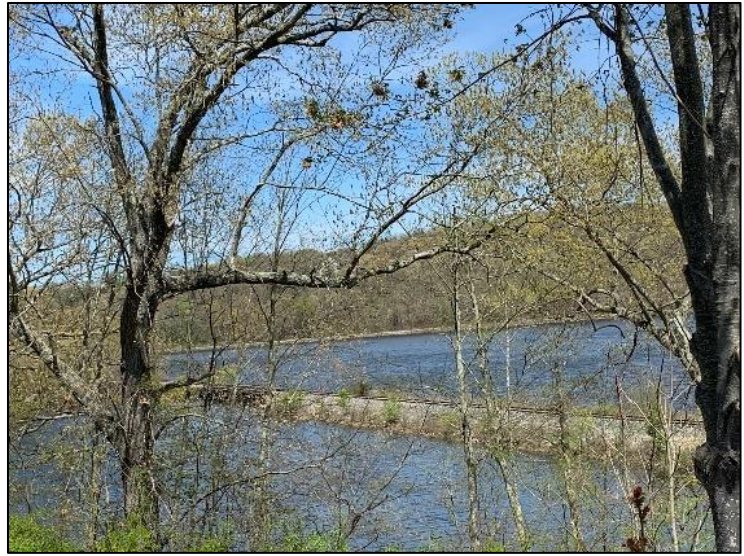
Figure 21: Thru-Girder Bridge at Trading Cove (MP 10.90)
