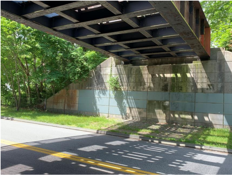
Figure 147: MP 1.35 - UG Bridge - Shennecossett Road
