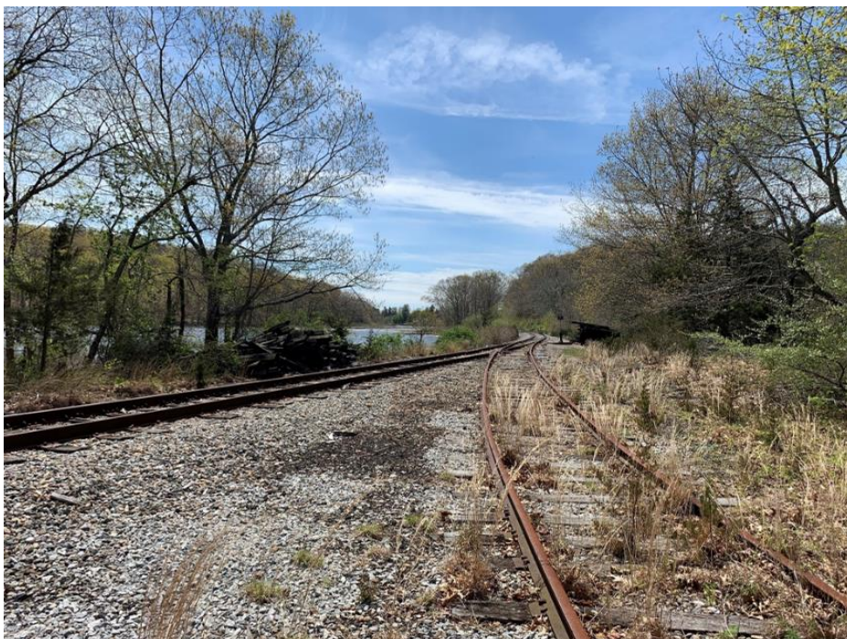
Figure 44: MP 3.00 – Track - Riverhead Building Supply – Looking South
