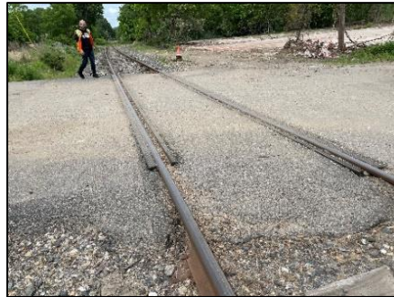
Figure 33: Good Condition - Terminal Way (MP 12.08)
