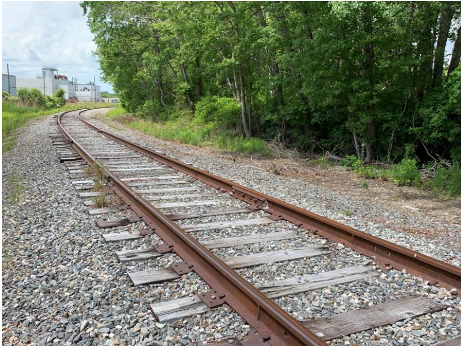
Figure 145: MP 1.18 - Track - Tower Avenue (Looking South)
