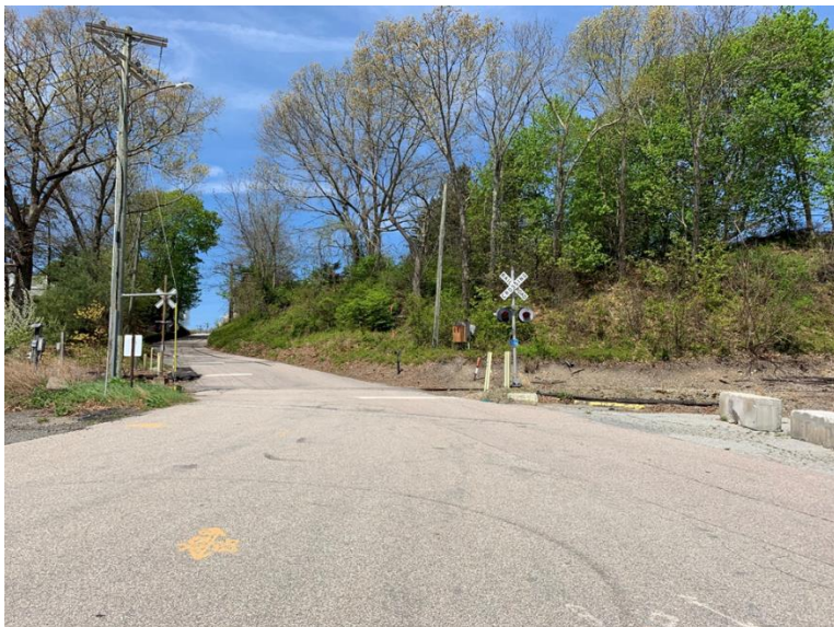
Figure 55: MP 5.76 - Grade Crossing - Dock Road (Looking West)
