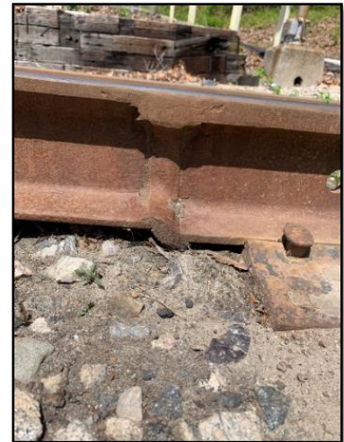
Figure 2: Weld between 100 and 115 lb. Steel Rail
