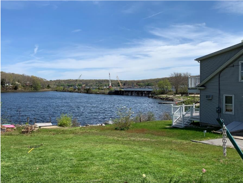
Figure 45: MP 3.25 – UG Bridge - Richards Grove Road - Timber Bridge - (Looking North)
