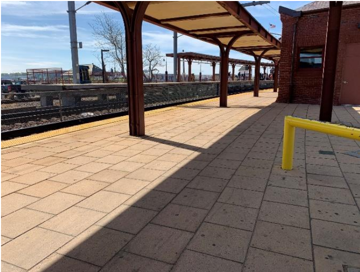
Figure 5: MP 122.90 – Platforms - New London Station (Looking Southeast from West Platform)
