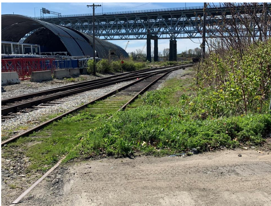
Figure 17: MP 0.91 - Grade Crossing - Eastern Avenue (Looking South)
