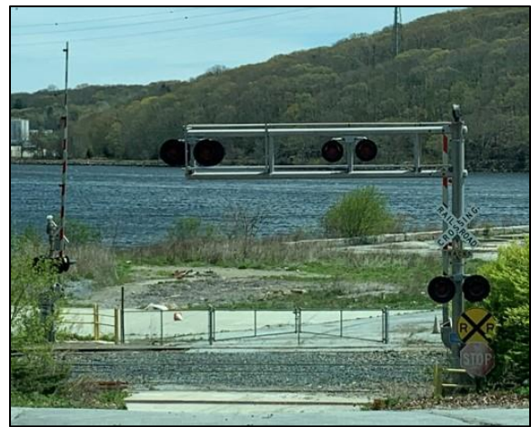
Figure 31: Depot Road Grade Crossing (MP 5.96)
