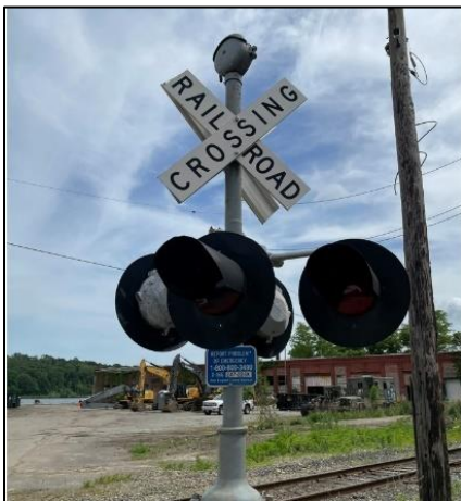
Figure 40: Terminal Way (MP 11.90)
