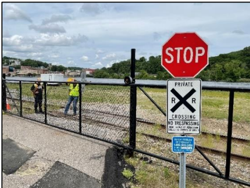
Figure 43: Fenced Grade Crossing - South Thames Street (MP 13.00)
