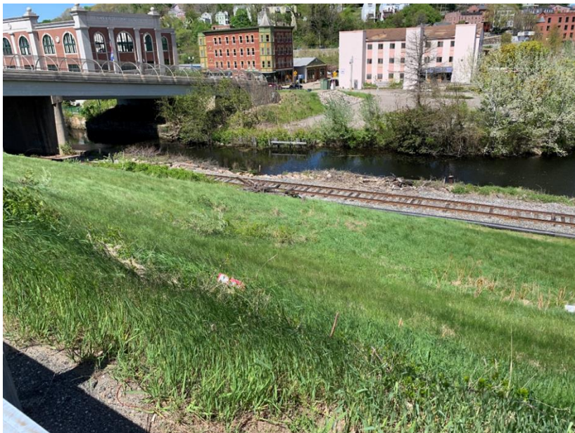
Figure 89: MP 13.14 – OH Bridge - West Main Street (Looking Northeast)
