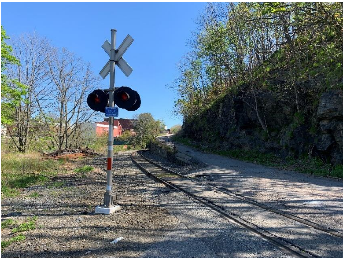
Figure 124: MP 11.99 - Grade Crossing - Shetucket Iron South (Looking North)
