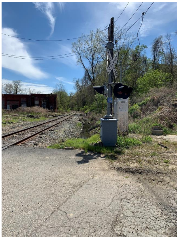
Figure 76: MP 11.90 – Grade Crossing - Terminal Way (Looking South)
