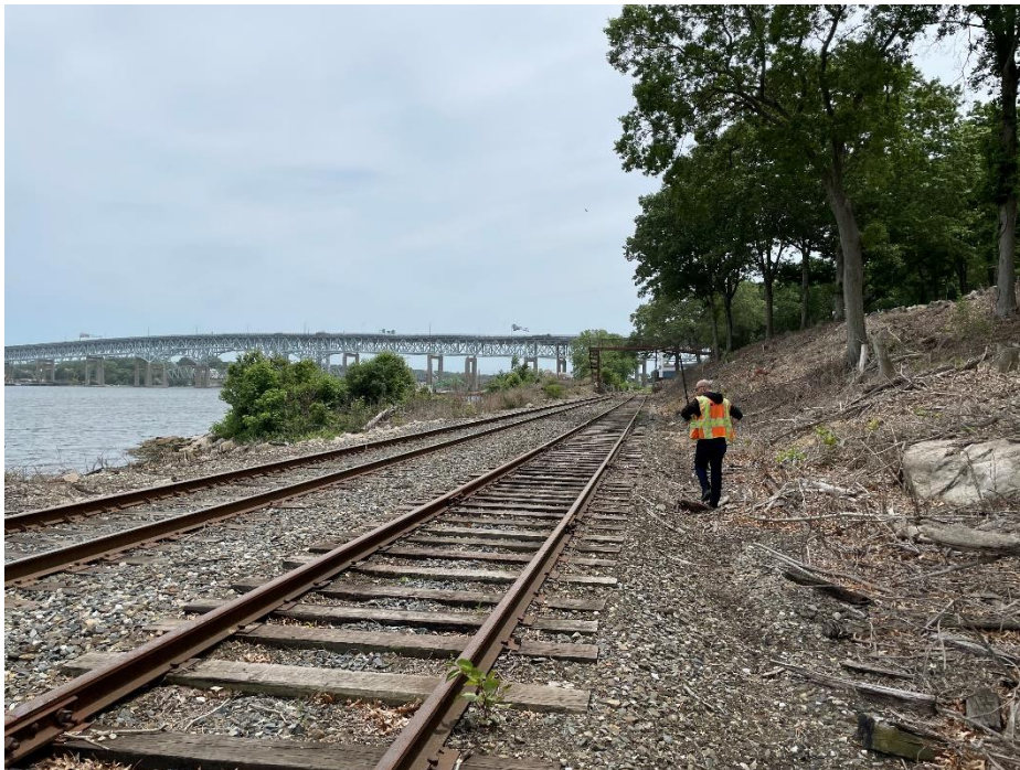
Figure 24: MP 1.07 – Track - Riverside Park - Right of Way
