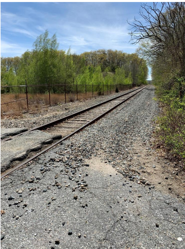
Figure 49: MP 5.05 - Grade Crossing - Lower Bartlett Road (Looking South)
