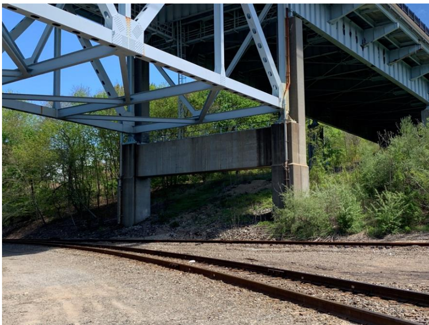
Figure 97: MP 0.82 – OH Bridge - Gold Star Memorial - I95 Southbound
