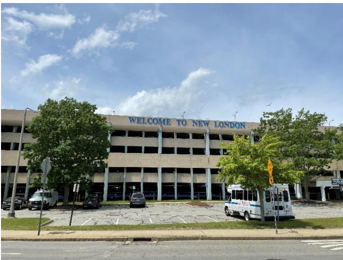
Figure 10: MP 122.90 - Parking Garage – Ferry Street - Designated Parking for New London Union Station
