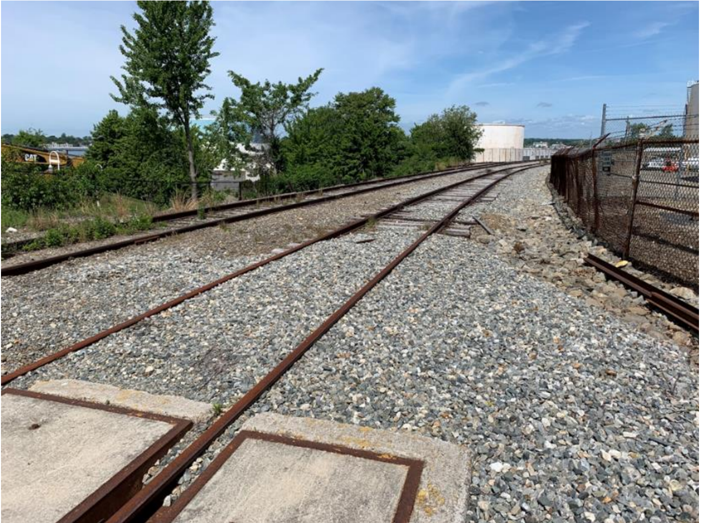
Figure 154: MP 2.85 - Track - General Dynamics (Looking West)
