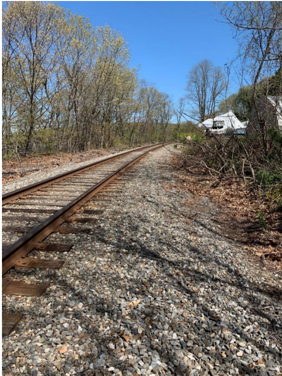
Figure 108: MP 5.11 - Track (Looking North)
