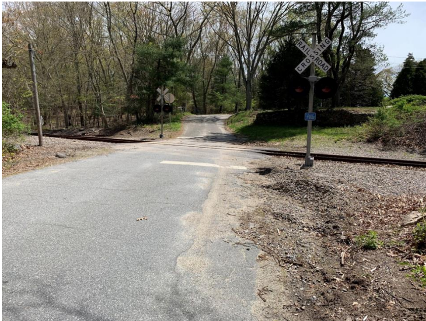
Figure 70: MP 7.87 – Grade Crossing - Derry Hill Road (Looking East)
