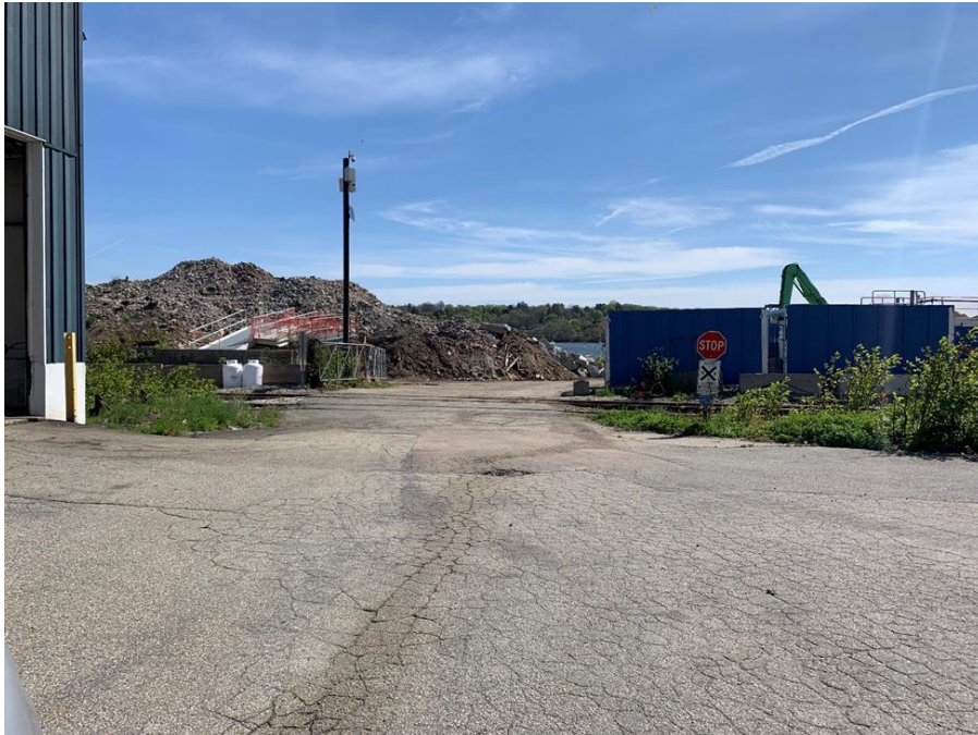
Figure 16: MP 0.91 – Grade Crossing - Approach near Eastern Ave - Looking East
