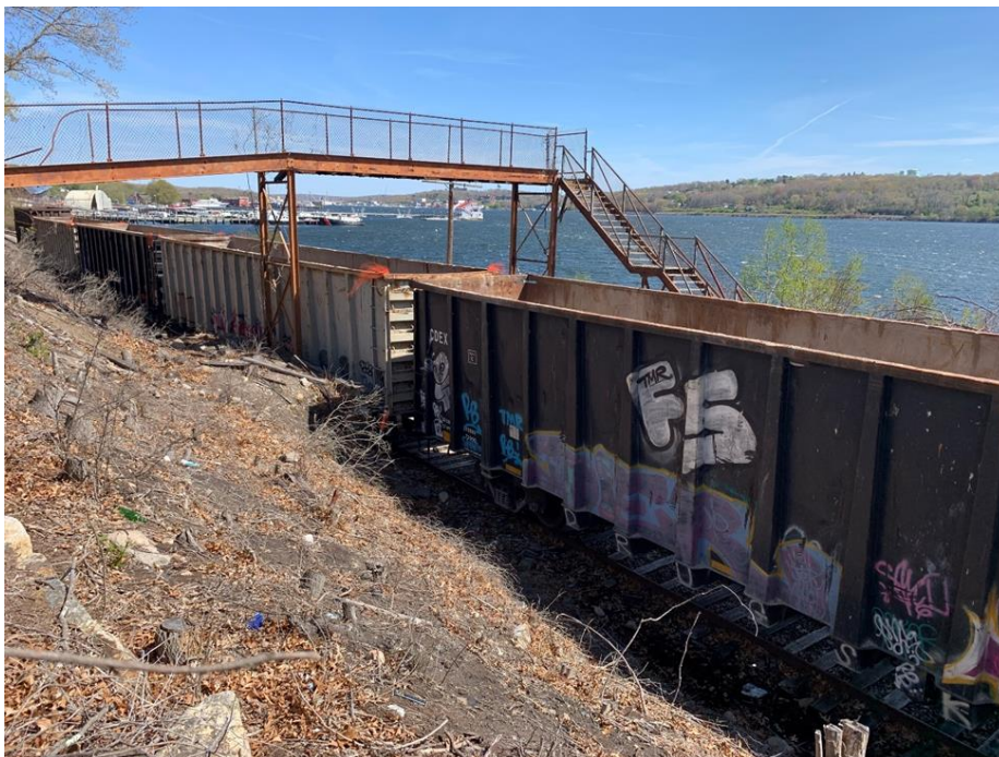
Figure 25: MP 1.07 - OH Bridge – Ped Bridge Riverside Park (Looking Northeast)
