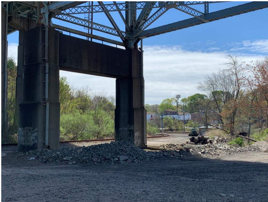
Figure 96: MP 0.82 – OH Bridge - Gold Star Memorial - I95 Northbound
