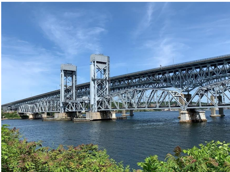
Figure 95: MP 123.90 – UG Bridge - Thames Moveable Bridge (Amtrak)
