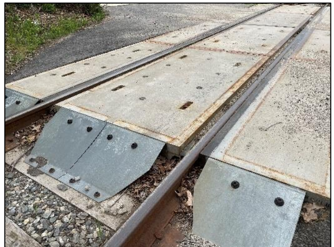
Figure 29: Point Breeze Grade Crossing (MP 6.50)
