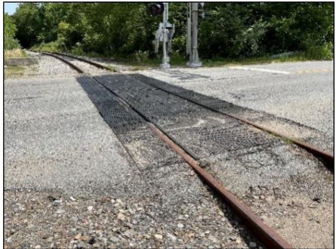
Figure 28: Benham Avenue Grade Crossing (MP 2.37)
