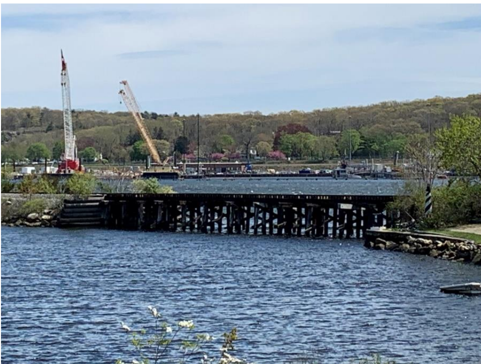
Figure 46: MP 3.25 – UG Bridge – Richards Grove Road - Timber Bridge - Zoomed In
