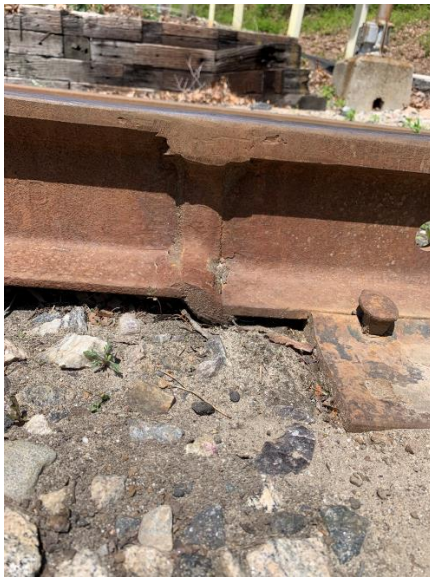
Figure 54: MP 5.76 - Track - Dock Road - CWR
