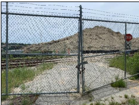
Figure 8: Thomas Griffin Road - Fenced Off Crossing with Private GC Sign
