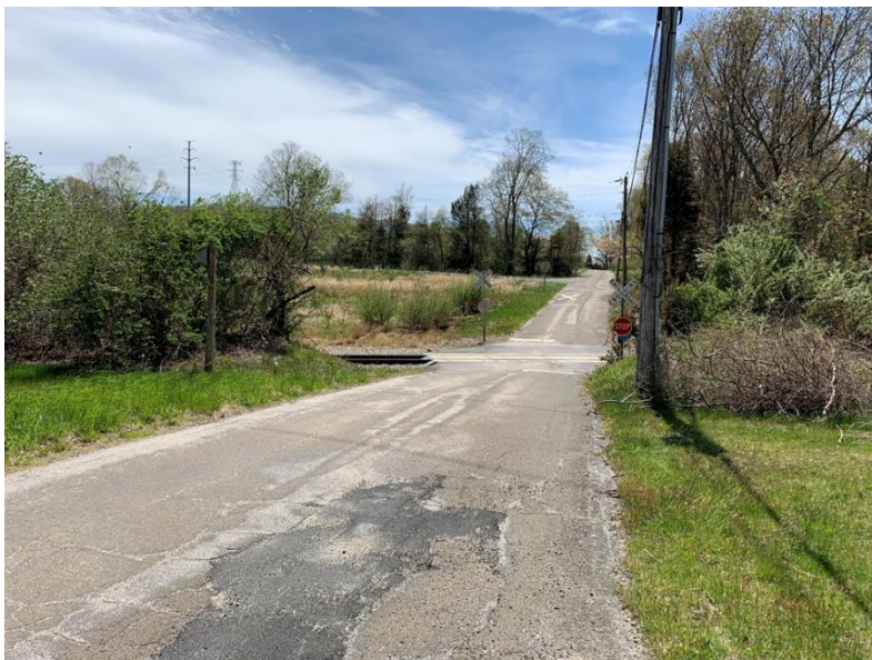
Figure 65: MP 6.50 - Grade Crossing - Point Breeze Road (Looking East)
