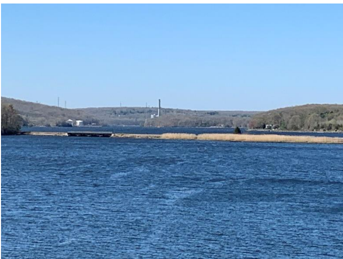
Figure 123: MP 7.83 - UG Bridge - Poquetanock Cove (No Access)
