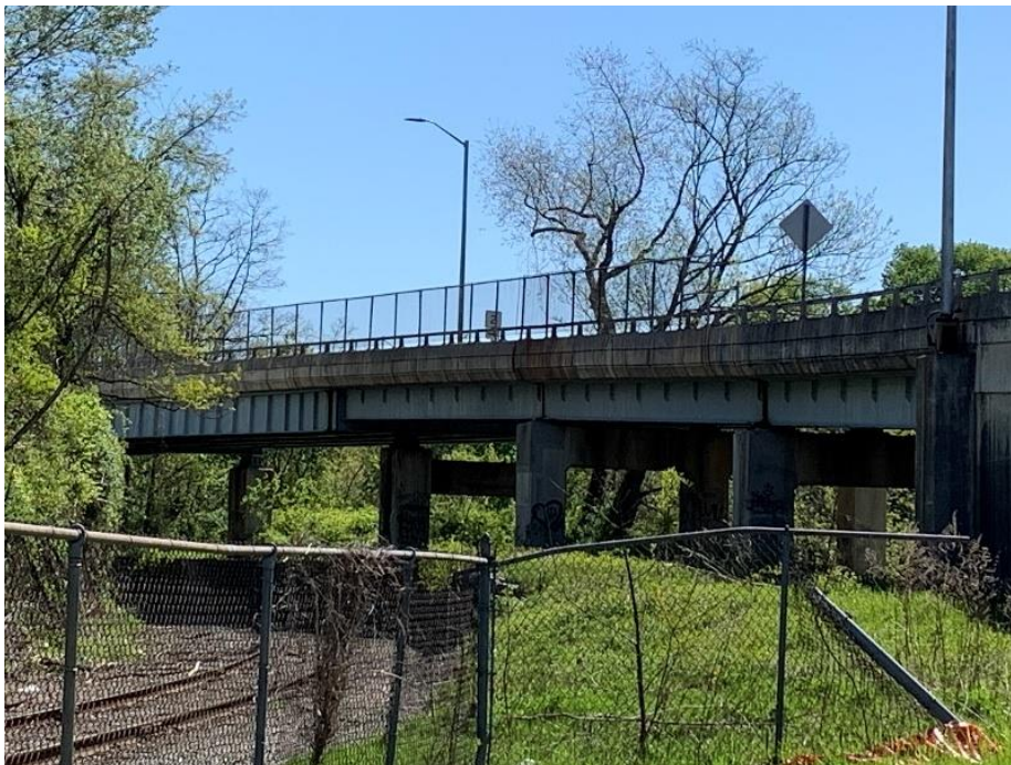
Figure 142: MP 12.36 - OH Bridge - Route 12 Viaduct (Looking East)
