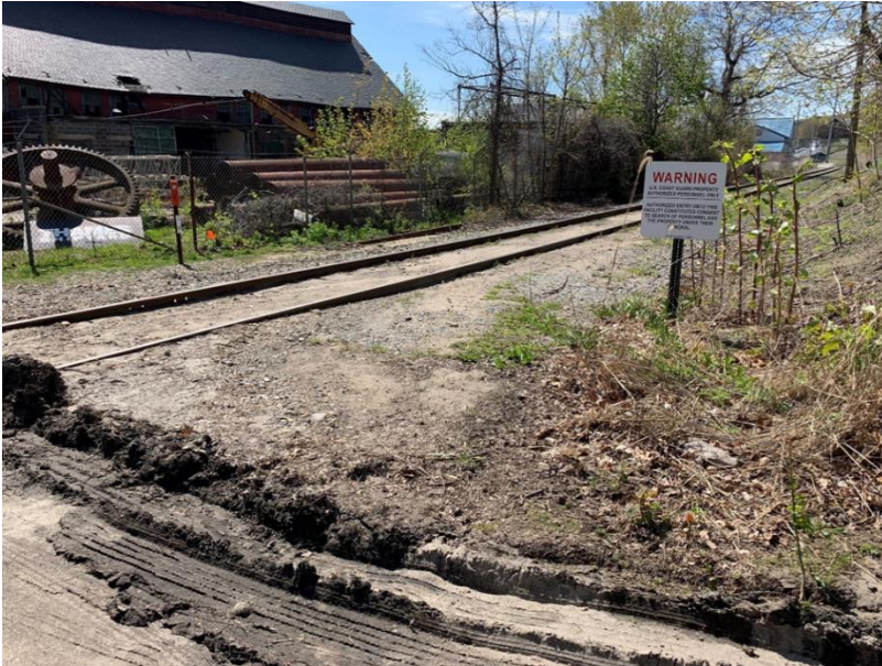
Figure 33: MP 1.79 - Grade Crossing - Farnsworth Street - Old Thames Shipyard (Looking South)
