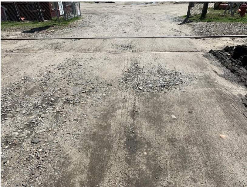
Figure 34: MP 1.79 - Grade Crossing - Farnsworth Street - Old Thames Shipyard (Looking East)
