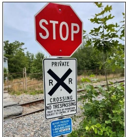
Figure 42: Unfenced Private Grade Crossing - Lower Bartlett Road (MP 5.05)
