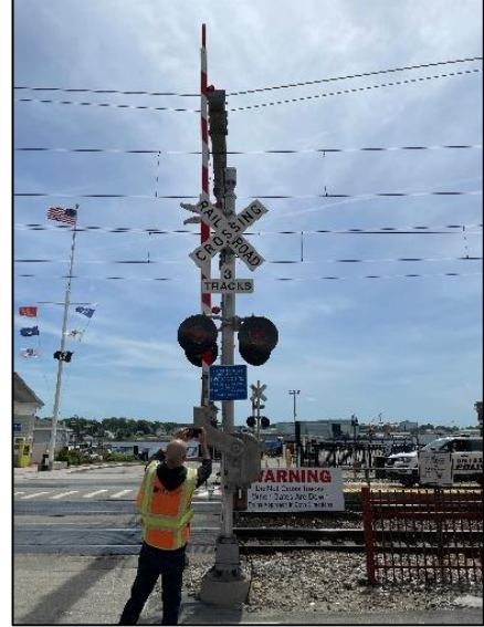
Figure 38: New London Train Station Grade Crossing (MP 122.76)
