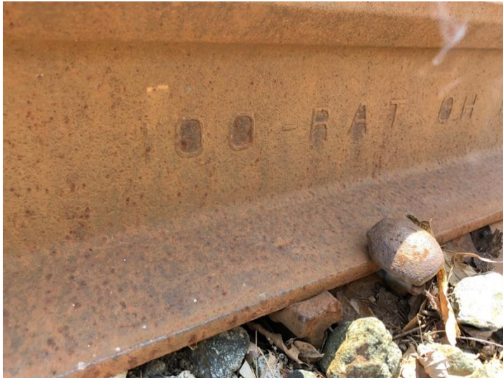
Figure 37: MP 2.37 – Track - Bentham Avenue
