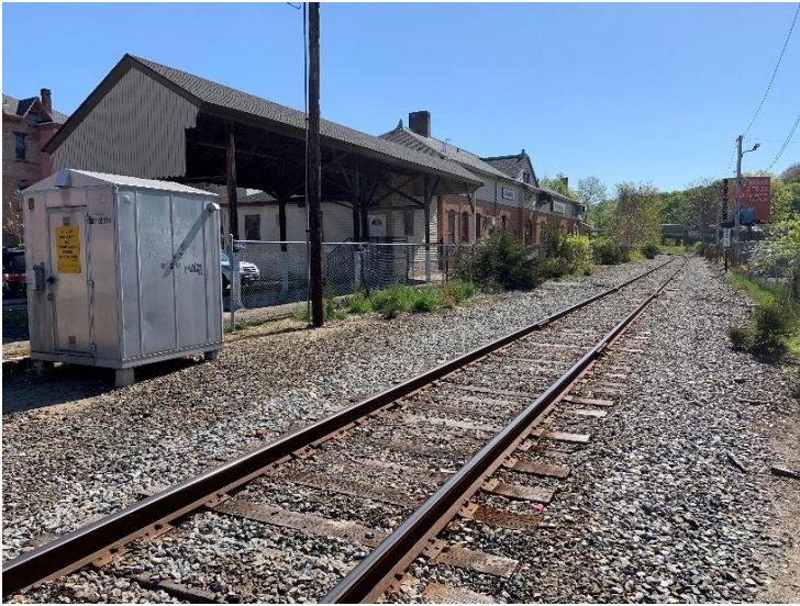
Figure 139: MP 12.16 - Grade Crossing - Norwich Station - Cabinet (Looking North)
