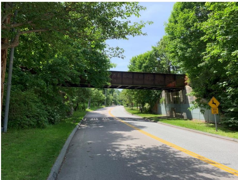
Figure 146: MP 1.35 - UG Bridge - Shennecossett Road (Looking North)
