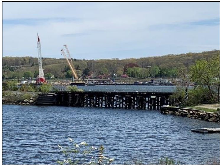
Figure 22: Timber Trestle (MP 3.18)
