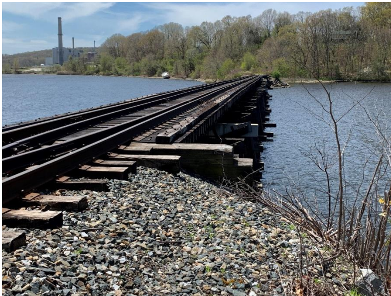
Figure 64: MP 6.23 - UG Bridge – Horton Cove - (I-Beam Pile Truss)
