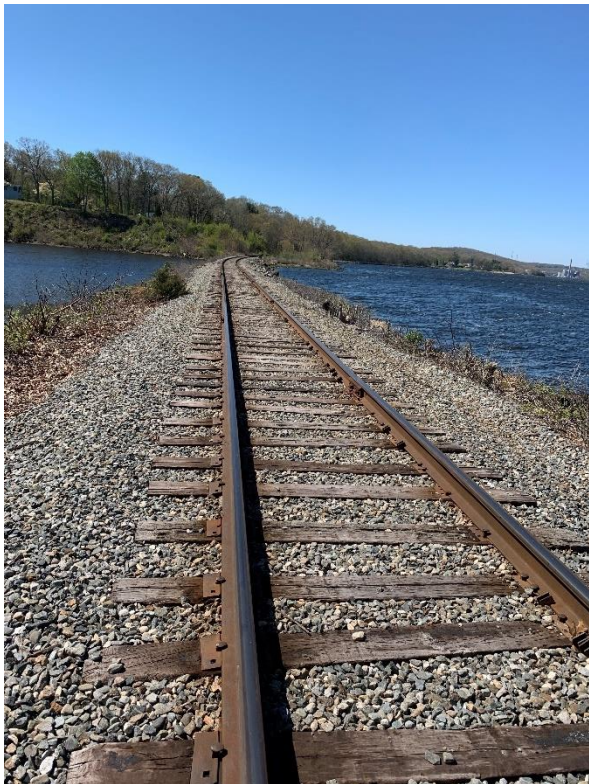
Figure 122: MP 7.09 - Track - Stoddard Cove (Looking South)
