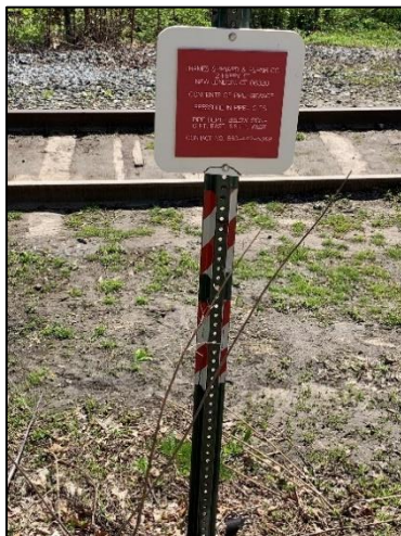
Figure 47: Signage for Buried Sewage Pipe (New London)
