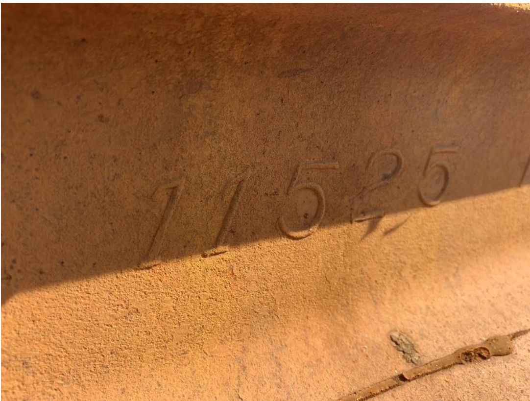
Figure 136: MP 12.14 - Track - Shetucket River/Norwich Station - (Looking East) - 115 Rail
