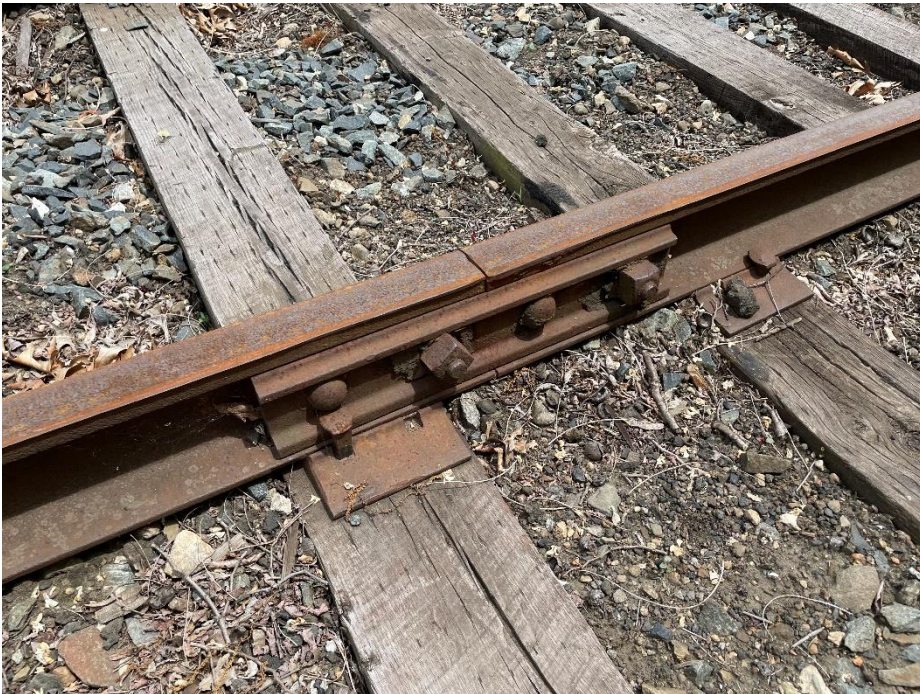
Figure 23: MP 1.07 – Track - Typical Rail Joint and Tie Condition
