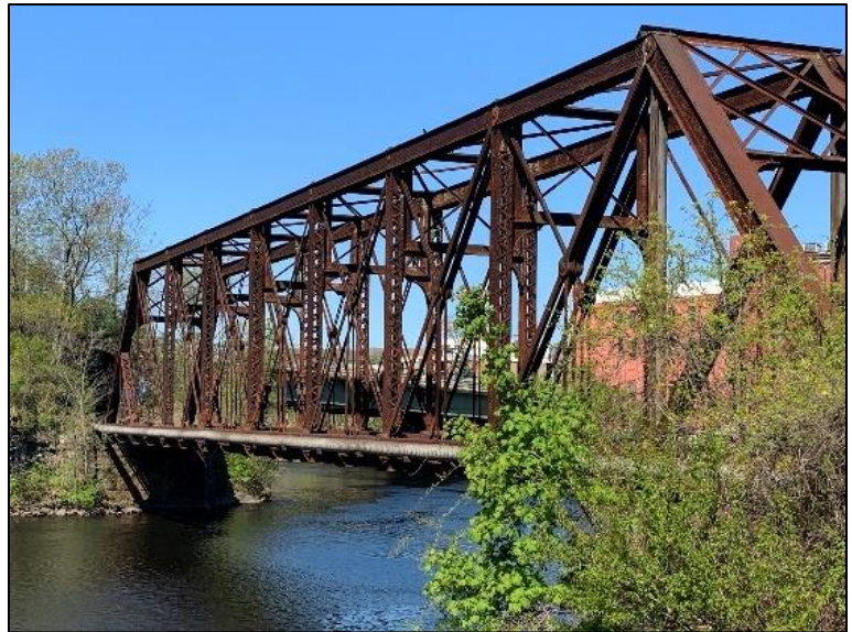
Figure 20: Steel Truss Bridge at MP 12.14
