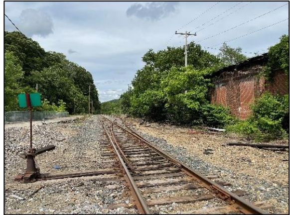
Figure 14: Manual Track Switches and Interlockings
