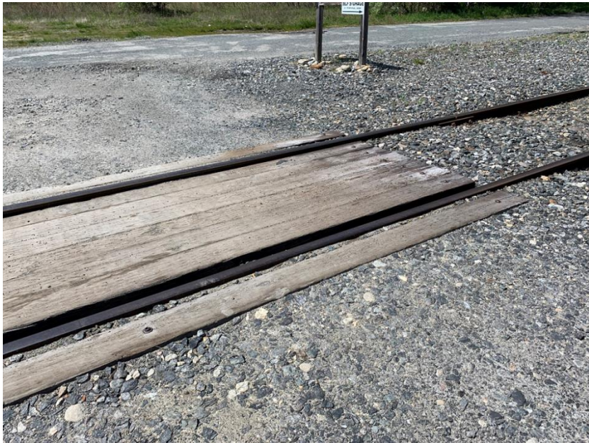
Figure 80: MP 12.08 – Grade Crossing - Terminal Way - (Looking Northwest)
