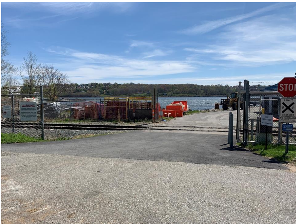
Figure 28: MP 1.70 - Grade Crossing - North of USCGA Rowing Center (Looking East)
