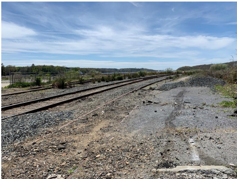
Figure 61: MP 5.96 – Grade Crossing - Depot Road - (Looking South)
