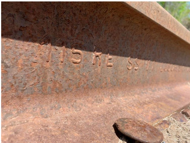
Figure 53: MP 5.76 – Track - 115RE lb/yd Running Rail
