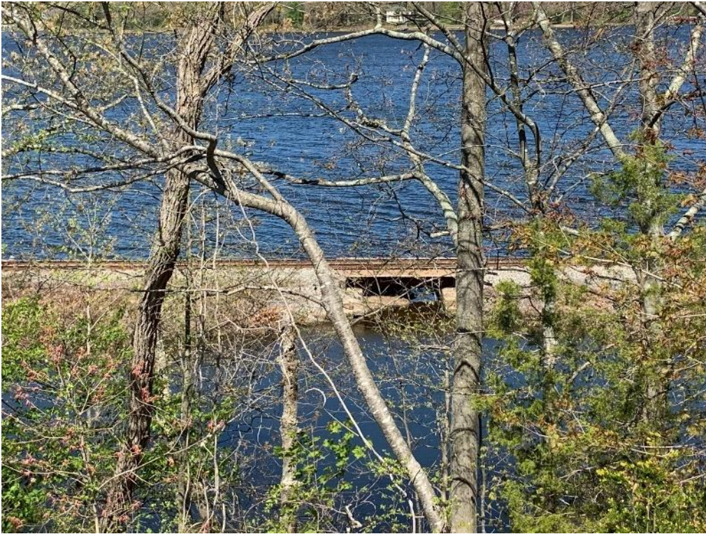
Figure 116: MP 6.79 - UG Bridge - Stoddards Warf Road
