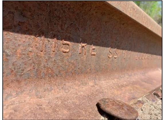
Figure 11: 115 RE Steel Rail
