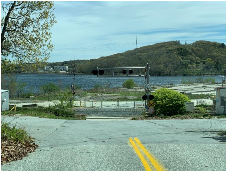
Figure 60: MP 5.96 – Grade Crossing - Depot Road - Approach (Looking East)
