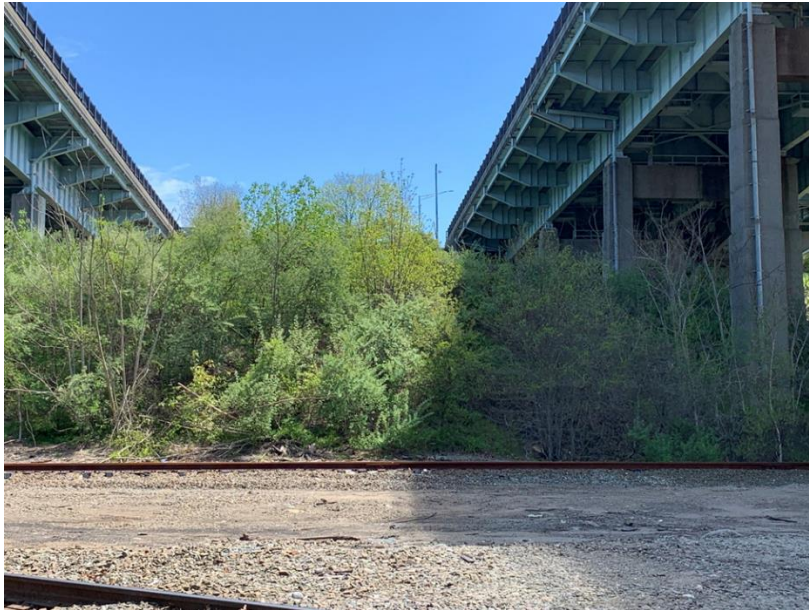
Figure 98: MP 0.82 – Track - Under I-95 Bridge (Looking East)
