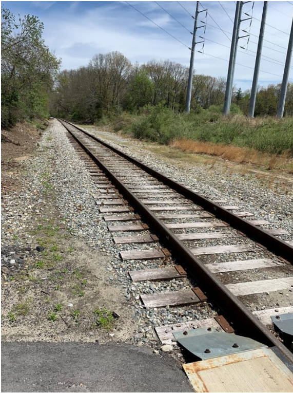
Figure 68: MP 6.50 - Grade Crossing - Point Breeze Road (Looking North)
