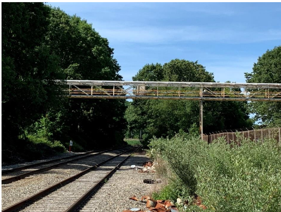
Figure 113: MP 6.08 - OH Structure - Unidentified (Looking South)
