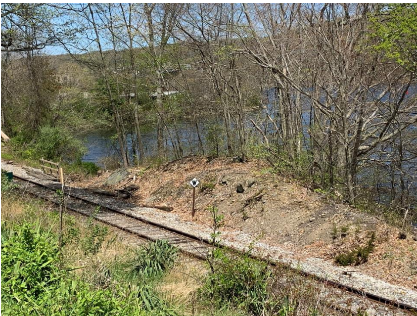
Figure 75: MP 11.72 - UG Bridge - Timber Trestle - from Coolidge Street (Looking North)
