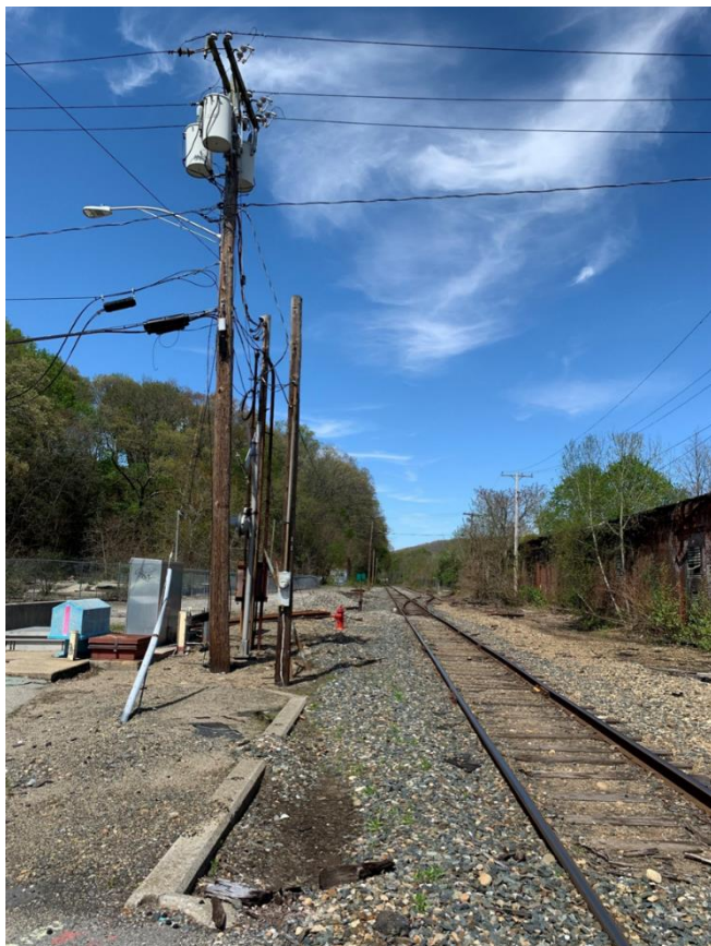
Figure 85: MP 12.12 – Track – Terminal Way - (Looking North)
