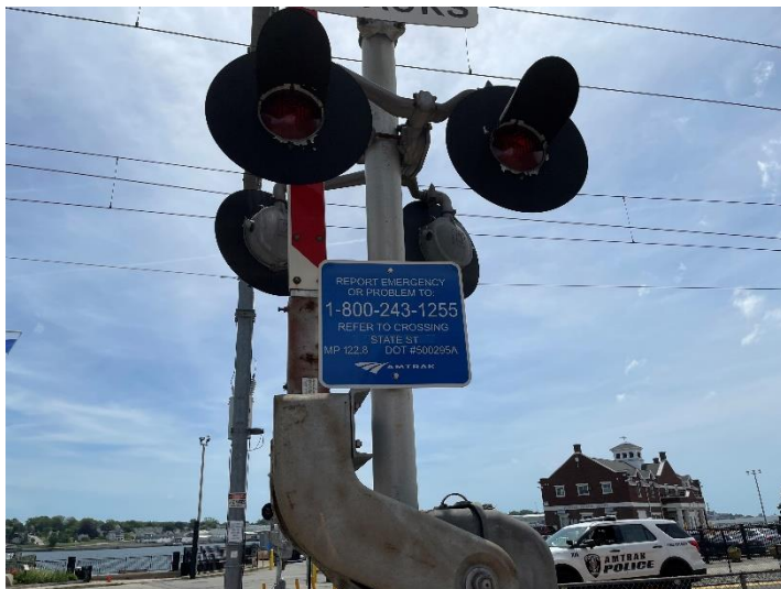
Figure 3: MP 122.76 - Grade Crossing – State Street – GC Protection System with Gates, Flashers, and Bells
