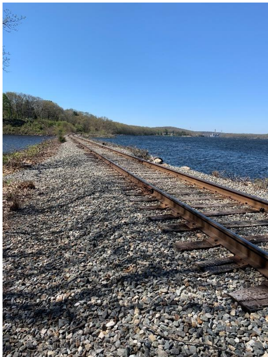
Figure 120: MP 7.09 - UG Bridge - Stoddard Cove (Looking South)
