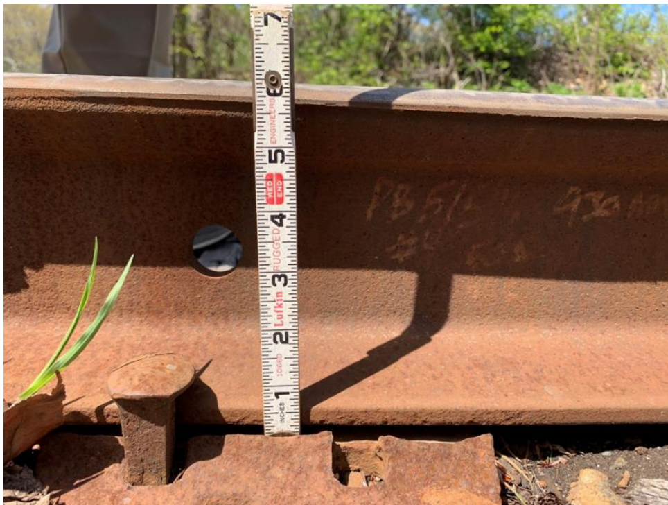
Figure 39: MP 2.37 - Track - Bentham Avenue – Measure of Vertical Height
