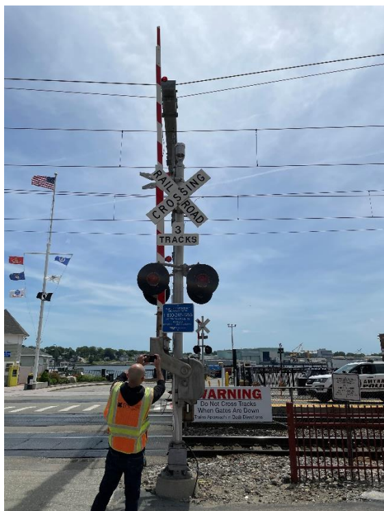
Figure 3: MP 122.76 - Grade Crossing – State Street – GC Protection System with Gates, Flashers, and Bells
