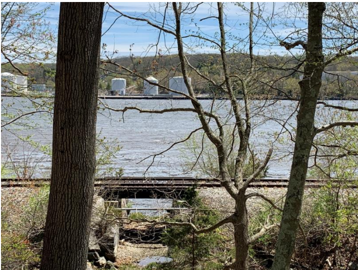
Figure 69: MP 6.81 - UG Bridge (I-Beam)
