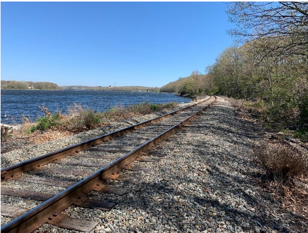
Figure 117: MP 6.79 - Track - Stoddards Warf Road (Looking North)
