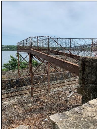
Figure 23: Riverside Park (MP 1.07)
