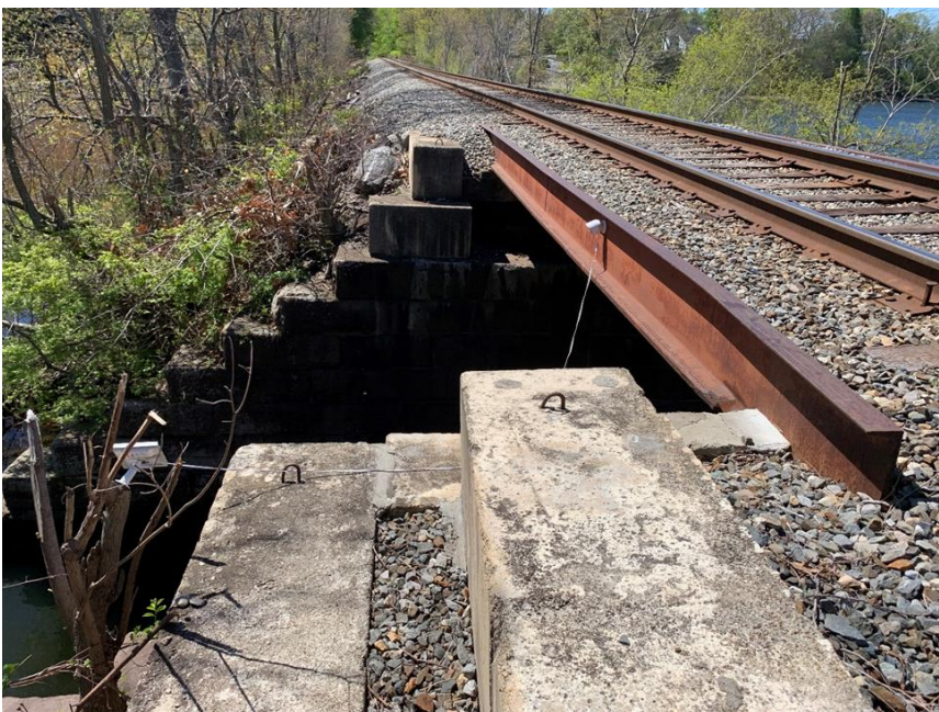
Figure 103: MP 5.11 - UG Bridge - Clark's Cove (Looking South, East of Bridge)
