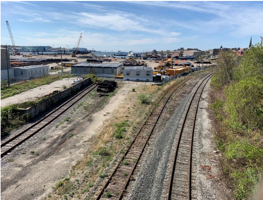
Figure 13: MP 0.62 – OH Bridge - State Pier Road (Looking South)
