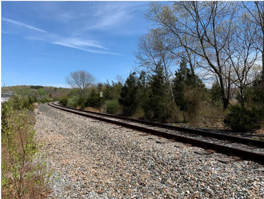
Figure 43: MP 3.00 – Track - Riverhead Building Supply - Looking North
