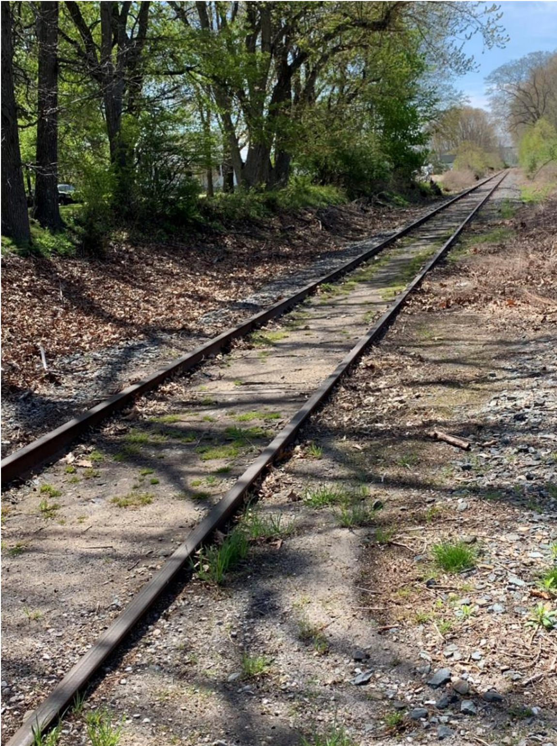
Figure 41: MP 2.37 - Grade Crossing - Bentham Avenue (Looking South)
