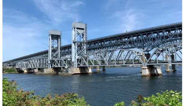
Figure 4. Groton Moveable Bridge
