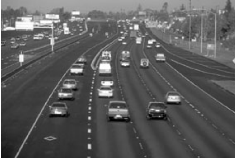
Figure 2-4. Example ML Entrance from GP Lanes I-15, Orange County, CA Source: A Guide for HOT Lane Development , FHWA, March 2003
