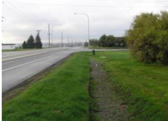
Image from the Washington DOT Highway Runoff Manual, Engineered Dispersion, Pg. 5-140. Dated April 2014 with supplement February 2016. https://www.wsdot.wa.gov/publications/manuals/fulltext/M31-16/highwayrunoff.pdf
