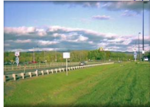
Image from the MA Stormwater Handbook, Volume 2, Chapter 2, Water Quality Swale, Pg. 77
