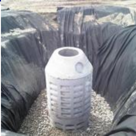
Image from the Washington DOT Highway Runoff Manual. Dry Well, Pg. 5-156. Dated April 2014 with supplement February 2016. https://www.wsdot.wa.gov/publications/manuals/fulltext/M31-16/highwayrunoff.pdf
