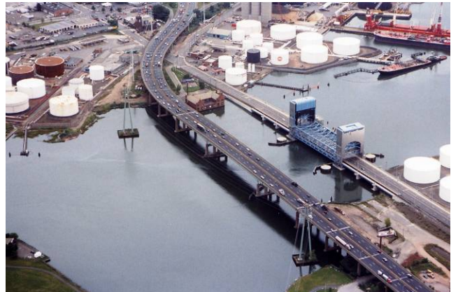
Figure II-3. “Q” Bridge - I-95 in New Haven
