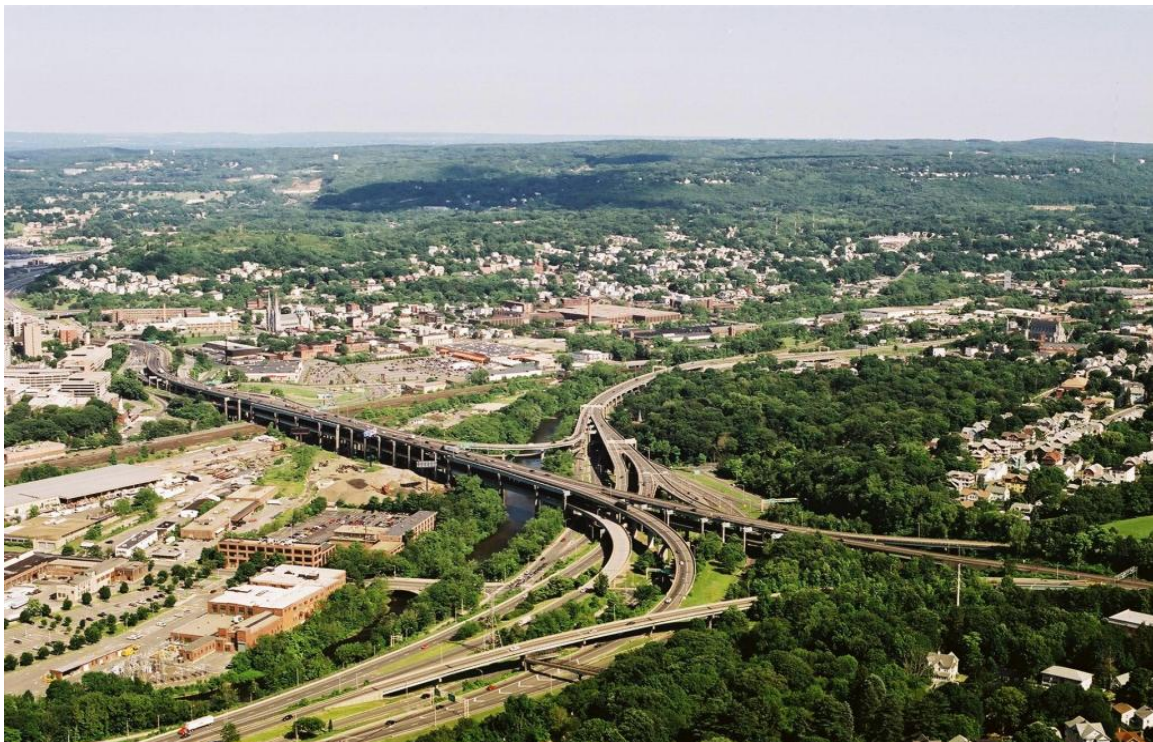
Figure II-7. I-84 / Route 8 Interchange in Waterbury
