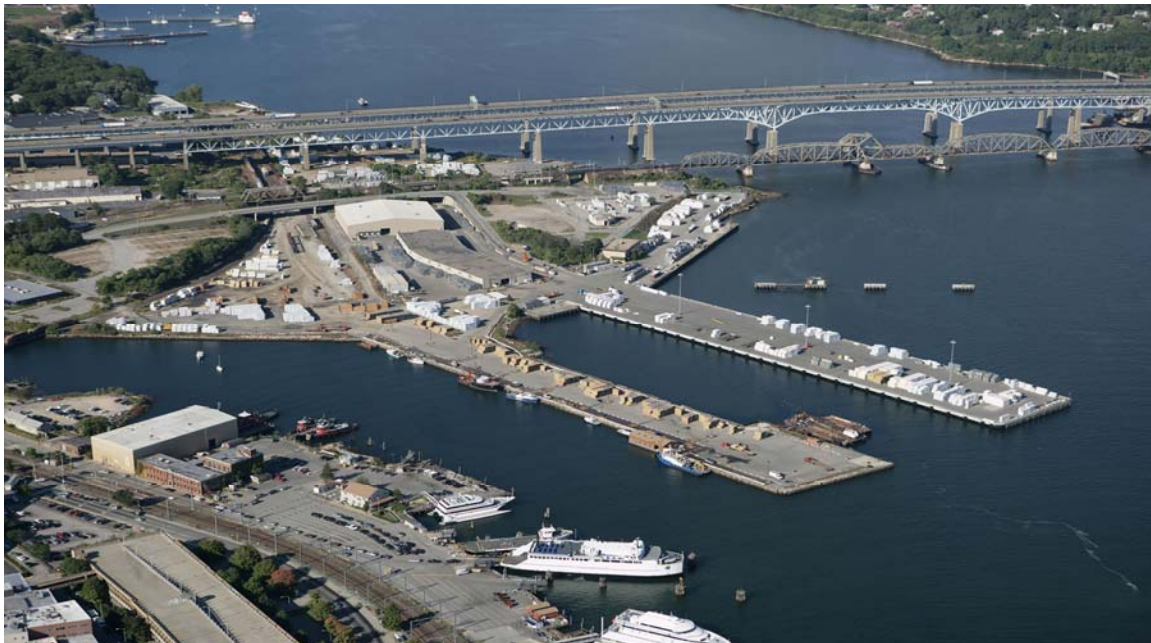
Figure II-12. Aerial View of State Pier Complex in New London, CT
