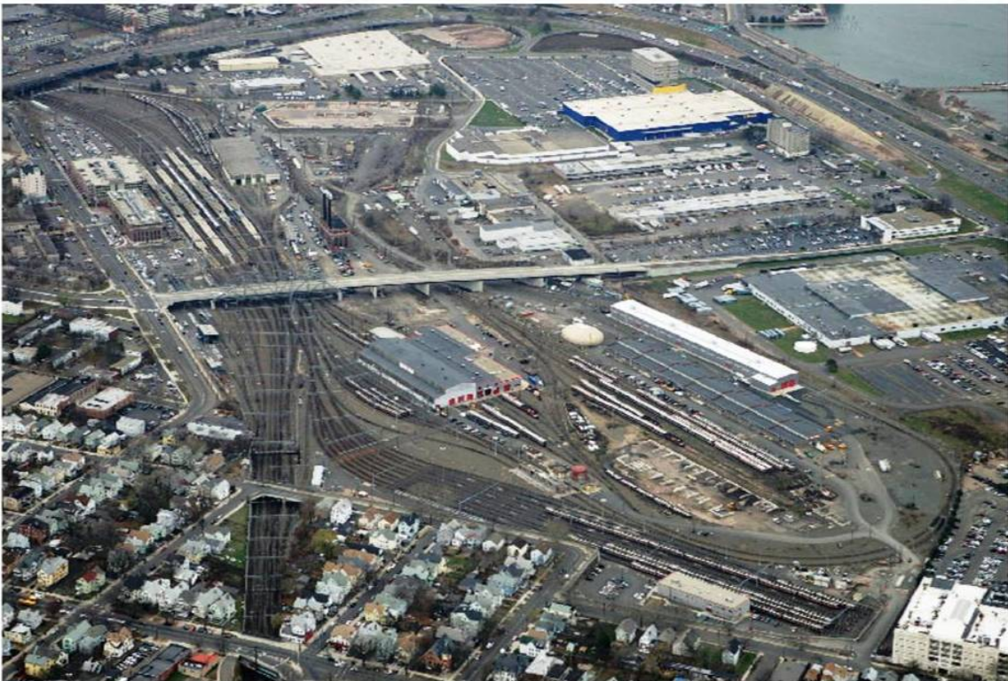
Figure II-7 Aerial Photo of New Haven Rail Yard
