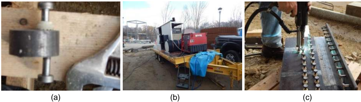
Figure 2.14 Installation of Studs for the UHSC Repair
