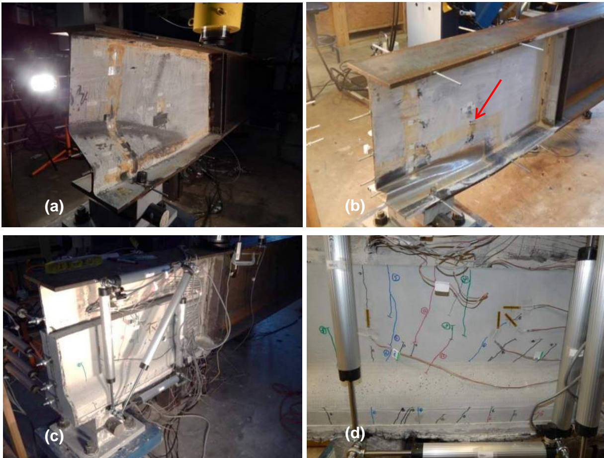
Figure 13. Appearance of the Failed Girders (a) Undamaged, (b) Damaged, (c) Repaired, (d) UHPC Cracking
