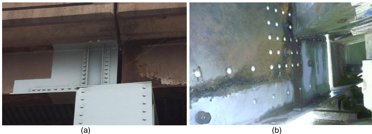
Figure 1.3 Traditional Rehabilitation with Steel Shapes
