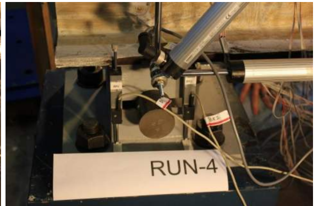
Figure B.2.37 Damaged Girder Bearing: 32 kip
