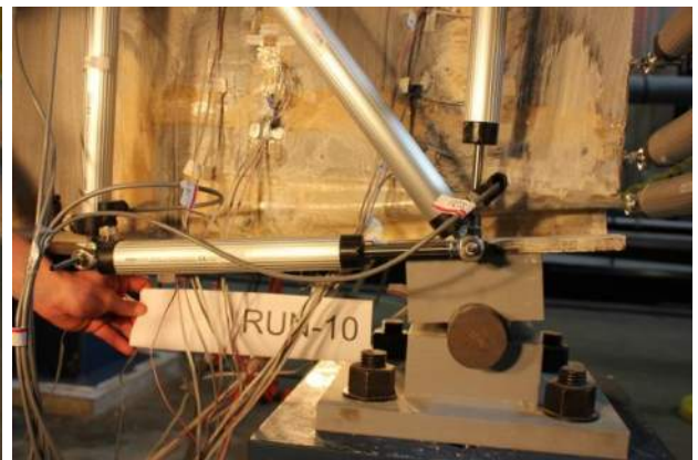
Figure B.2.43 Damaged Girder Bearing: +1.00 in
