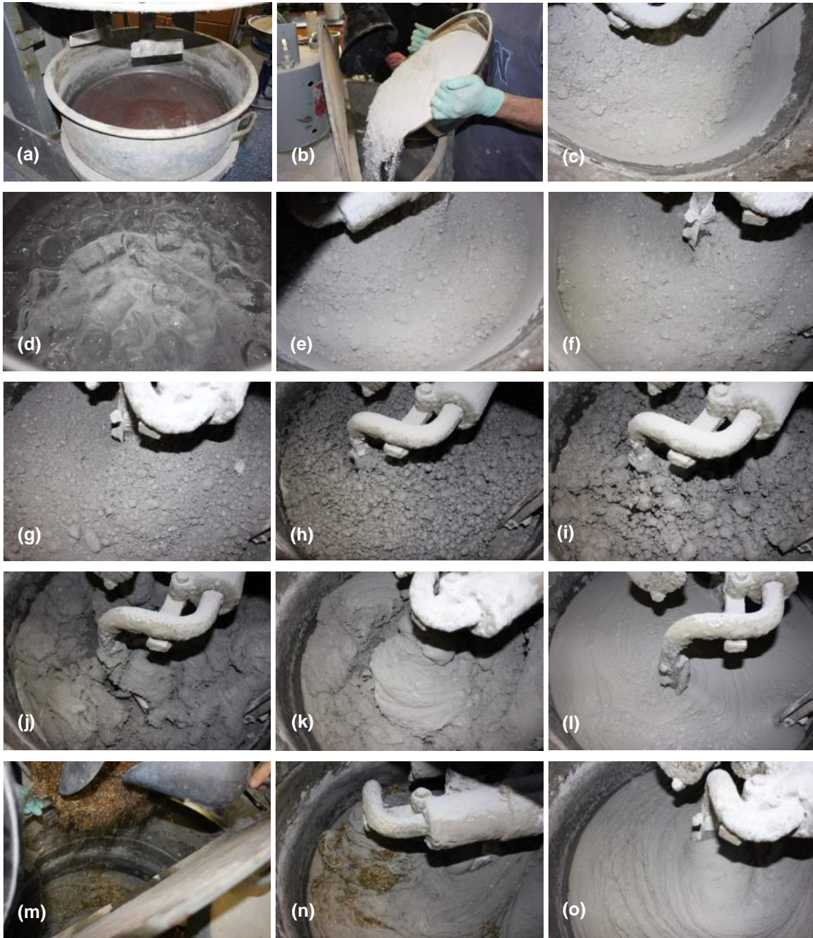
Figure 2.17 Mixing the UHPC
