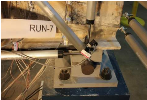
Figure B.2.40 Damaged Girder Bearing: +0.25 in
