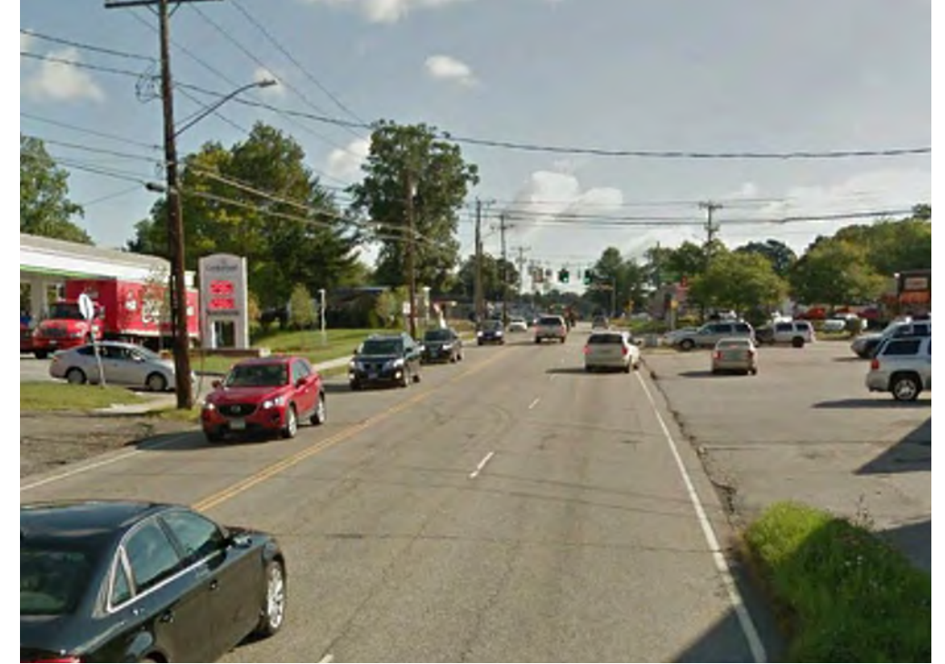
Excessively Wide Curb Cuts Compromise Safe Vehicular and Pedestrian Movement
