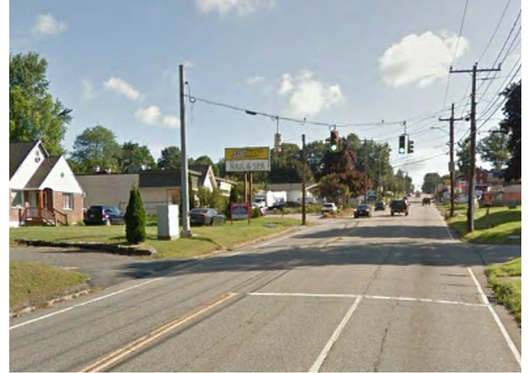
Safe Pedestrian Facilities Lacking Throughout Corridor
