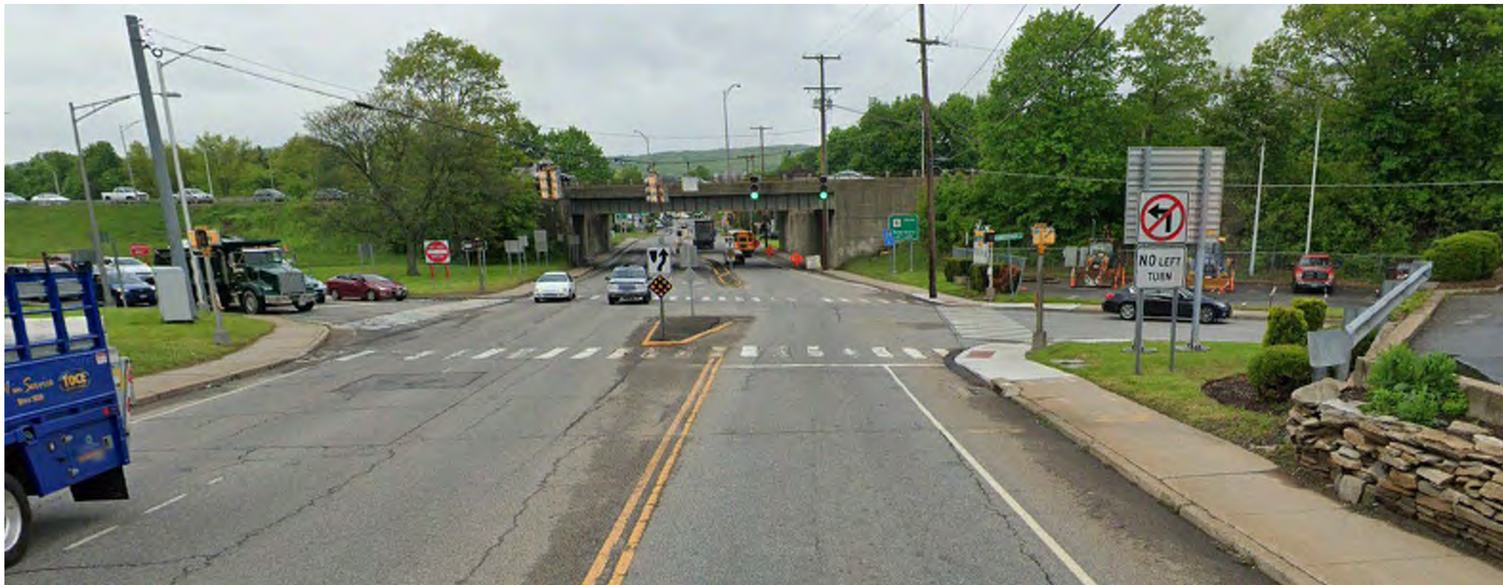
Existing View at Route 8 Gateway
