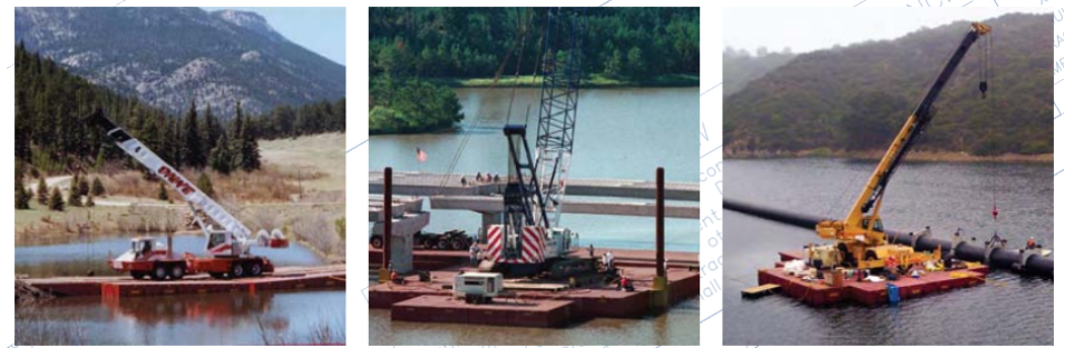
Rehabilitation of Bridge No. 00571A // State Project No. 126-176
