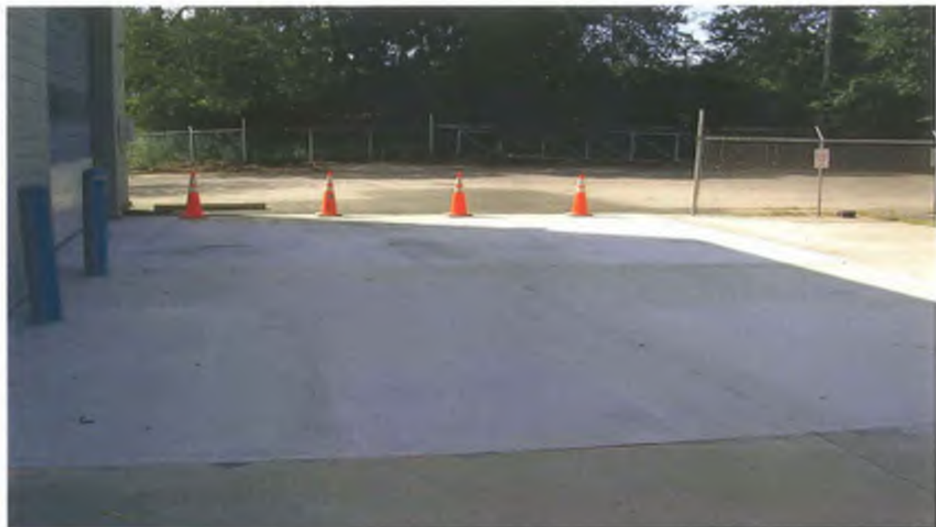
Photo 21: Completed concrete pad over former UST #1 and #2 location.
