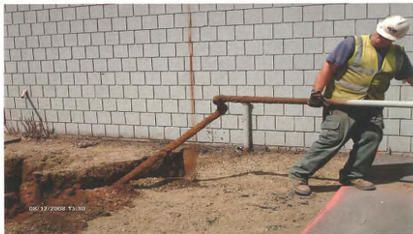
Photo 8: Removal of UST #3 vent pipe.
