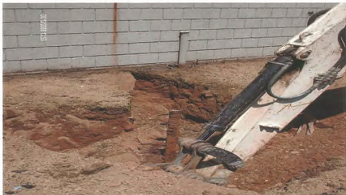
Photo 9: Excavation of UST #3.
