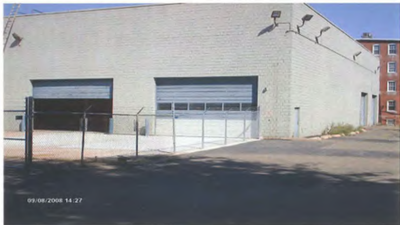
Photo 24: Reestablished security fence through former fuel dispenser island area.
