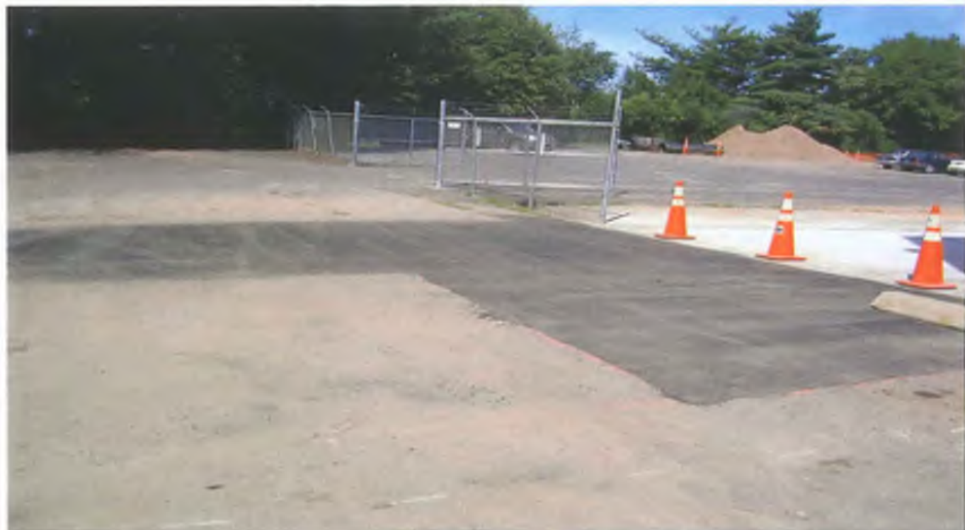
Photo 23: Former dispenser island area backfilled, compacted, and completed with bituminous concrete.
