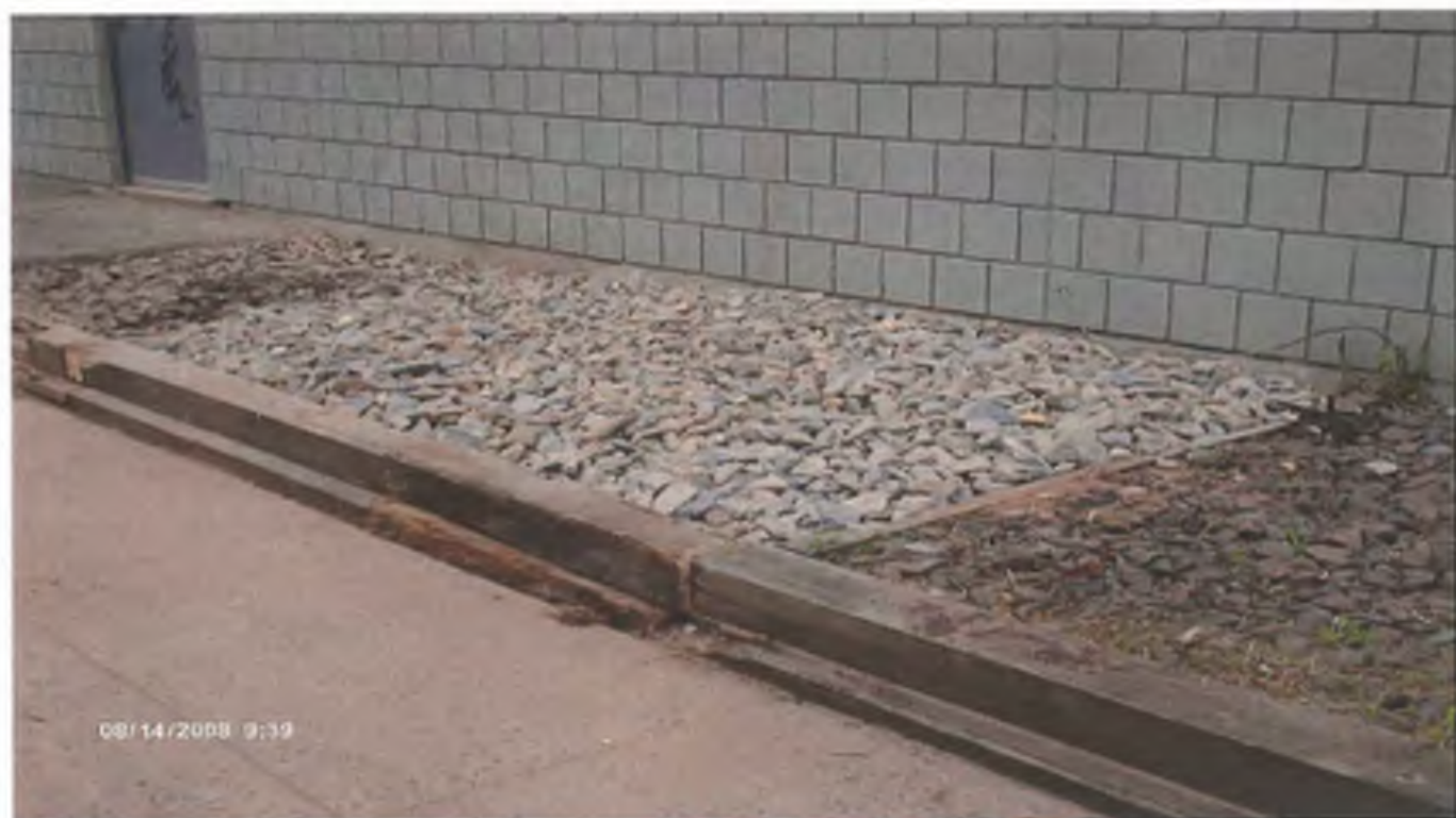
Photo 7: UST #4, backfilled with final restoration complete.
