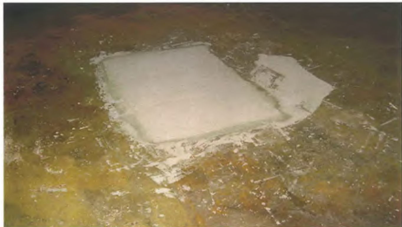
Photo 22: Sealed interior floor drain to UST #4.
