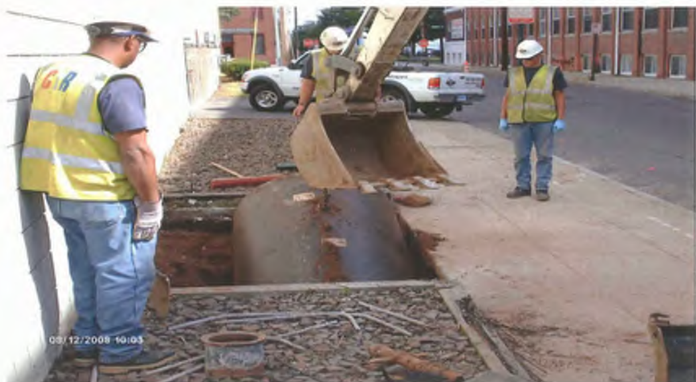
Photo 5: Removal of UST #4.
