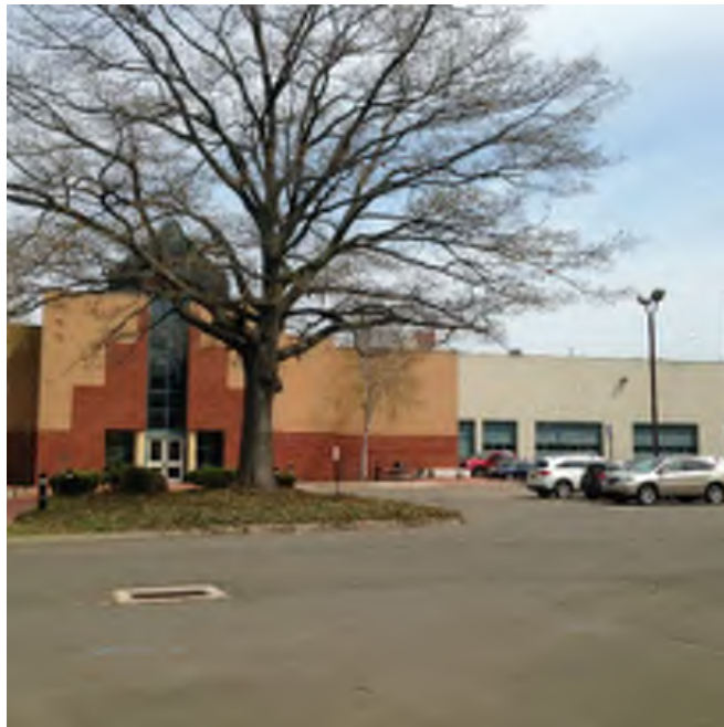
Photo 4 – Building Entrance and Parking Area
