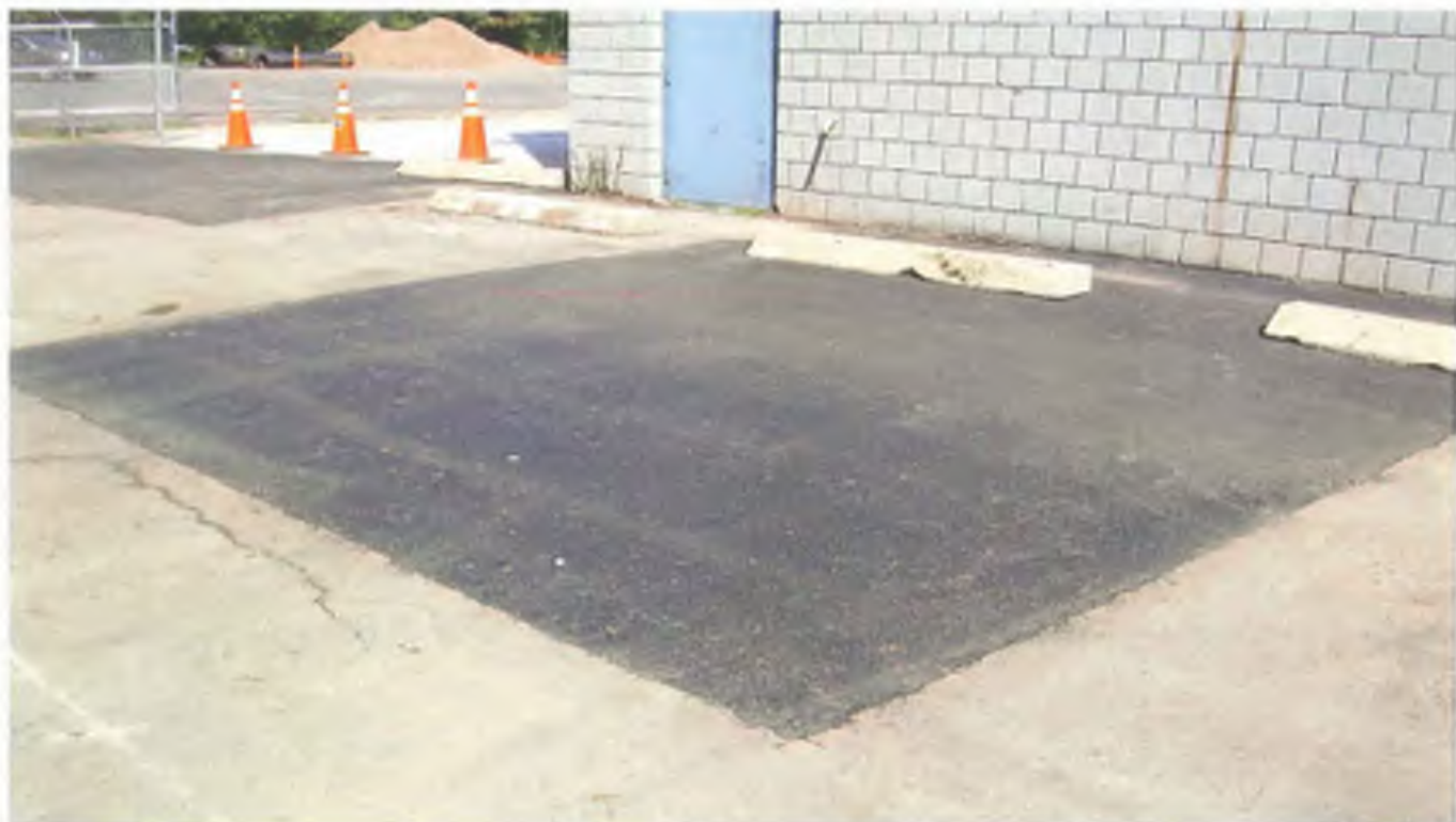
Photo 12: UST #3 excavation completed with bituminous concrete.
