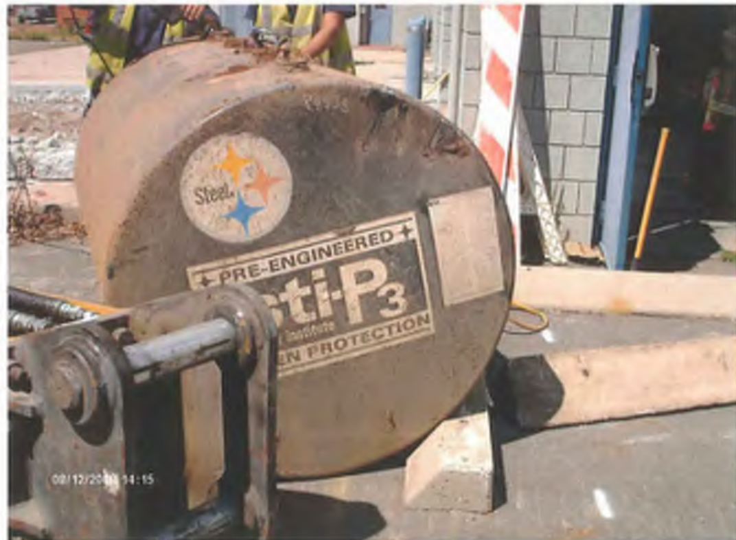
Photo 10: UST #3 removed and staged for decontamination and disposal.
