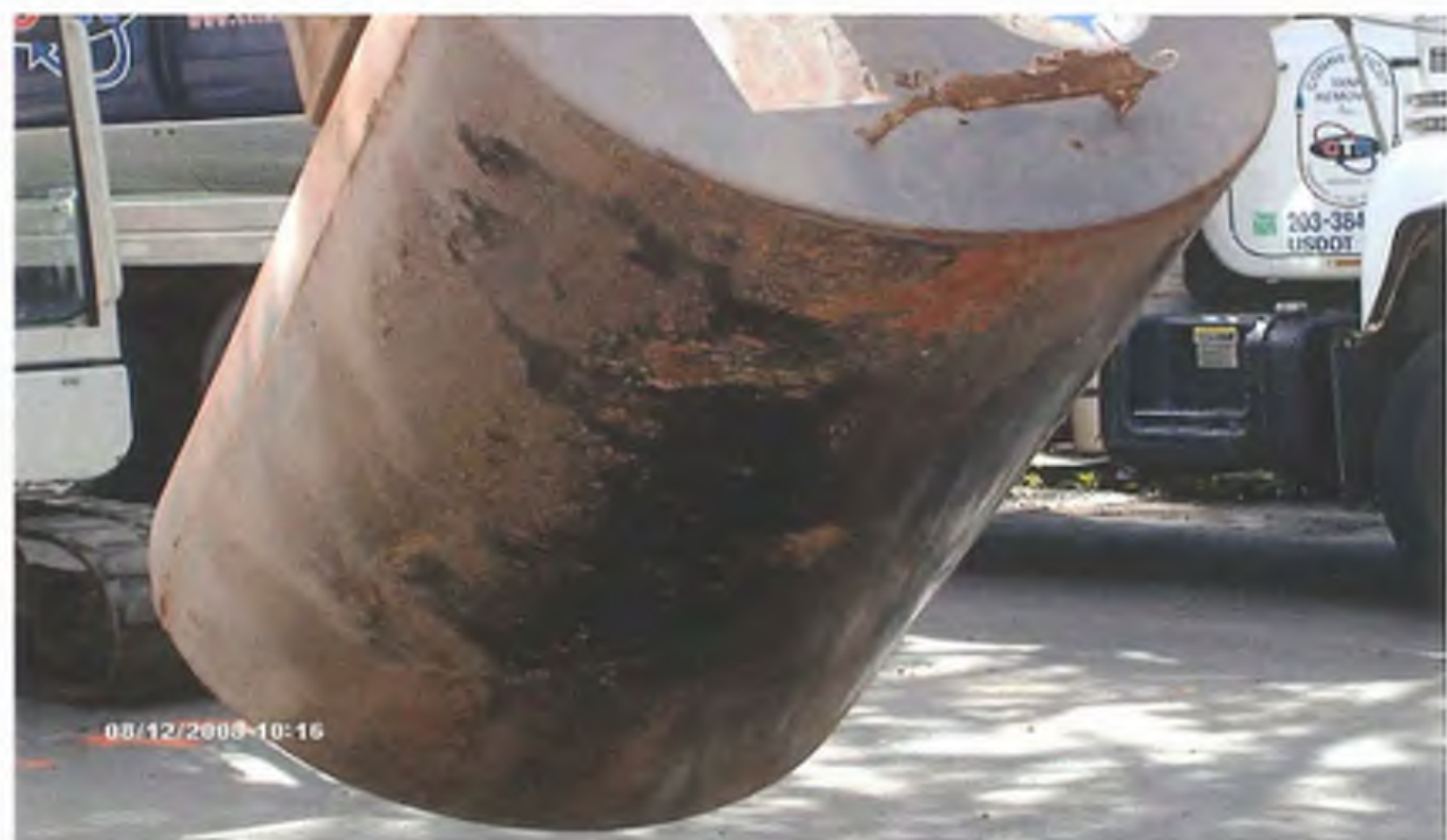
Photo 6: UST #4, minor pitting on bottom.
