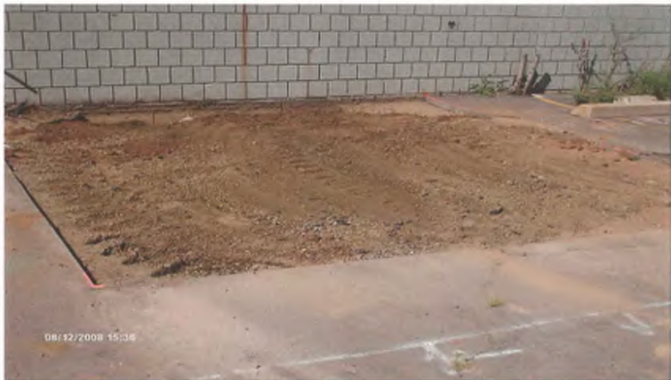
Photo 11: UST #3 excavation backfilled and compacted.
