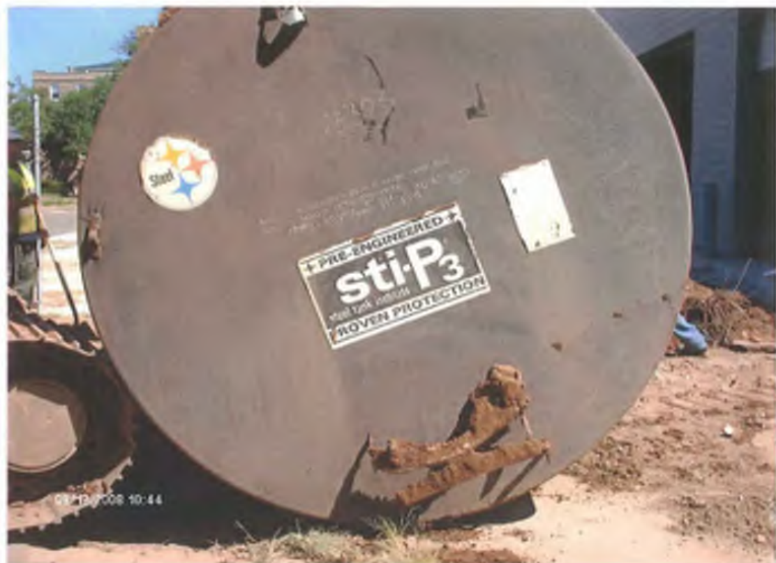
Photo 15: UST #1 removed from excavation.
