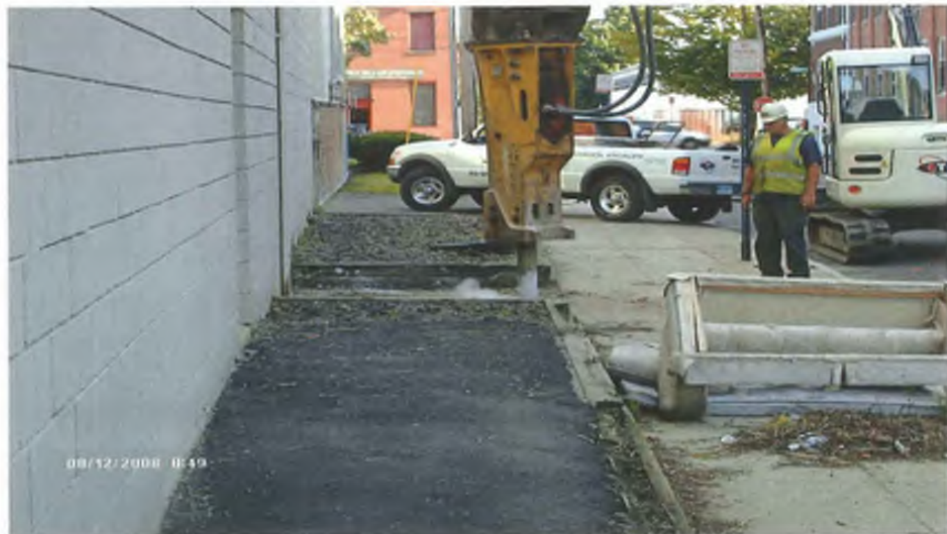
Photo 4: Removal of concrete slab over UST #4.
