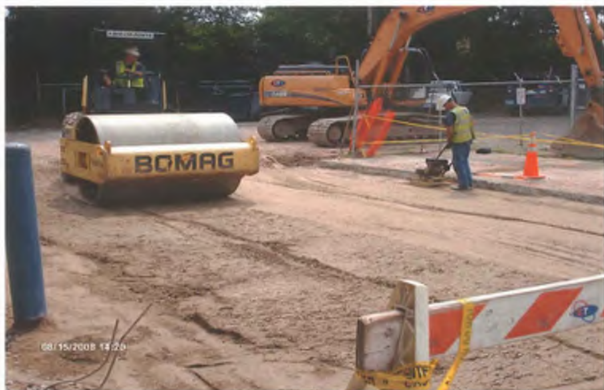
Photo 19: UST #1 and #2 excavation nearly backfilled and compacted.
