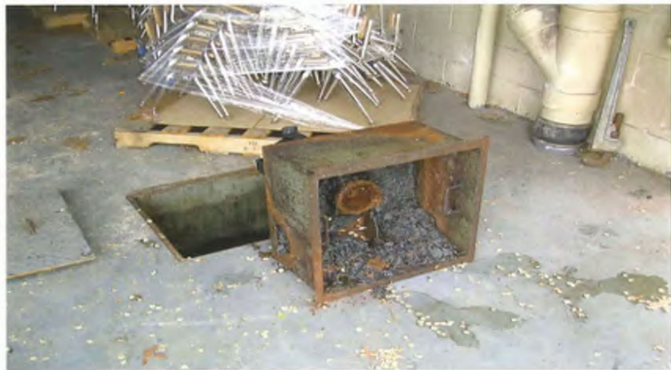
Photo 2: Interior floor drain sump and extracted sediment trap.
