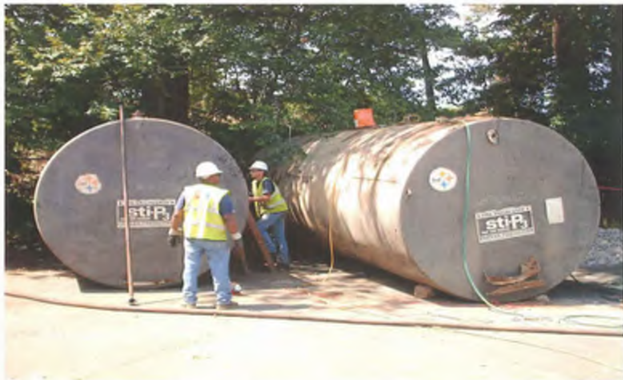
Photo 18: UST #1 and #2, preparation for decontamination and off-site disposal.
