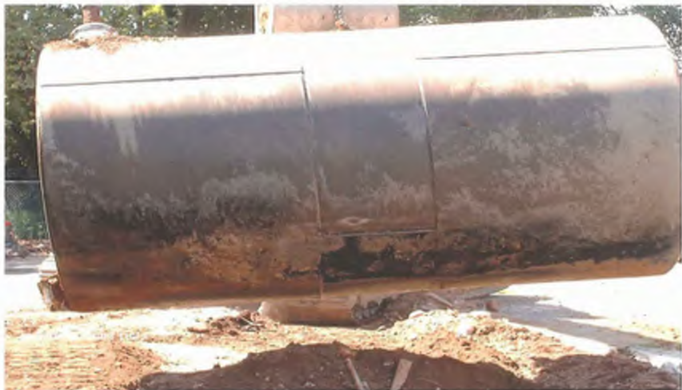
Photo 17: UST #2 removed from excavation, minor pitting observed.
