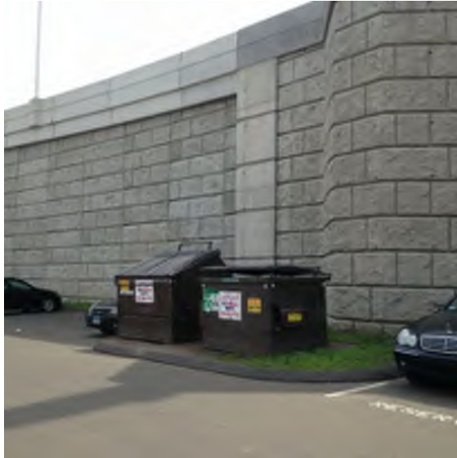
Photo 3 – I-95/I-91 Ramp and Dumpster Storage
