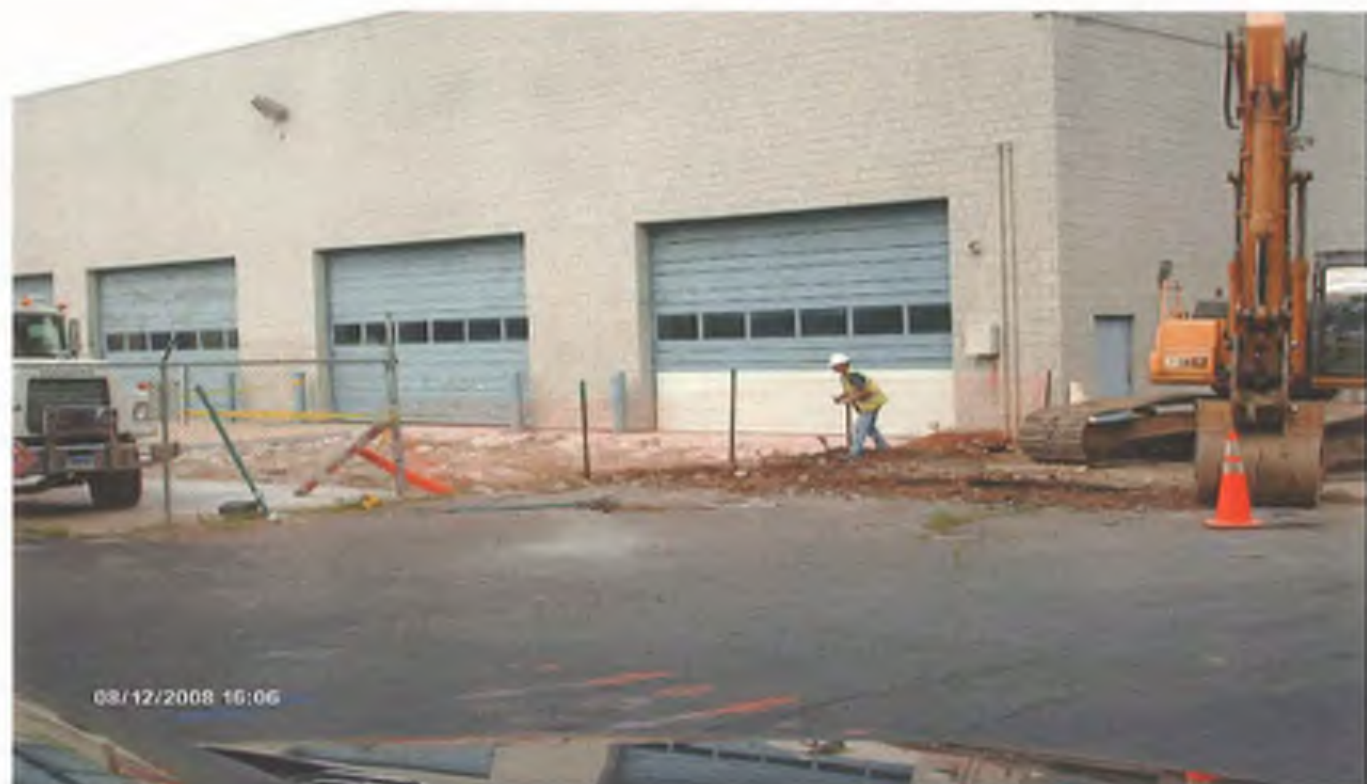
Photo 13: UST #1 and #2 concrete pad, dispenser island, and security fence removed.
