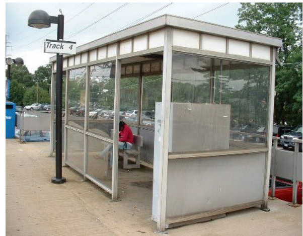
Typical Platform Shelter
