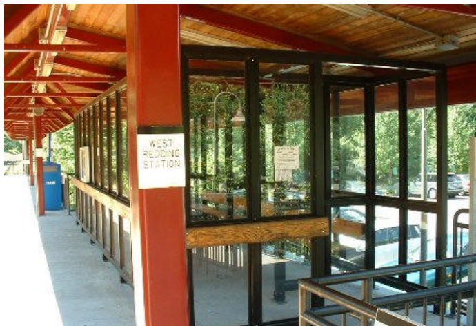
West Redding Platform Shelter
