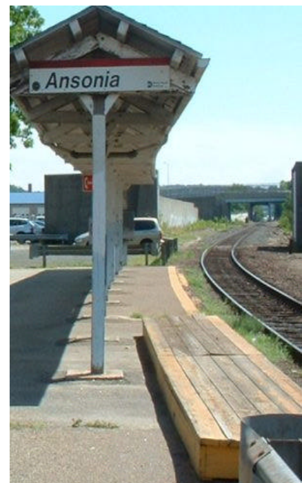
Wooden Low-Level Platform
