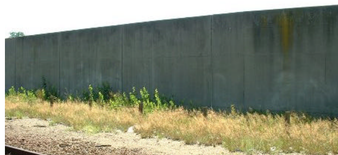
Ansonia Station Floodwall
