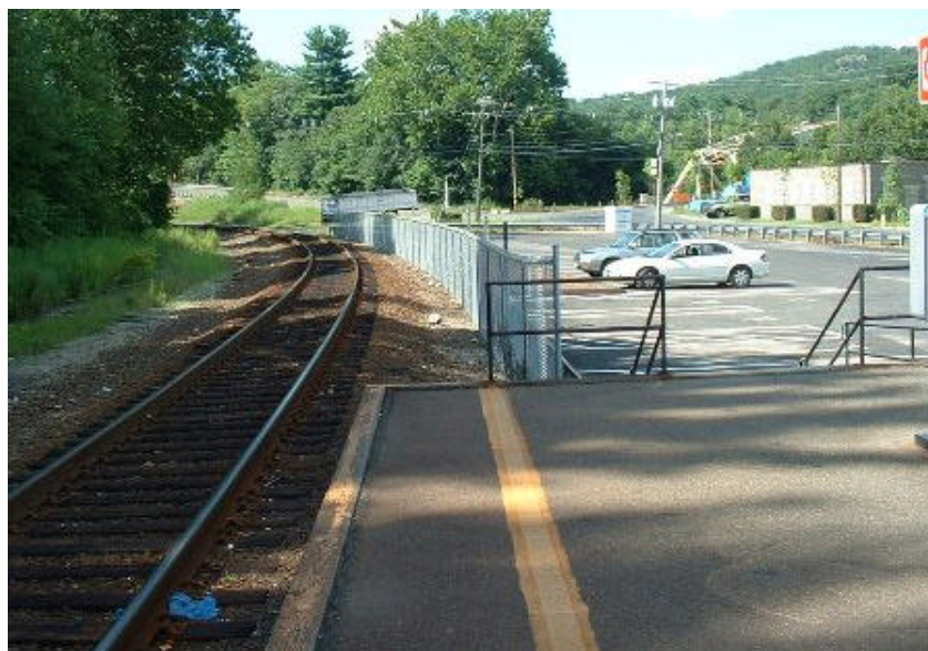
Beacon Falls Station Platform – Looking North
