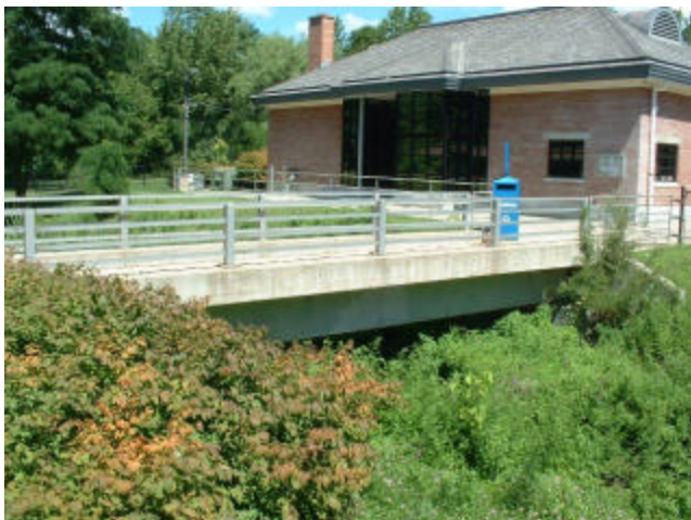
Footbridge to Platform at Bethel Station
