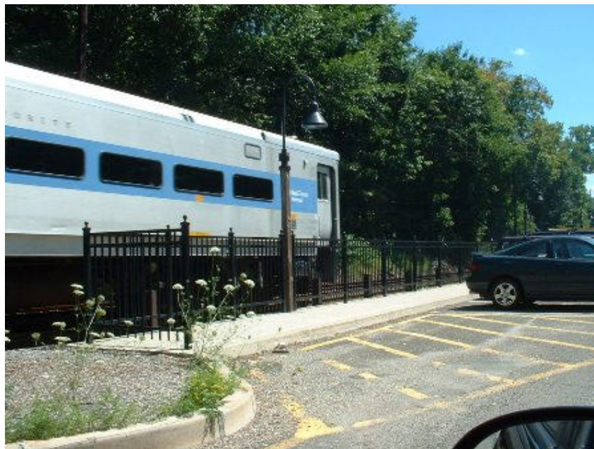
New Walk, Railing and Lights at Branchville Station
