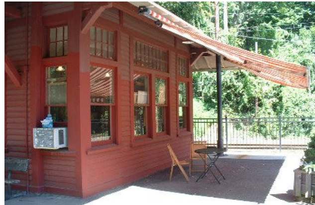
Seating Under Awning on Side of Station
