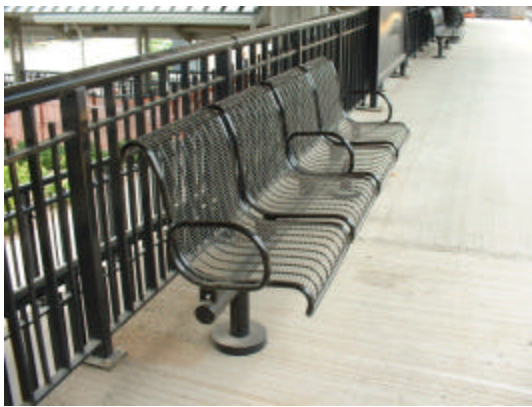
Bench (Contemporary) and Railing
