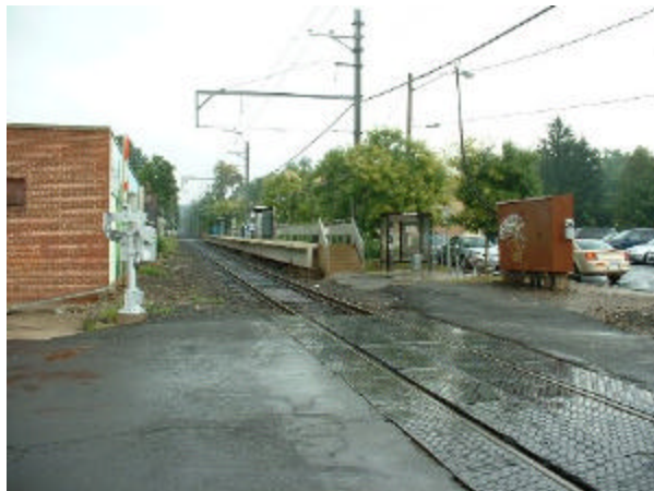
Glenbrook Station Platforms from South
