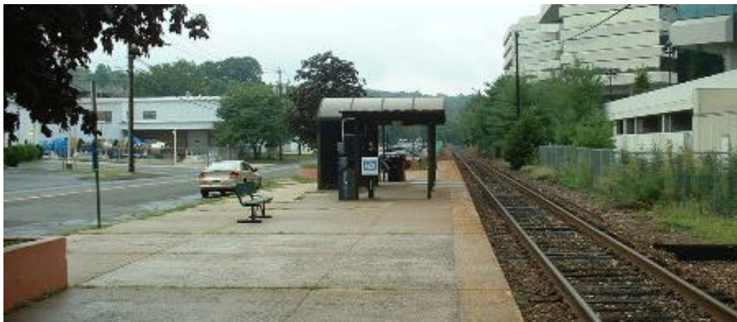
Merritt 7 Station Platform
