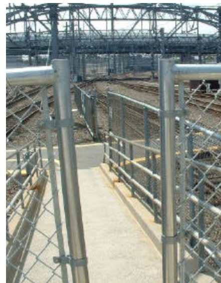
Gap in Platform Gate
