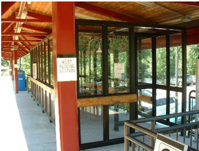
New Platform Shelter at West Redding Station
