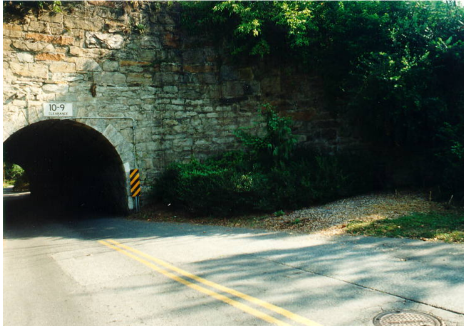
Figure 6.2.13b – Stone Masonry Arch Viaduct
