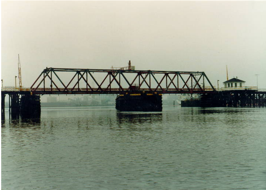
Figure 6.2.11a – Swing Span Truss Bridge.
