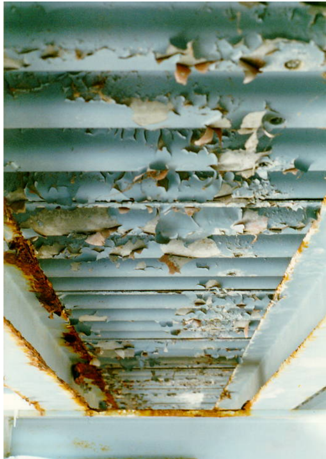
Figure 6.1.3a – Underside of Asphalt Filled Metal Deck Pans.
