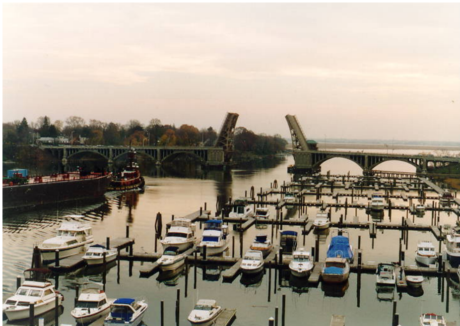
Figure 6.2.11b – Bascule Bridge in the Open Position.
