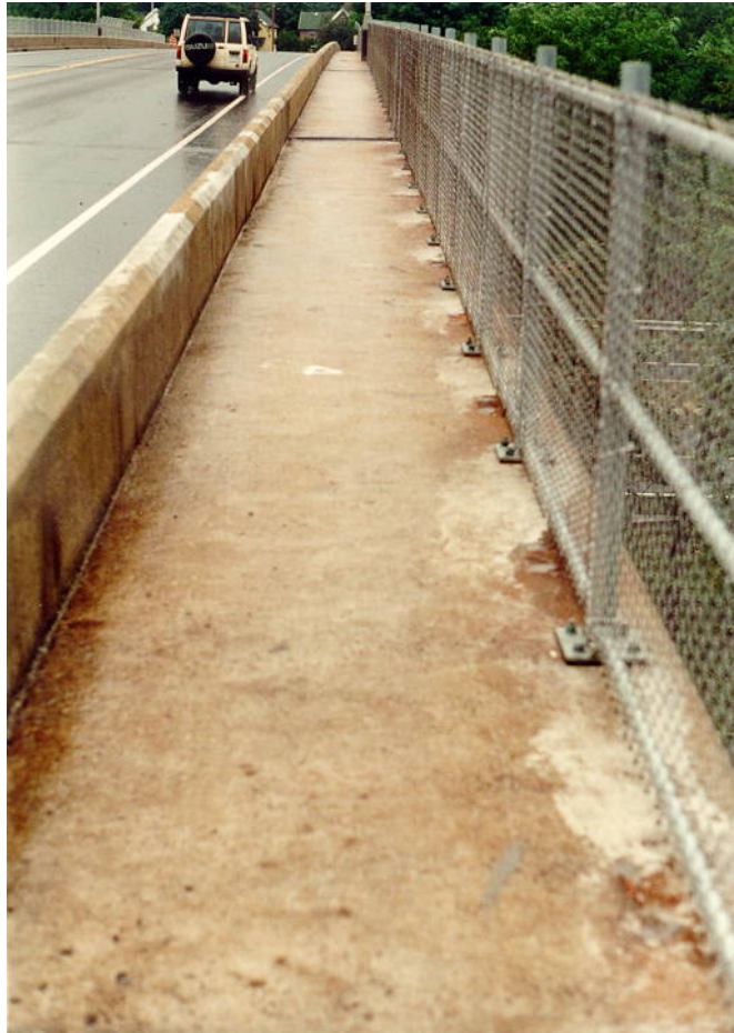
Figure 6.1.7a – Concrete Sidewalk with Pedestrian Fence and Traffic Divider.
