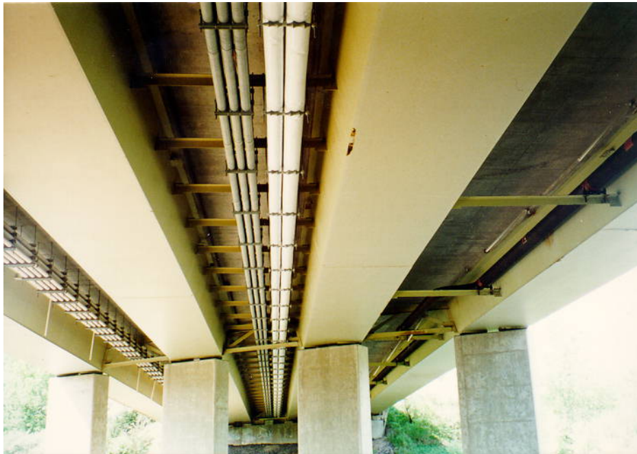
Figure 6.1.11a – Typical Under-Bridge Utility Installation
