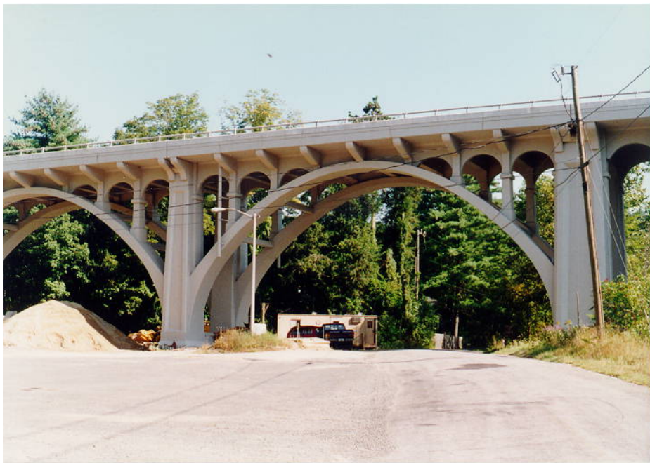
Figure 6.2.5a – Open Spandrel Concrete Arch Bridge.
