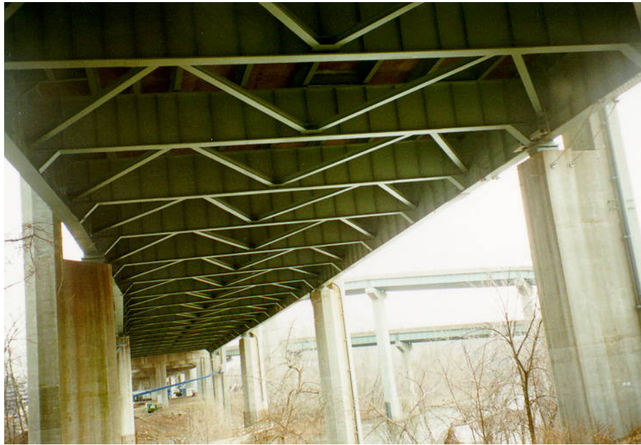
Figure 6.2.8a – Large Girder-Floorbeam-Stringer Bridge.
