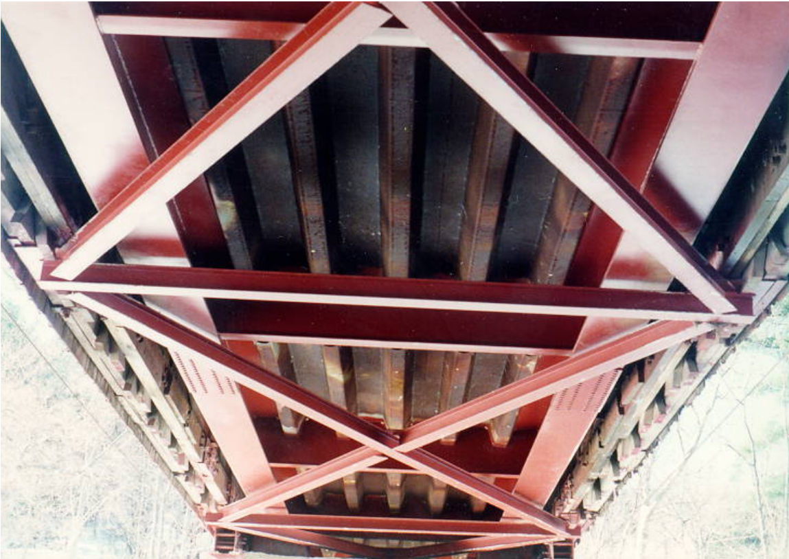
Figure 6.1.3b – Underside of Orthotropic Steel Plate Deck
