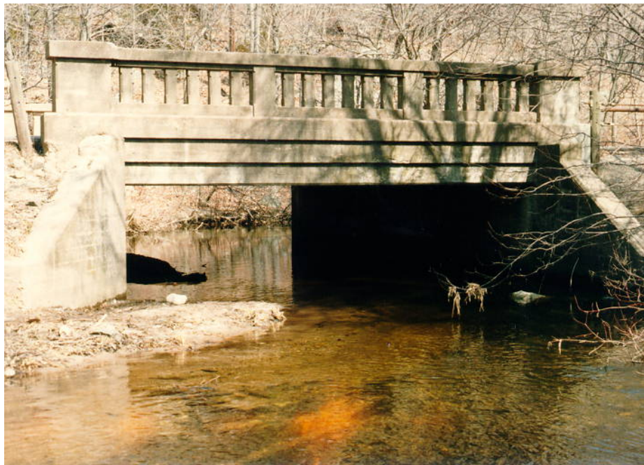
Figure 6.2.2a – Typical Concrete Slab Bridge.
