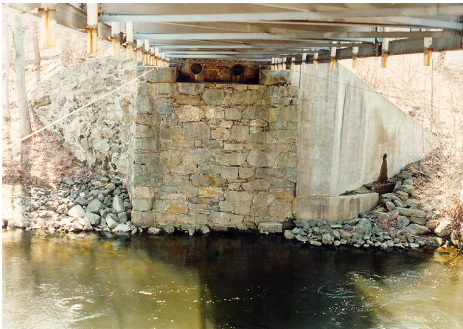
Figure 6.3.2a Tall Stone Masonry Bridge Abutment with Newer
