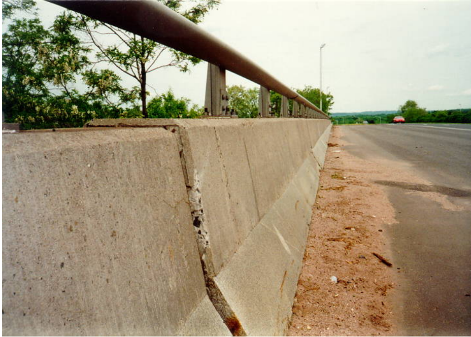
Figure 6.1.5b –Sloped Granite Curb on Concrete Parapet.
