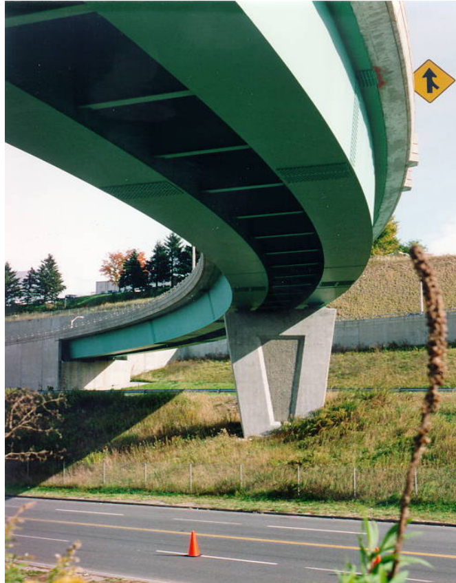
Figure 6.2.9a – Curved Steel Box Girder Bridge.
