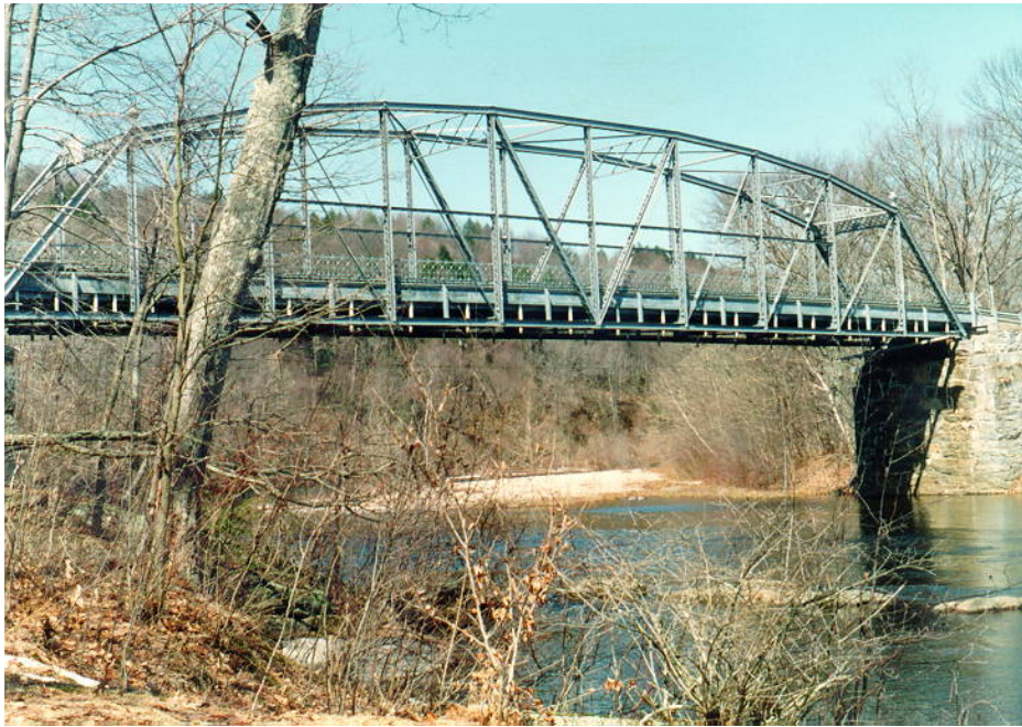
Figure 6.2.10a – Historic Steel Through Truss Bridge.
