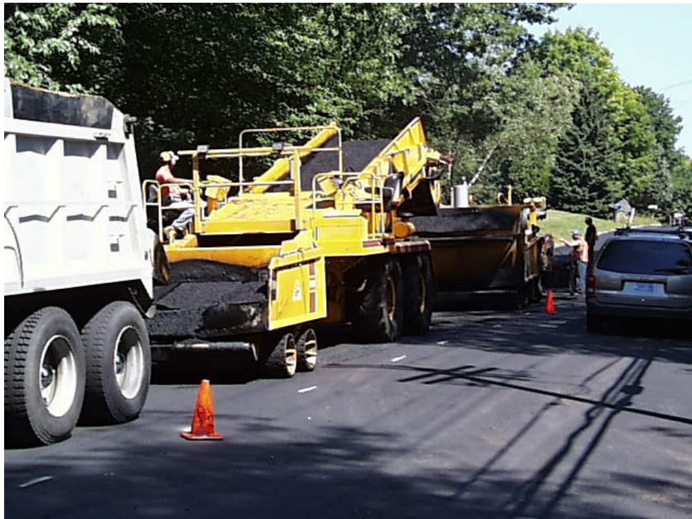
Photo 11. Blaw-Knox MC-30 Material Transfer Vehicle.
