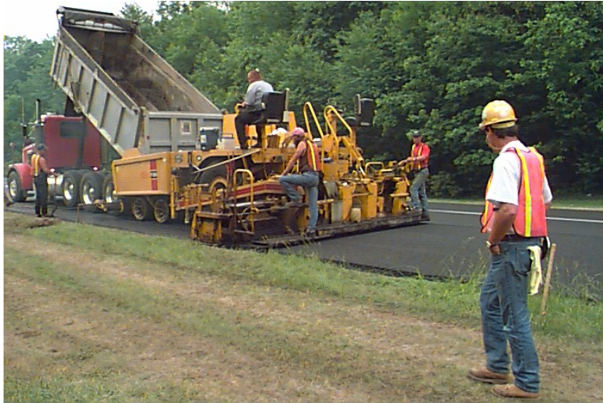
Photo A-1. Blaw-Knox PF-180H Paver Used at Sites 1 and 2.
