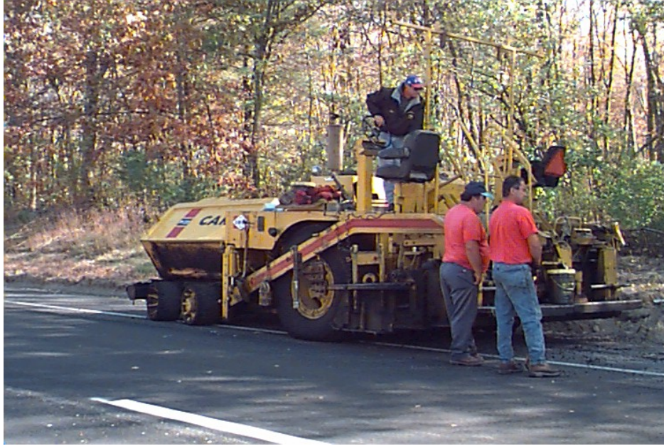
Photo A-5. Blaw-Knox PF-200 Paver Used at Site 4.
