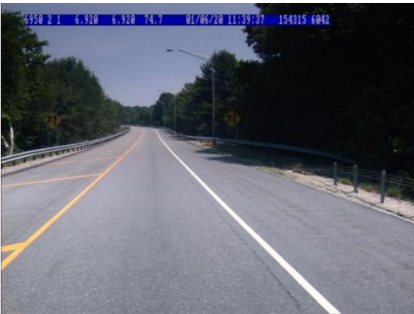
2001 - 3-years After Paving Operations
