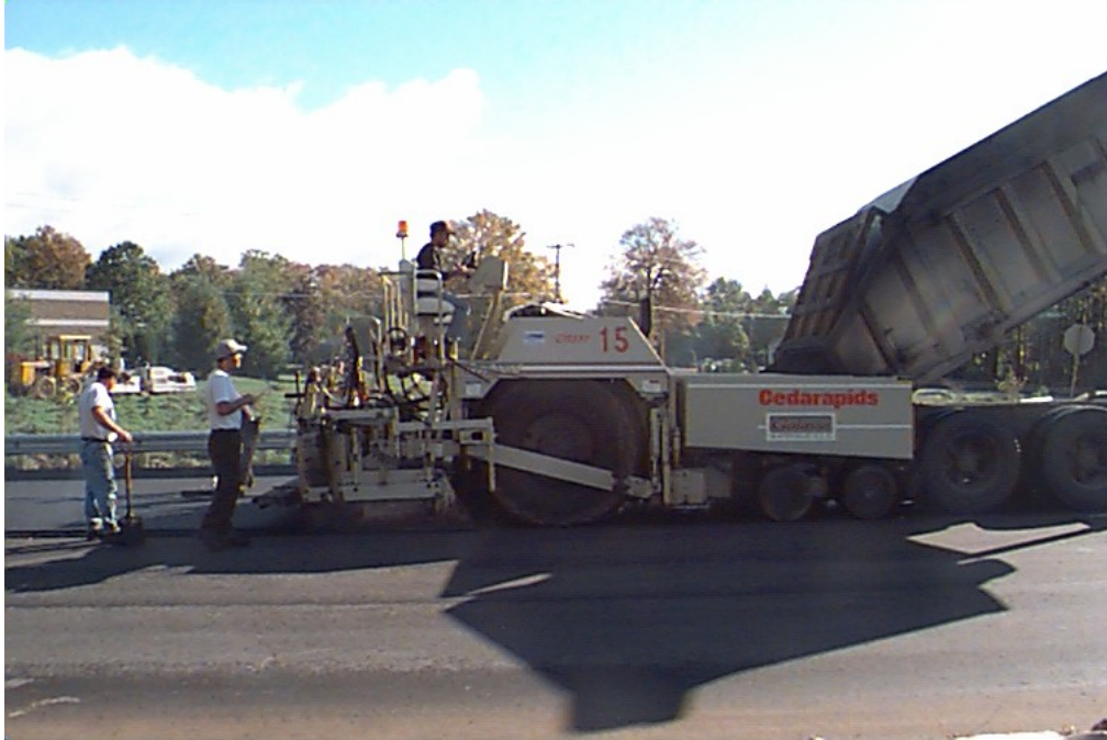
Photo A-6. Cedar Rapids CR-551 Paver Used at Site 6.
