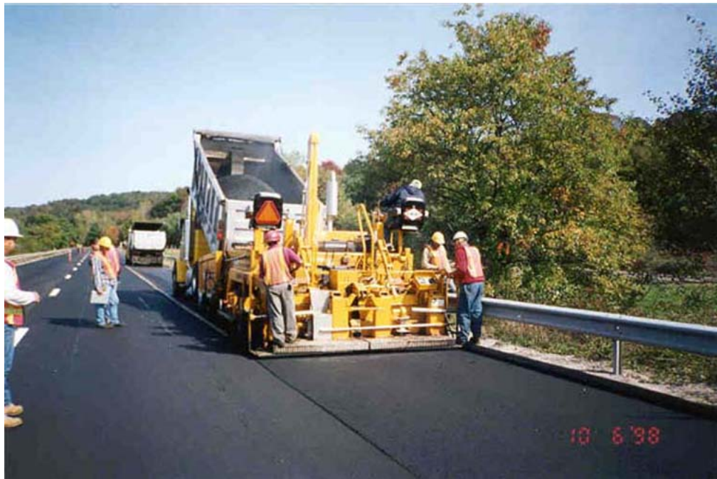
Photo A-3. Blaw-Knox PF-3200 Paver Used at Site 3.
