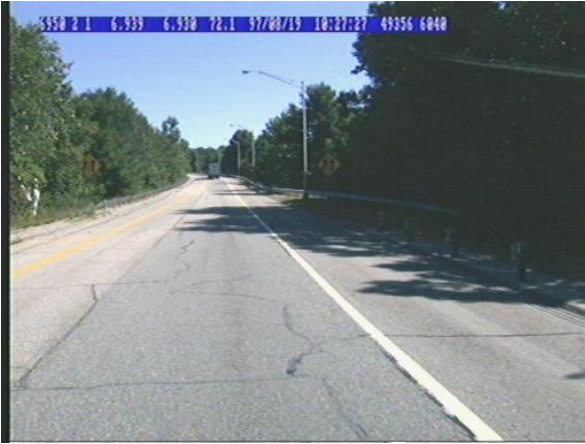
1997 - Before Paving Operations. Note: pavement was cold-in-place recycled for base.
