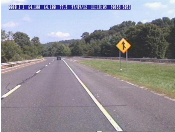
1997 - Prior to Milling and Paving
