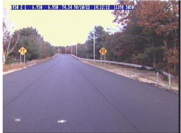
1998 - Immediately after Paving Operations. Surface paved over cold-in-place recycled base.
