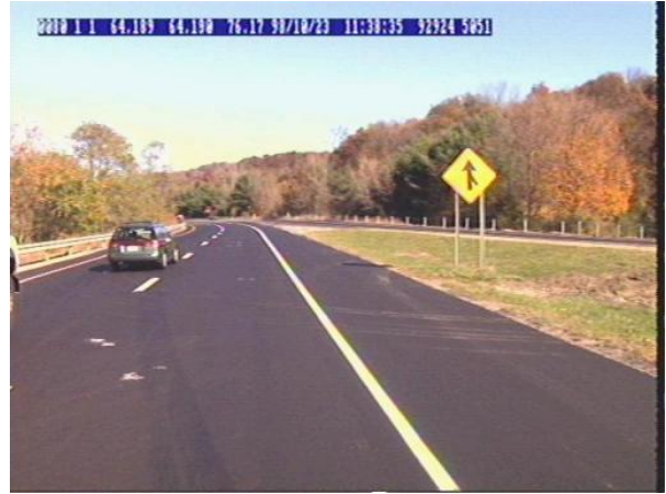
1998 - After Milling and Paving
