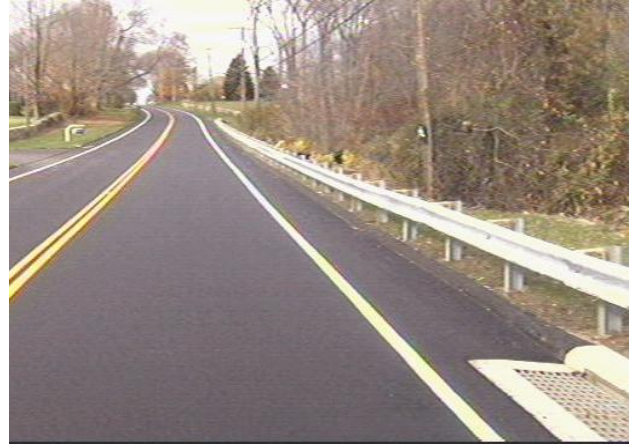
1998 - After Paving Operations
