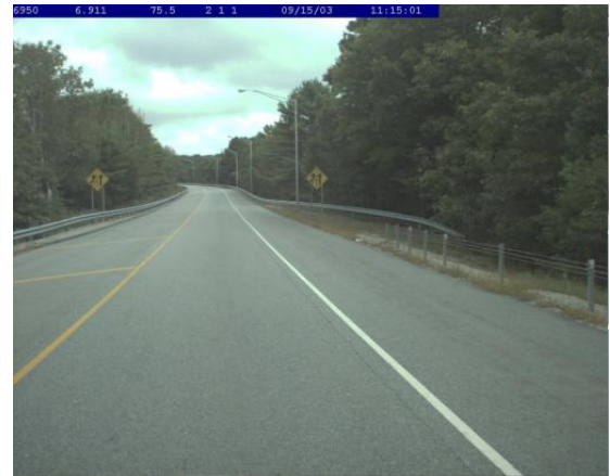
2003 - 5-years After Paving Operations
