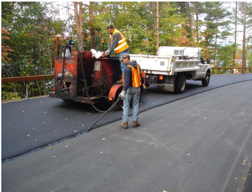
Figure 13 Rubberized Joint Sealant Application
