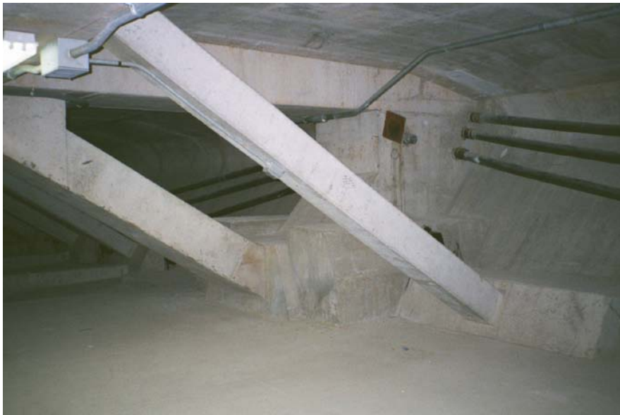
Figure 4. View of Bridge Interior
