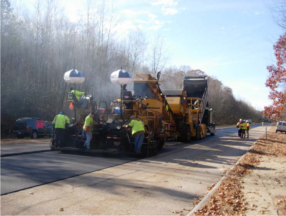
FIGURE 1 Paving Train at Project 28-197.
