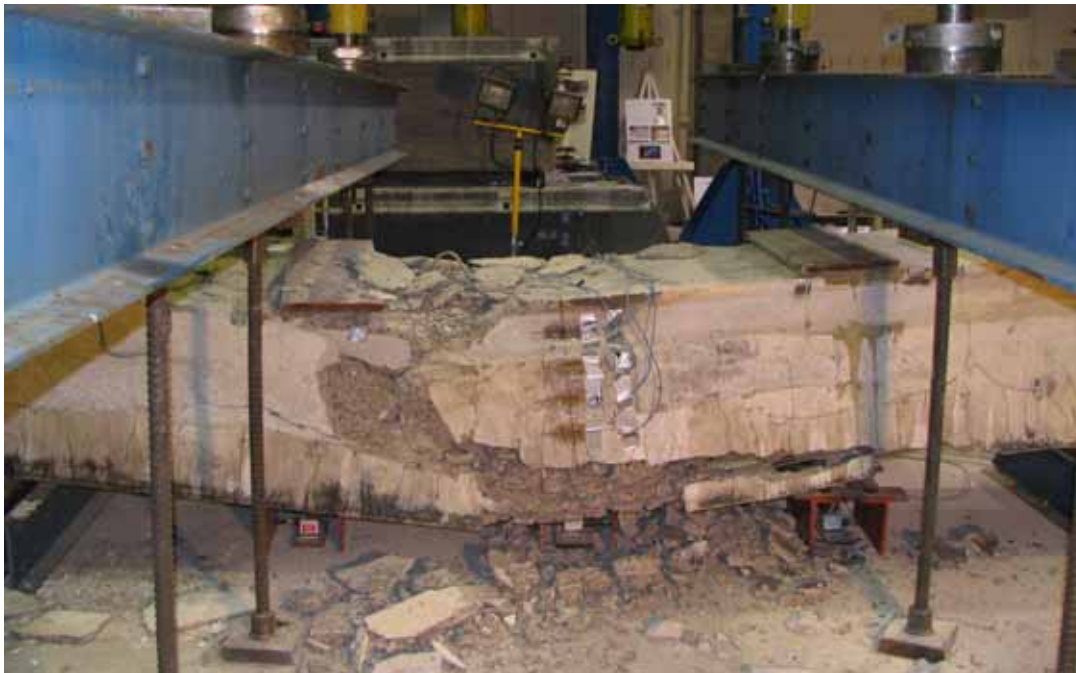
Figure 24. Photo. Failed Beam 14.
