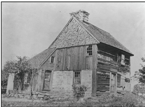
The ca.1690 Norton House, Guilford. This house was a small one-room end-chimney type with a lean-to off the back.
