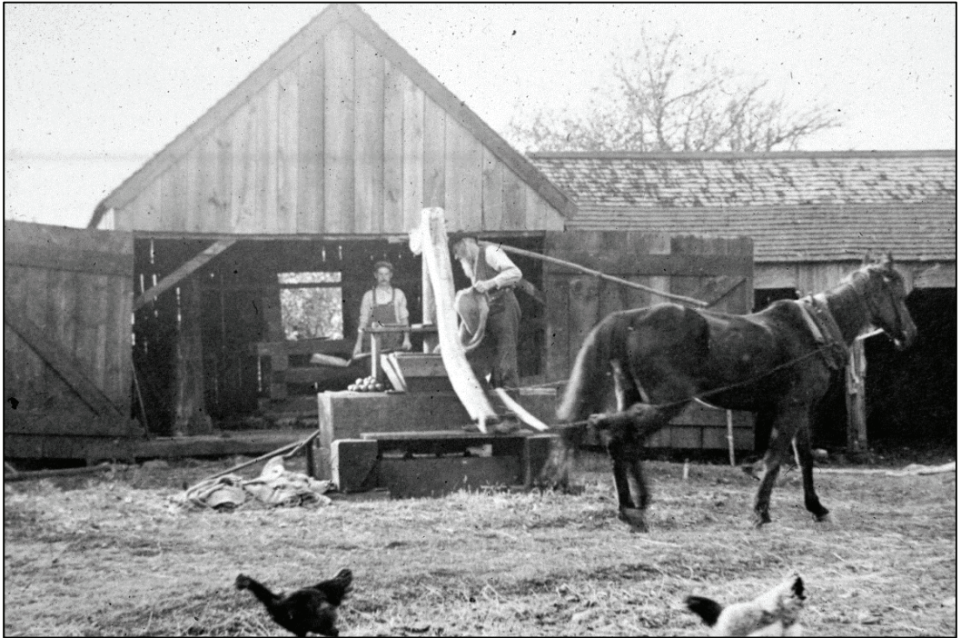
An old photograph of Connecticut farmers working a horse-powered cider mill. The mechanism ground up the apples which were then pressed to extract the juice. The Goodsells' cider mill may have looked a lot like this one.
