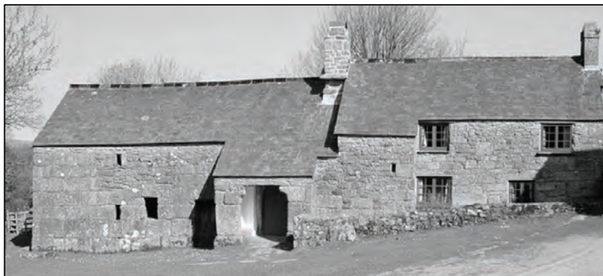
The Sanders longhouse, an early 16th-century stone cross-passage house in Devon, England. Photograph courtesy of Derek Harper.
