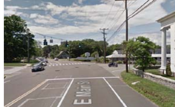
This intersection has very wide turning radii, which encourages fast right turns and creates unsafe walking environment in Clinton
