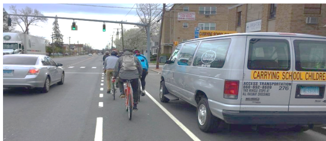
E. Hartford, Route 44 Road Diet 4 lanes reduced to 2 thru lane + 2 bike lane
