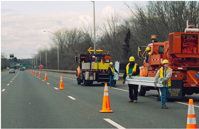
CTDOT making SOGR improvements
