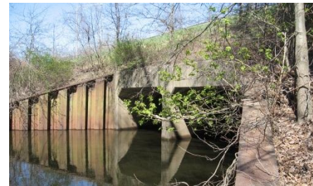
Keeney Cove Culvert
