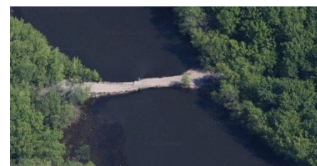
Point Road bridge over Keeney Cove (Source: Google)
