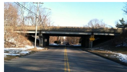
Route 3 bridge over Naubuc Avenue
