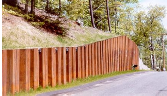
Example sheet pile retaining wall that is similar in appearance to the retaining wall recommended for use along the shared use path in Glastonbury. If desired, alternative façade treatments can be incorporated into the wall design and construction for additional cost.
