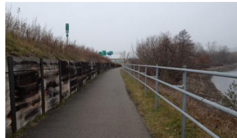
Example of a shared use path cut into the side of a roadway embankment along I-890 in Schenectady, NY.
